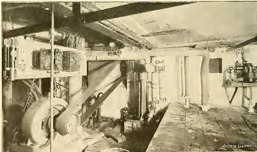
FIG. 3. MECHANICAL AND ELECTRICAL EQUIPMENT OF THE UNION HOTEL.—MOTORS IN THE ENGINE ROOM.
