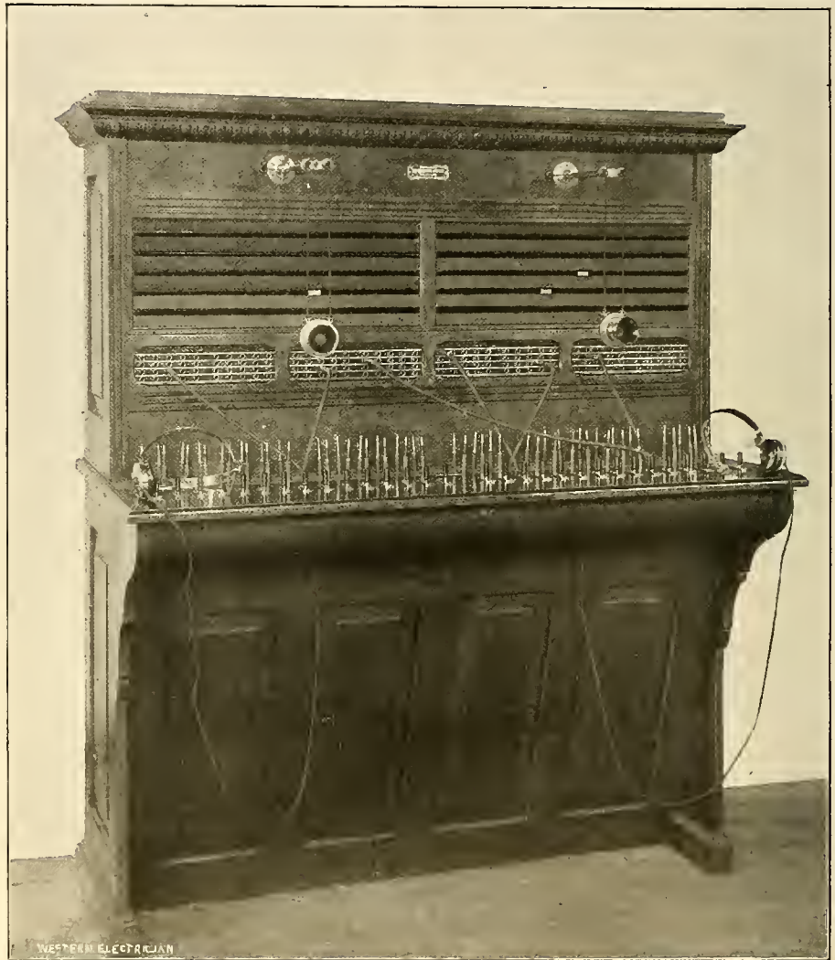
FIG. 1. CHICAGO BOARD OF TRADE TELEPHONE SYSTEM.
