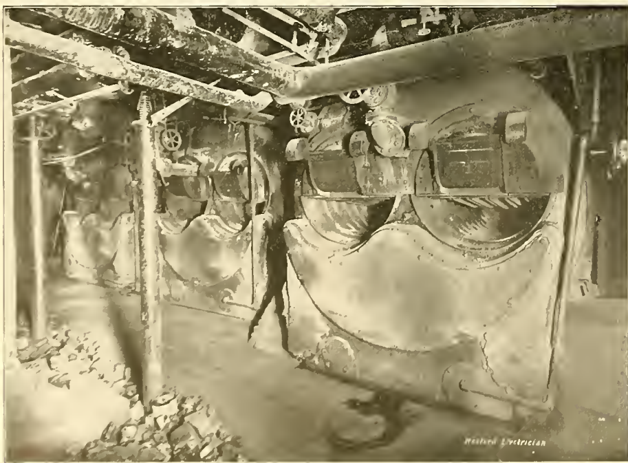
FIG. 2. GREAT NORTHERN ELECTRICAL PLANT.—SCOTCH BOILERS.
