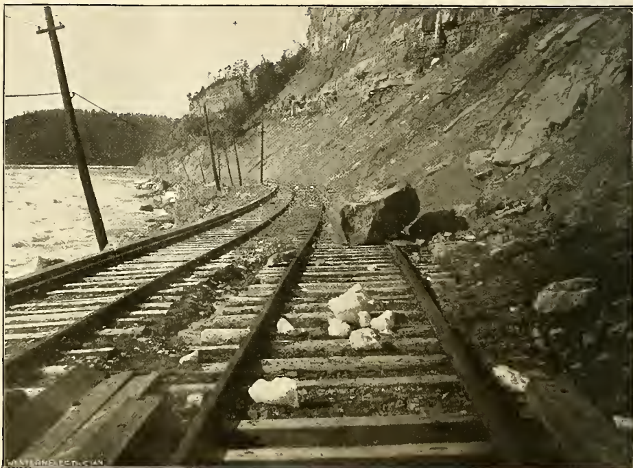
GORGE ROAD AT NIAGARA FALLS.—CONDITION OF TRACKS IN SPRING.
