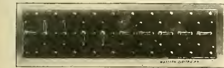
LEVER SWITCHBOARD FOR TOLL LINES.
