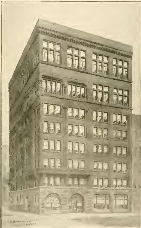
Building with the Addition Now Making.
