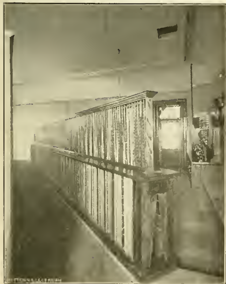
FIG. 3. CENTRAL OFFICE SYSTEM OF THE NEWARK TELEPHONE COMPANY.—DISTRIBUTING BOARD, TEST SIDE.
