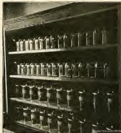
FIG. 4. CENTRAL ENERGY SYSTEM AT HENDERSON, KY.—BATTERY EQUIPMENT AT EXCHANGE.
