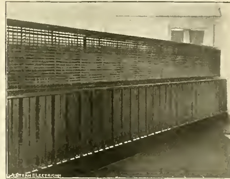
FIG. 4. CENTRAL OFFICE SYSTEM OF THE NEWARK TELEPHONE COMPANY.—DISTRIBUTING BOARD, ARRESTER SIDE.
