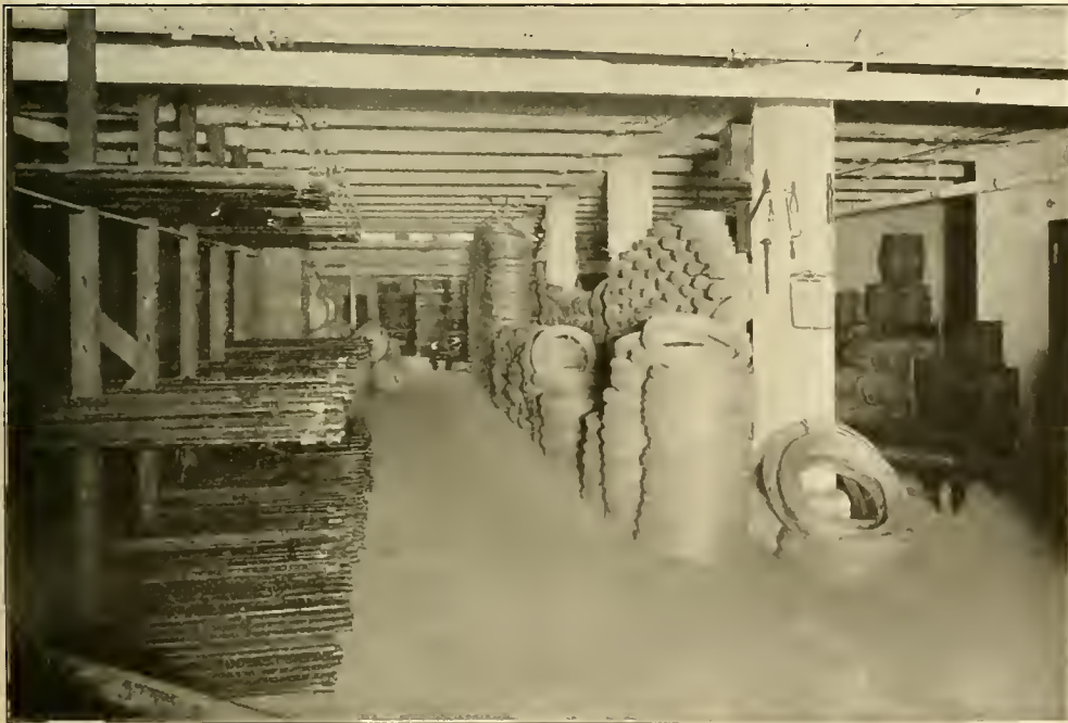
ELECTRIC APPLIANCE COMPANY IN ITS NEW HOME.—VIEW IN BASEMENT.
