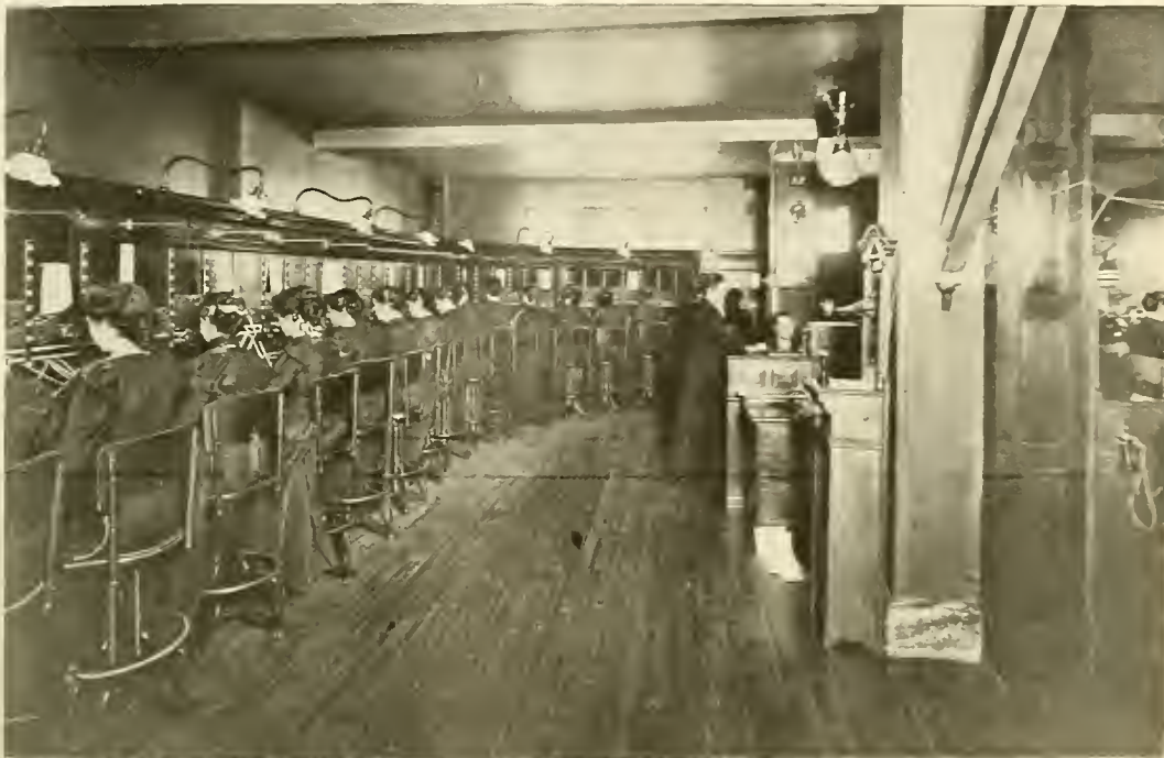
Fig. 1. "A" Switchboard at "Harrison"
