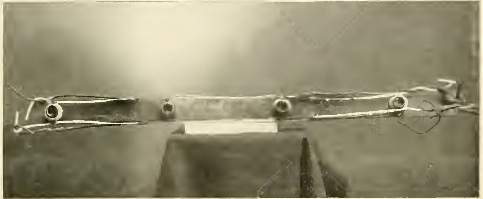
FIG. 1. POOR ELECTRICAL CONSTRUCTION.
