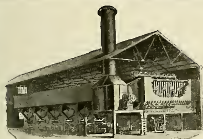
Battery of Boilers Equipped with Westinghouse Mechanical Draft.
