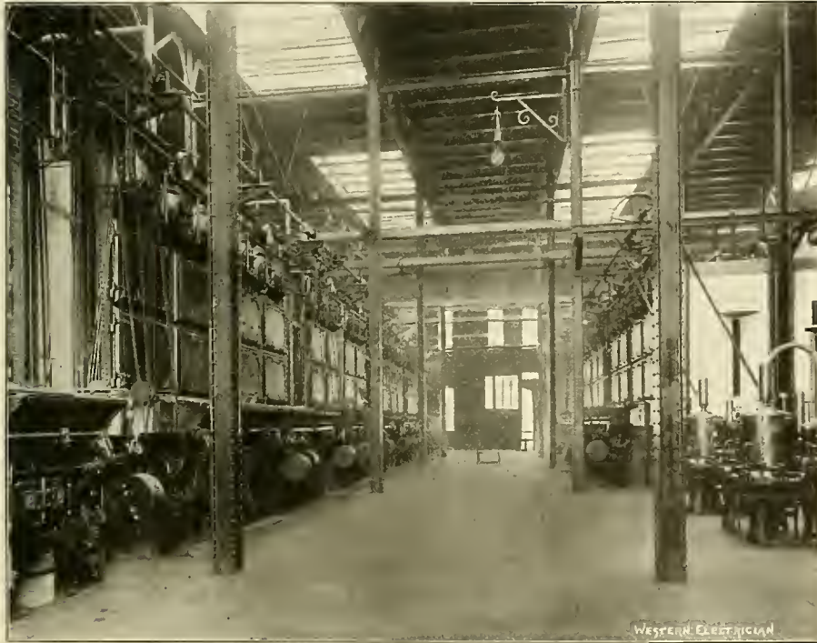
FIG. 5. UNION LOOP POWER HOUSE.—BOILER ROOM.
