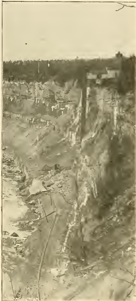
FALLING ROCK ON GORGE ROAD AT NIAGARA FALLS.
