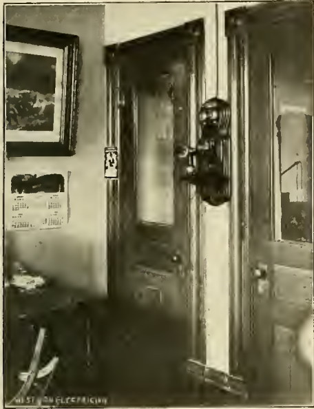
FIG. 3 CHICAGO BOARD OF TRADE TELEPHONE SYSTEM.
