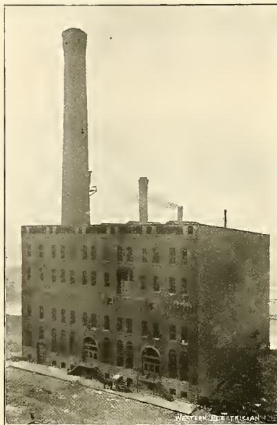
FIG. 2. UNION LOOP POWER HOUSE.
