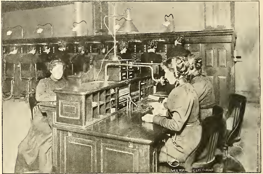
FIG. 3. TWO NEW TELEPHONE EXCHANGES IN CHICAGO.—CHIEF OPERATOR'S DESK AND "B" BOARD AT "CENTRAL."
