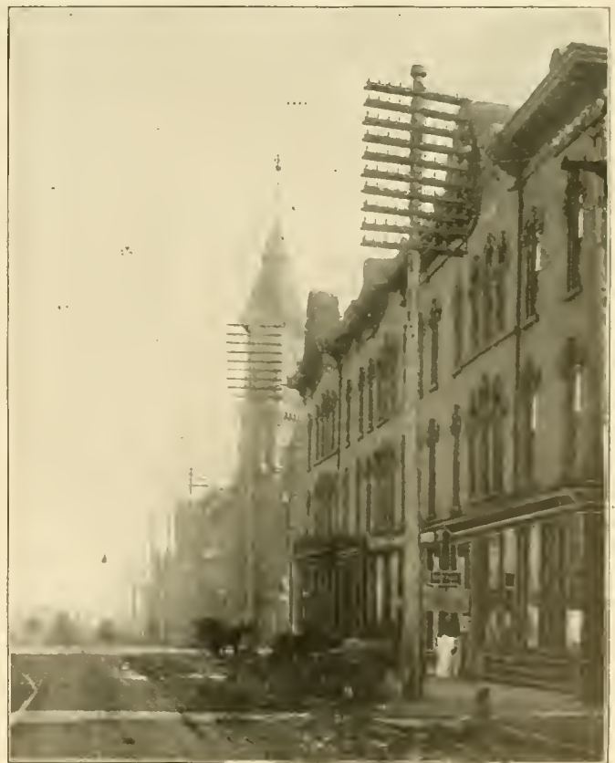
FIG. 4. LARGEST INDEPENDENT EXCHANGE IN IOWA.—LINE EQUIPMENT WITH POLE-TOP TERMINALS.
