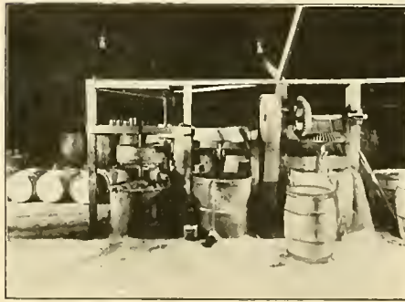
Fig. 3. Tank and Stock Floor.
