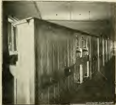
FIG. 2. CENTRAL OFFICE SYSTEM OF THE NEWARK TELEPHONE COMPANY.—BACK OF MAIN SWITCHBOARD.
