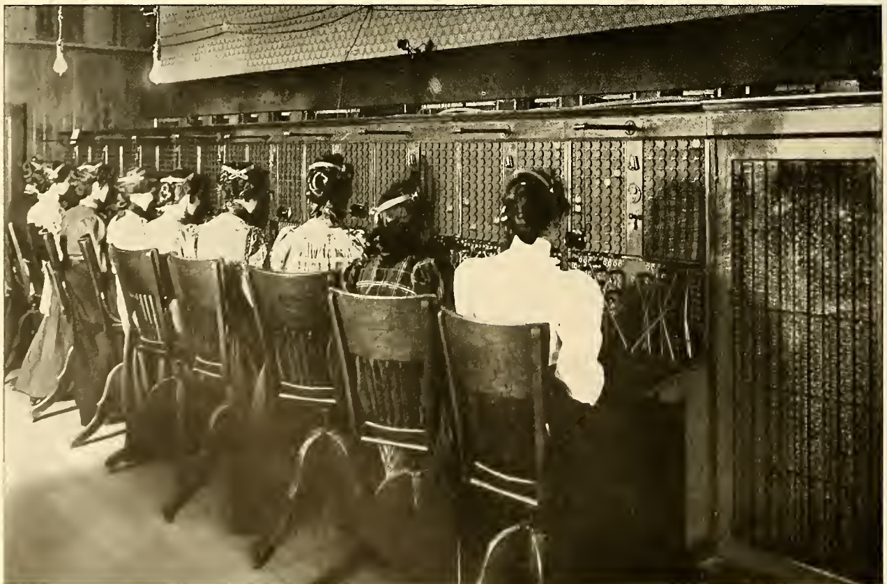
1,000-Drop Sterling Board Showing the Distributing Board at the Left.
