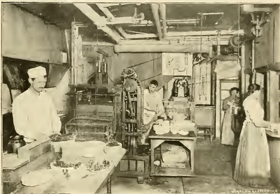
FIG. 4 MECHANICAL AND ELECTRICAL EQUIPMENT OF THE UNION HOTEL.—MOTOR-DRIVEN DISH-WASHING MACHINE AND DUMB-WAITERS.
