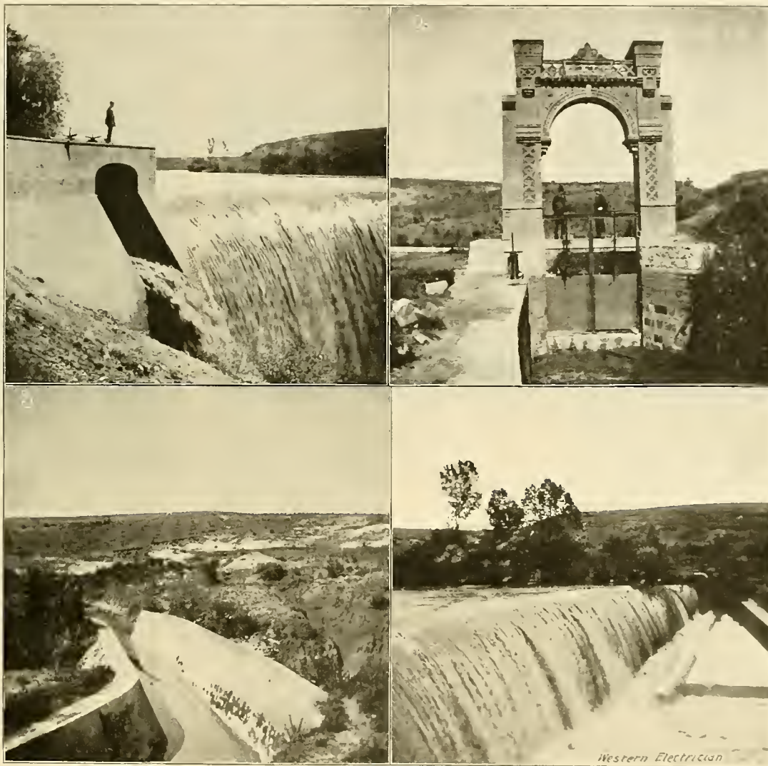
Fig. 1. Dam to Divert Water from Atoyac River into the Canal. Fig. 3. Section of Canal.
