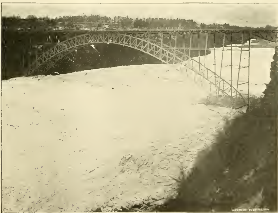
FIG. 2. STEEL ARCH BRIDGE AT NIAGARA THREATENED BY ICE BRIDGE.
