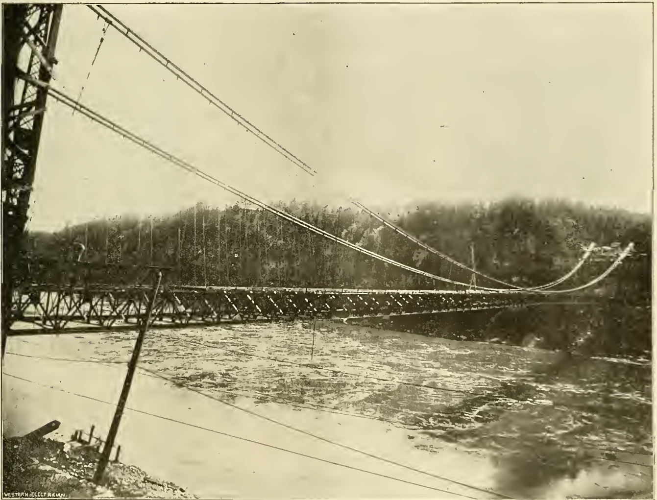
SUSPENSION BRIDGE FOR TROLLEY LINES AT NIAGARA.
