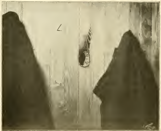
INCANDESCENT LAMP BURNS HOLE IN PARTITION.
