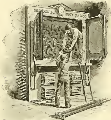
Handing down the second connecting bend. (Between this operation and that shown in the next cut, the same operations are performed at the rear of the boiler.)
