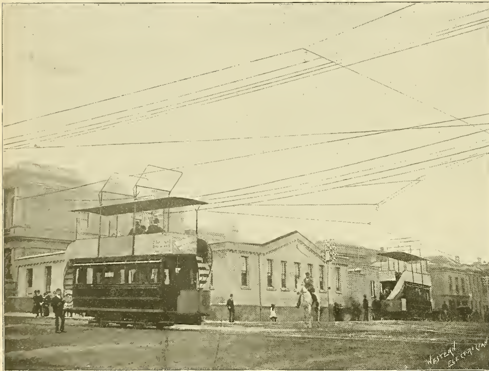
AN AUSTRALIAN ELECTRIC RAILWAY.
