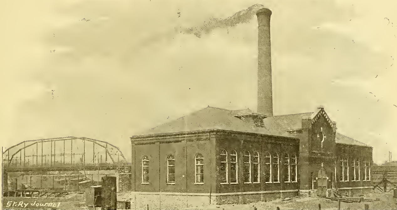
CENTRAL POWER STATION AT NEWPORT, KY.
