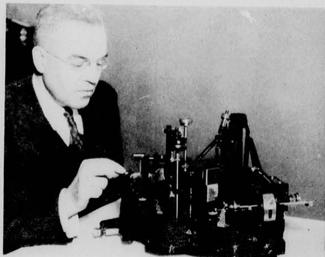
Above. Geophysicists of the Department of Geology developed this seismograph which is responsive to earth displacements of less than a millionth of an inch or to forces corresponding to a small fraction of the weight of a pinhead
