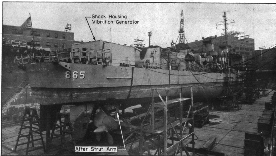
Figure 4a - Stern View Showing Temporary Shack
