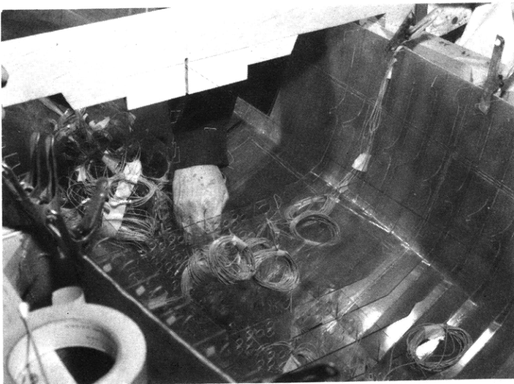
Figure E.6 - The 0-1 Level and Main Deck "Cross-Frame" Struc- ture is Removed for Installatio of Strain Gages on the Lower or Second Deck
