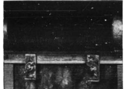
Use of gang saw to slot etched-wiring terminals of memory plane, in preparation for insertion of interconnecting shims
