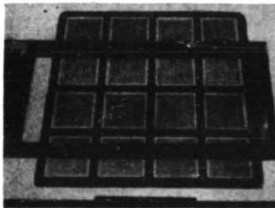
Array of 16 memory planes, interconnected by copper shims to give 256x256 memory plane. Complete random-access memory under development will have 38 of these large planes
