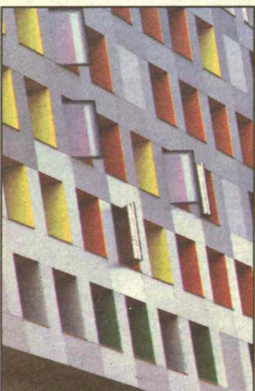
A closeup of the multicolored exterior windows at Simmons.
