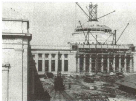
Construction of the original Cambridge campus, 1910s.
