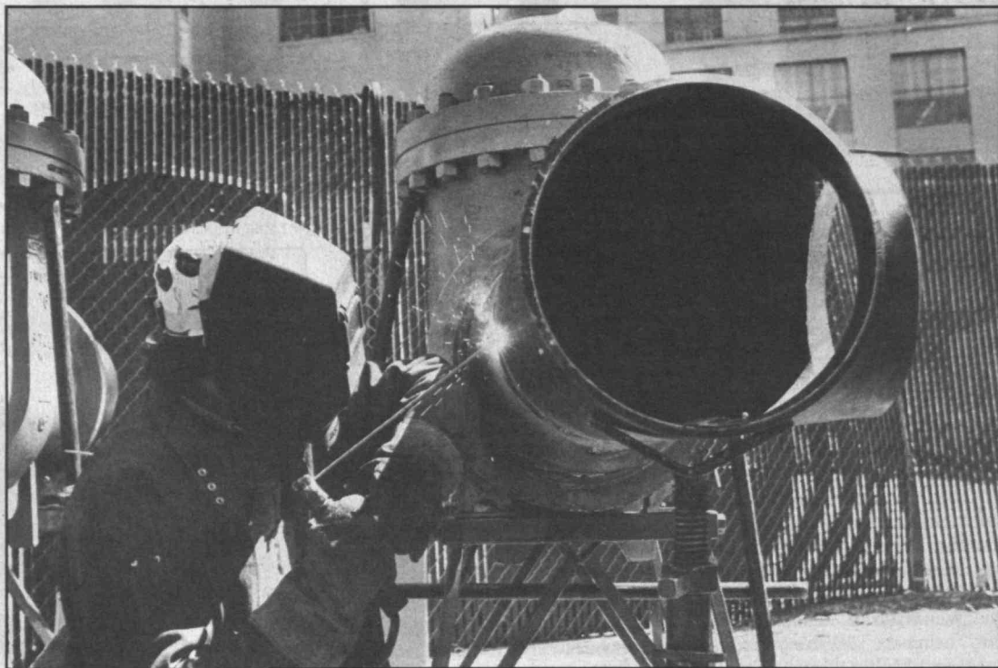
Marty Joseph of Pipefitters Local 537 does some welding outside Building 26.
