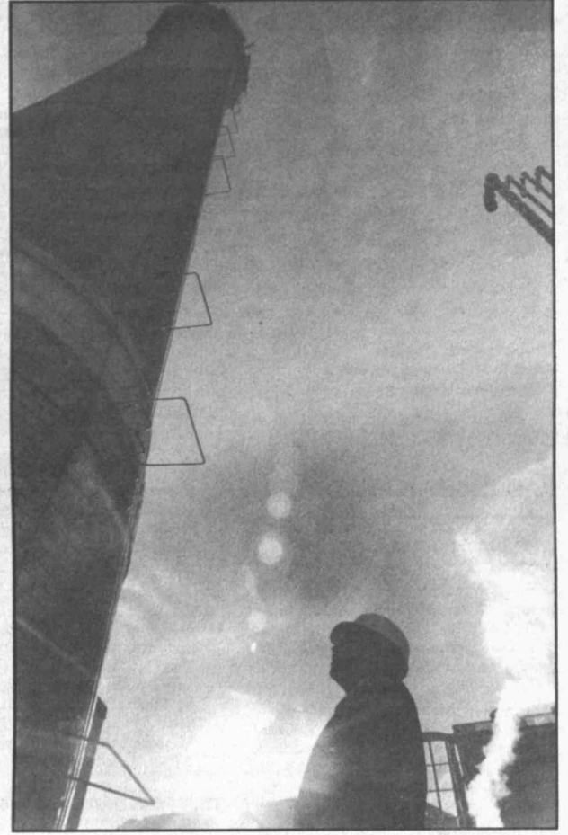
Physical Plant engineering assistant Vaughn Crayton gazes up at the plant's smokestack.
