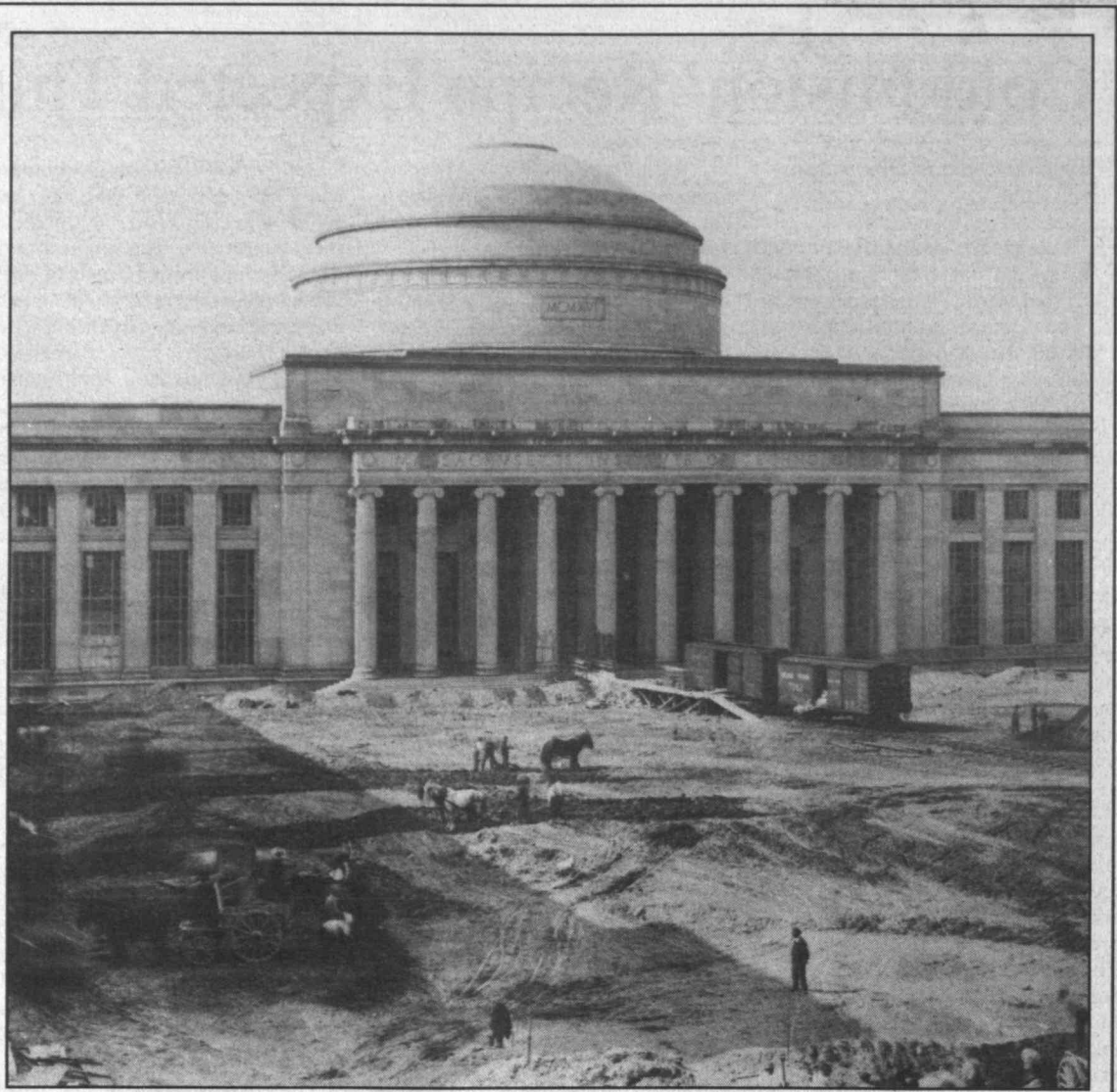
STATE OF THE ART 1915—A railroad siding was built into what is now Killian Court, and horses were used to move the Indiana limestone and other heavy materials needed for building the main MIT complex. MIT Museum Photo
