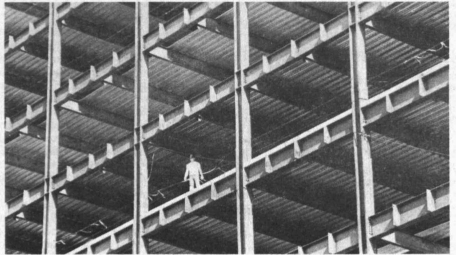
Workman is dwarfed in this construction picture in Kendall Square.
