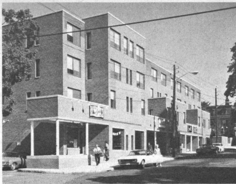
PEMBROKE DORMITORIES at Brown University were designed by Lyndon Associates, Inc., of Cambridge, an architectural firm founded by MIT Professor Donlyn Lyndon. The firm recently received an Honor Award from the Boston Society of Architects for its work on the dormitories.
