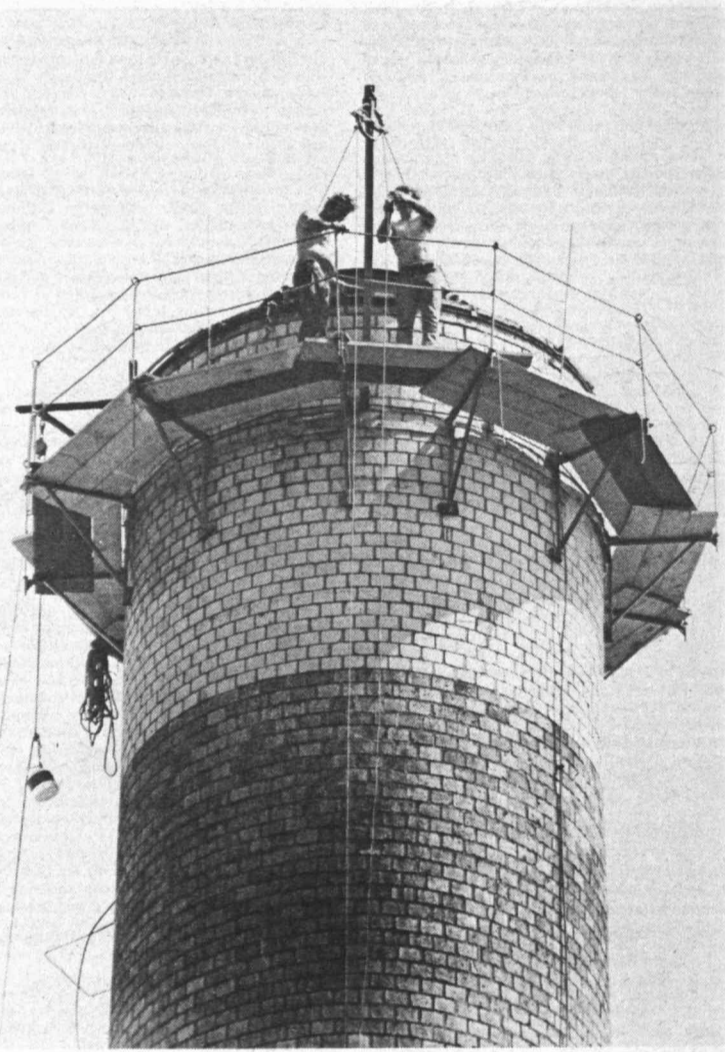
HIGH AND DRY are these employees of Boston Chimney and Tower Co., Salem, working in Tuesday's heat atop the 180-foot chimney at the MIT Central Utilities Plant, Building 42. They won't be dry for long, however, because the insulated jug being hoisted aloft on the rope to the left of the chimney is full of Kool Aid. The workmen are replacing the metal cone on the top of the chimney and repairing the brickwork on the face of the structure. The cone, part of the stack's anti-pollution equipment, was damaged in a recent windstorm. —Photo by Calvin Campbell
