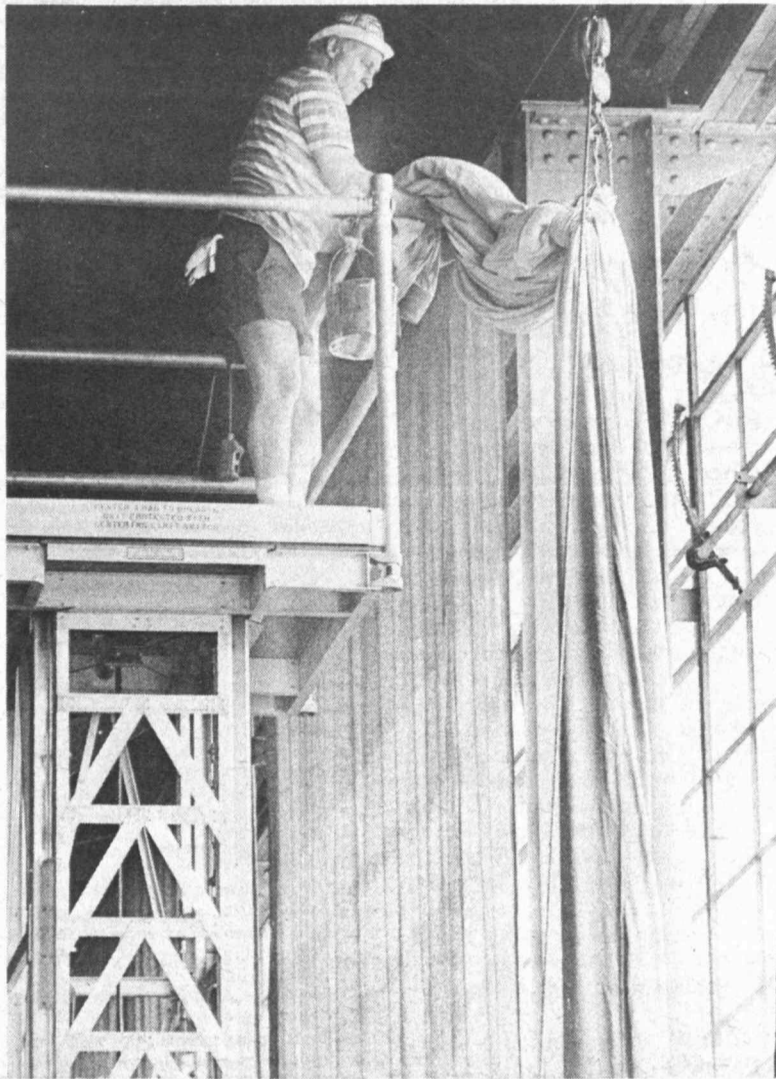
HANGING CURTAINS in Rockwell Cage for commencement is Tony Gedraitis, shade man in Physical Plant. He is standing on an electrical staging and taking the curtain from the block and tackle used to hoist it. Thirty-six curtains, each 22 feet long, are hung at the four walls of Rockwell Cage each year for commencement. Hanging the curtains takes five work days for three men; taking them down, another five work days for four men.
