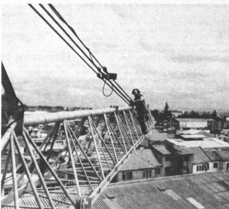
George S. Lechter, a junior in mechanical engineering, checks the boom of the heavy construction crane which he redesigned last summer while working for a Bogota, Colombia equipment manufacturer.
