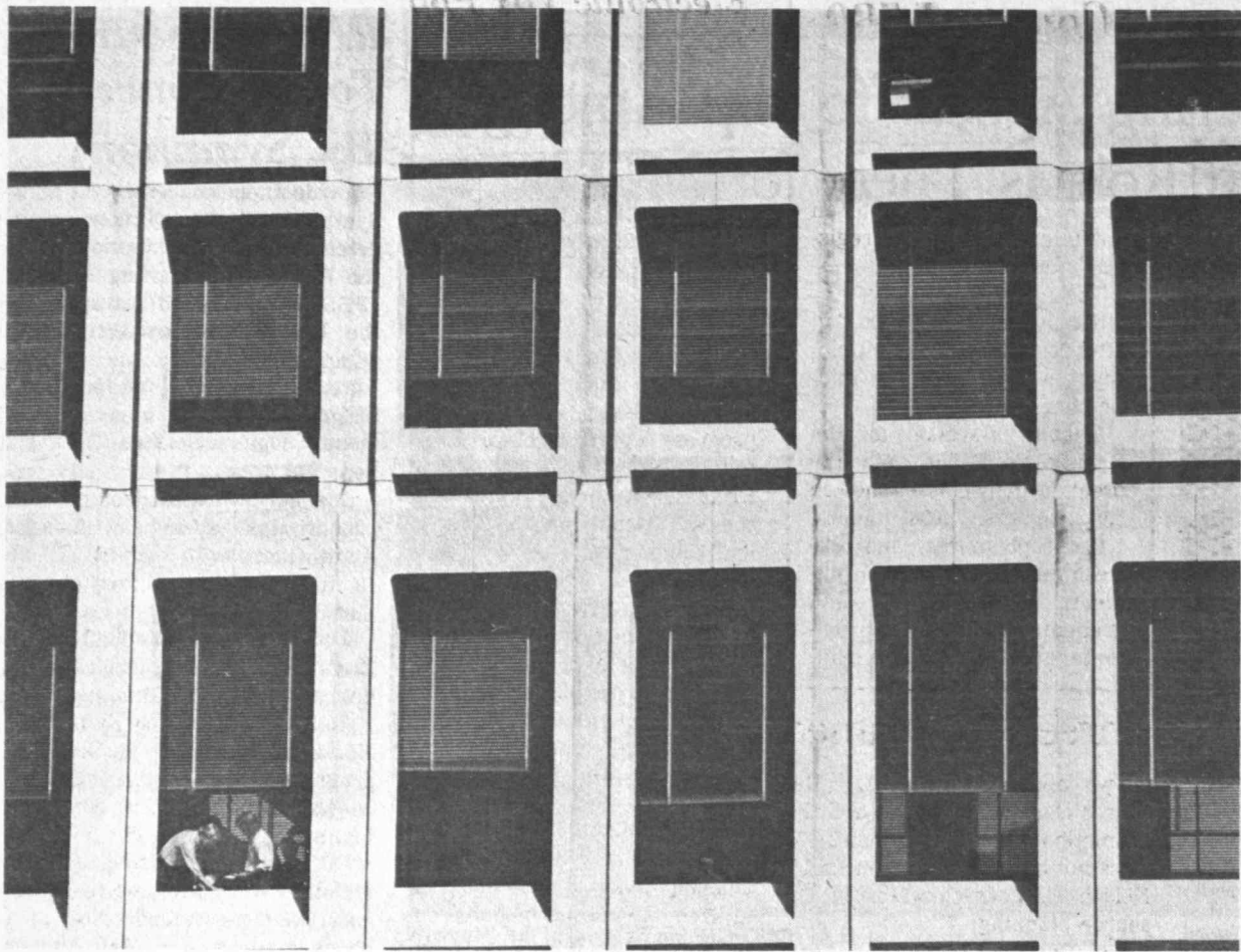
...of September shadows on Green Bldg. windows.
