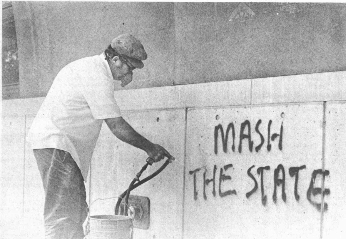
Graffiti removal has cost the Institute $22,647 between May, 1970 and May of this year. The sand blasting and washing necessary to remove paint from buildings sometimes leaves a discolored finish and there is a danger of actually exposing the
