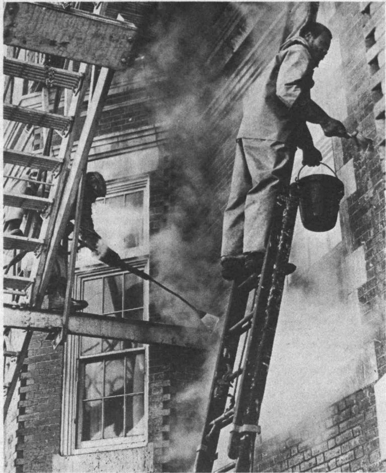
"Where there's smoke..." doesn't really apply in this case. The smoke here is steam, being used to clean the venerable facade of Ashdown house.
