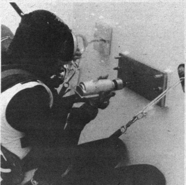
A diver holds himself in position to work by means of a belt and two storage magnets. He is drilling a tes specimen with a pneumatic impact wrench.
