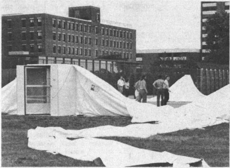
Spectators examine the deflated covering of the Carr Indoor Tennis Center. —Photo by Dave Searls, '73
