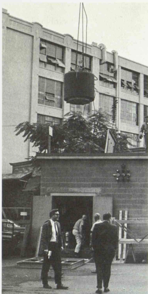
Bldg. 66's roof-top doors open wide to receive new cobalt-60 source.
