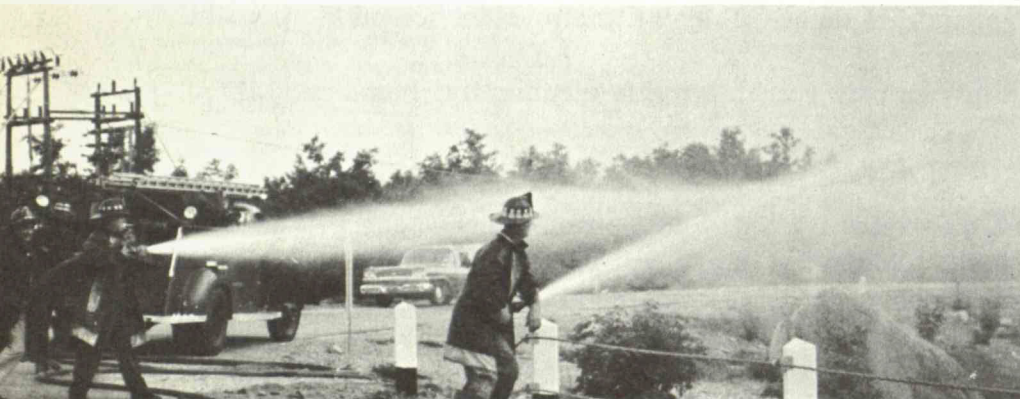
The Westford Fire Department pumper tests the performance of the hydrant and pond water supply at Millstone Hill.
