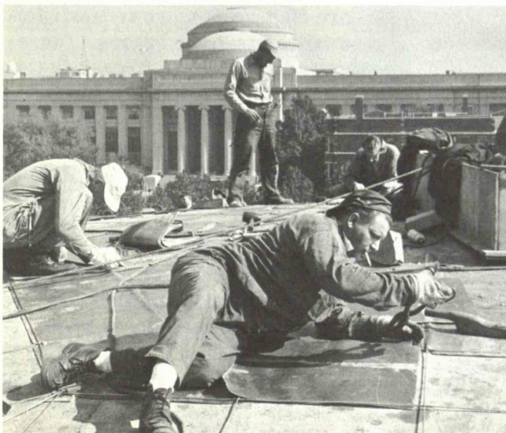
Busy on the roof
