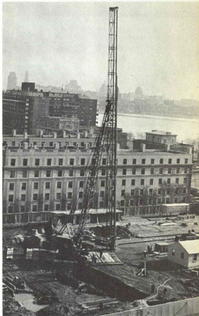
The pile driver.
