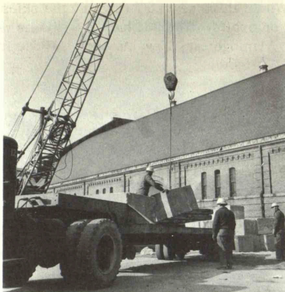
Test load arrives in two-ton blocks
