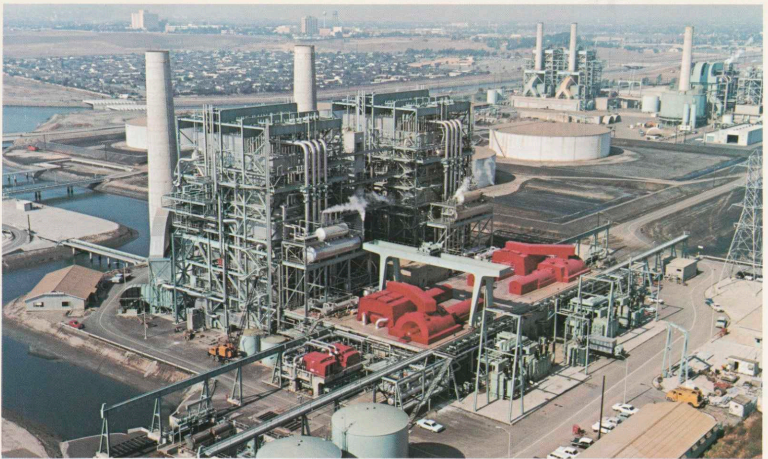
Southern California steam electric generating station has six units with a total capability of 1.9 million kilowatts.
