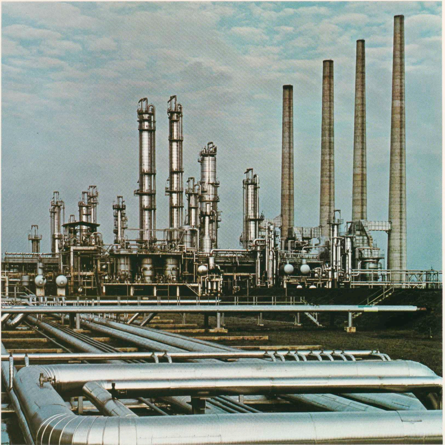
Eighteen months from design to start-up for a 100,000 barrels-per-day refinery, Belgium. The project also included a marine terminal and pipeline.
