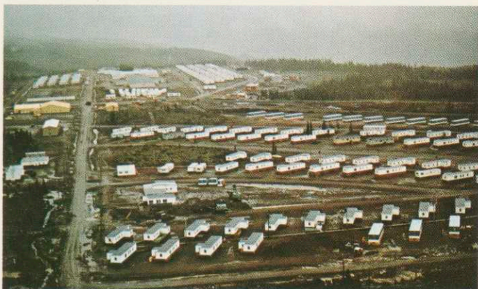
Grass-roots work camp and townsite, Labrador, with 20-man bunkhouses, mess and recreation halls, family trailers and auxiliary facilities.
