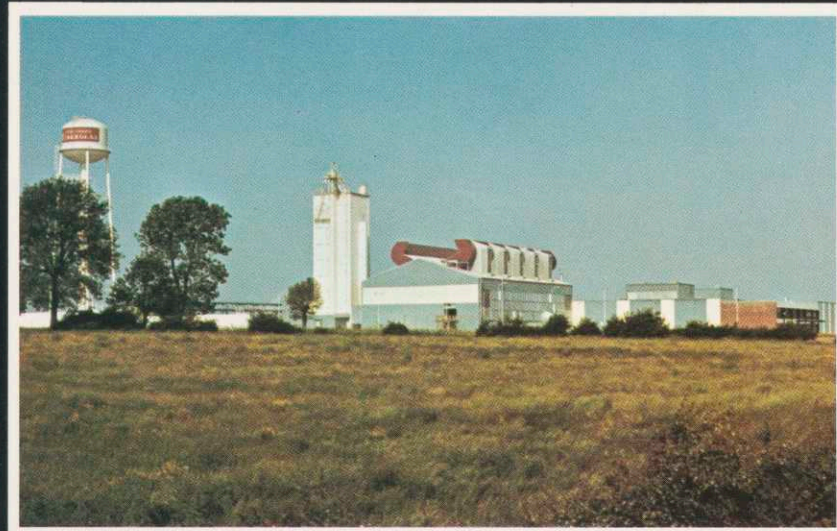
Glass fiber plant, Belgium, reflects capabilities for design of complex operations, and procurement services in the world markets.
