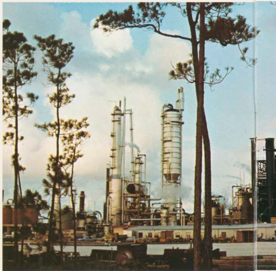
The world's largest single-train ammonia plant, Pascagoula, Mississippi, is rated at 1,500 tons-per-day.
