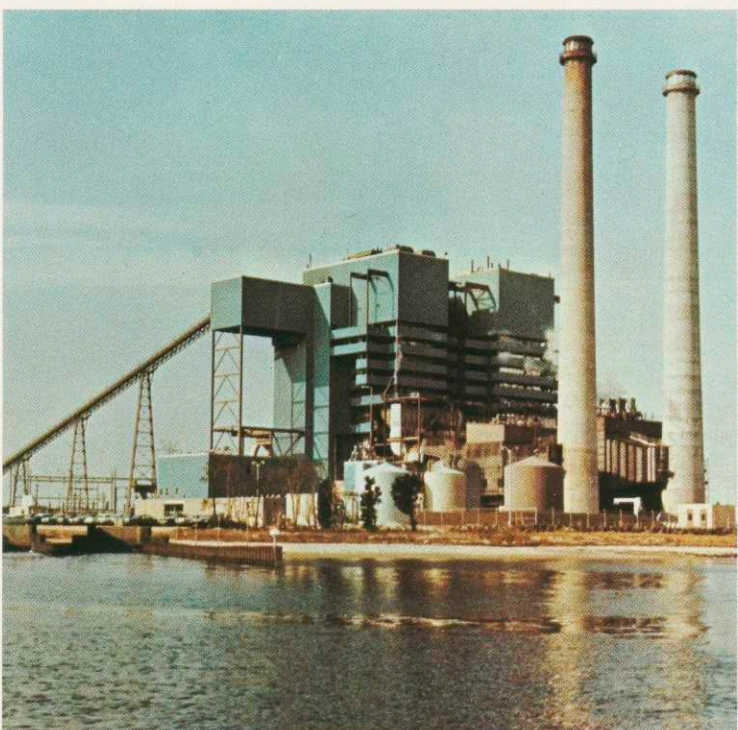
Conventional electric generating station, New Jersey, of which both units were turn-key responsibilities, features unit train coal handling.
