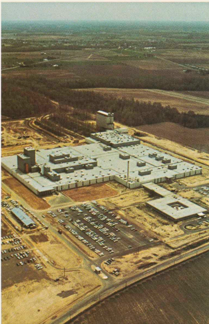
Food processing plant brought four existing plants, plus major expansions, into a single operation under the 20-acre roof.
