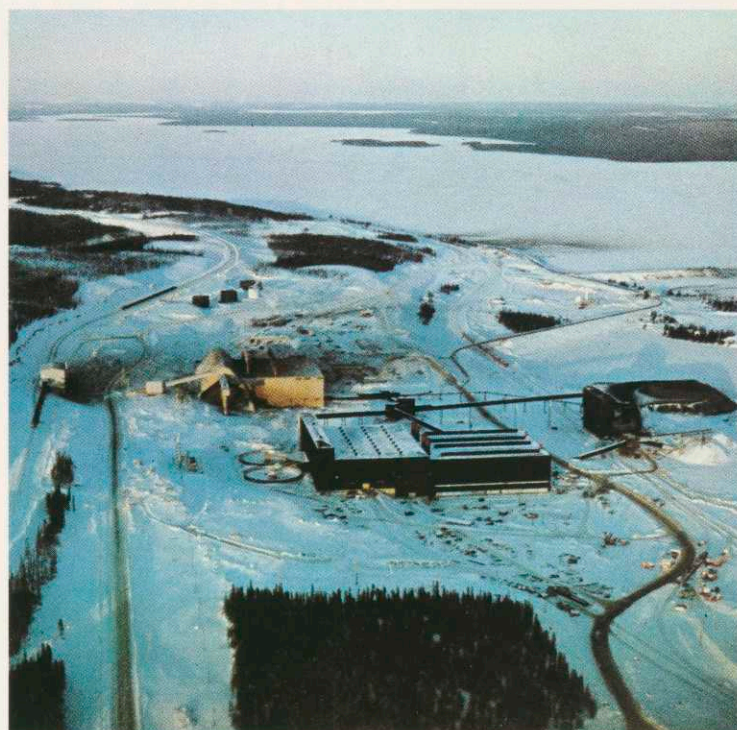
Iron ore complex, Labrador, has had numerous additions and expansions creating one of the world's largest facilities.
