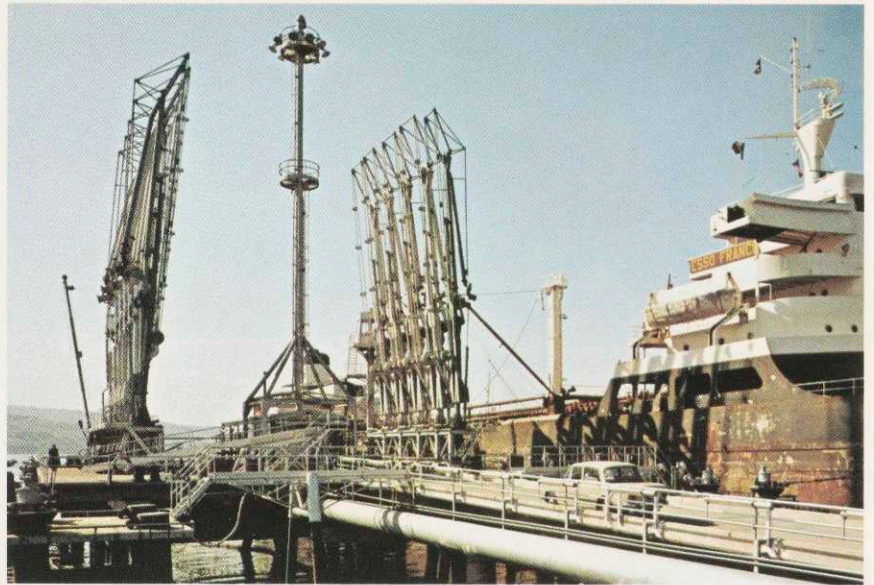
Petroleum pipeline marine terminal in northern Italy simultaneously berths four tankers of up to 160,000 deadweight tons.
