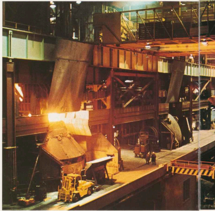
Many technological advances were combined to make the "Steel Mill of the Future" the first of its kind in the U.S., with construction by Bechtel.
