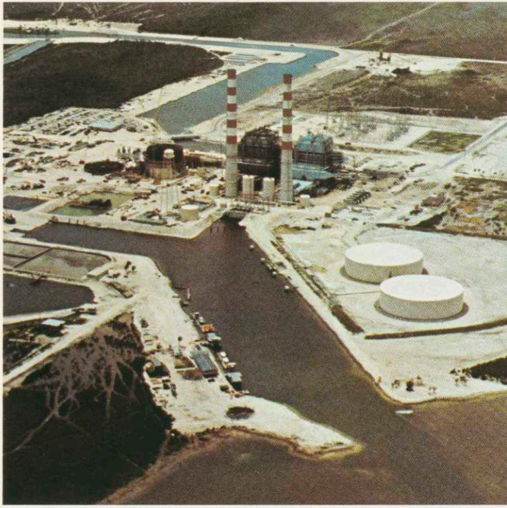
Electric generating station, Florida, combines two conventional and two nuclear units to total 2.3 million kilowatts.
