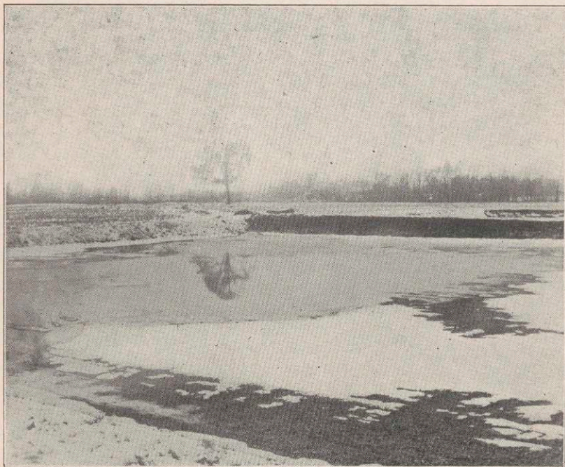
DIAGONAL VIEW ACROSS FILTER BED TOWARD CORNER WHERE SEWAGE EMPTIES. THE SEWAGE SINKS IN WITHOUT COVERING THE WHOLE BED. UNDISTURBED SNOW IN FOREGROUND. DIKE IN DISTANCE RUNNING IN DIRECTION OF TREE.
