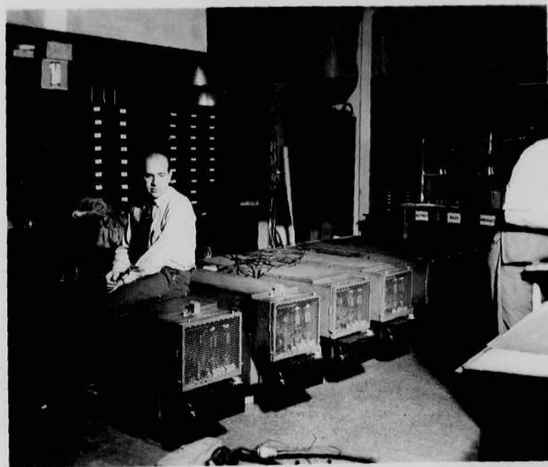
Fred Barston and D-3 unit which was installed in a B-24 Nov 17 1943 at Bedford airport.
