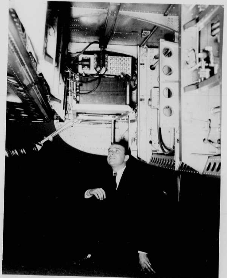
M-6. Set in place.
