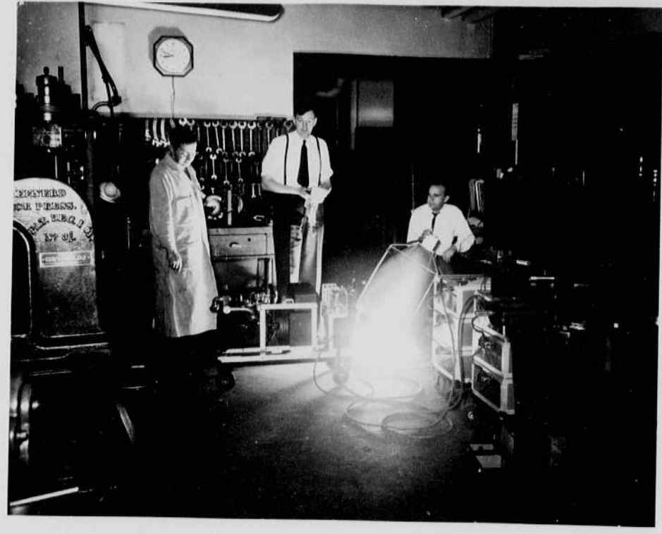
Test in Shop, before installation
