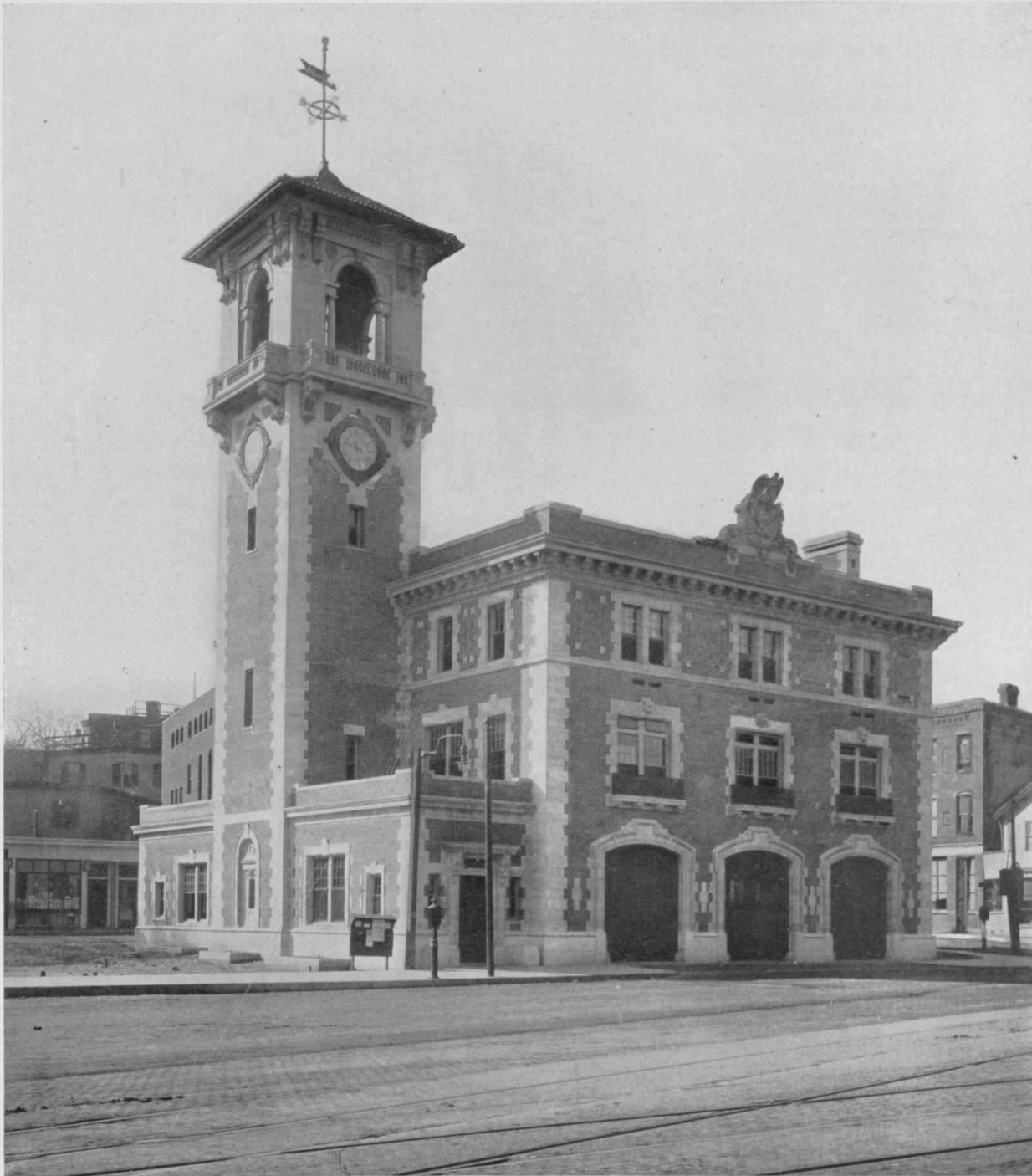
FIRE STATION, BROOKLINE, MASS.
