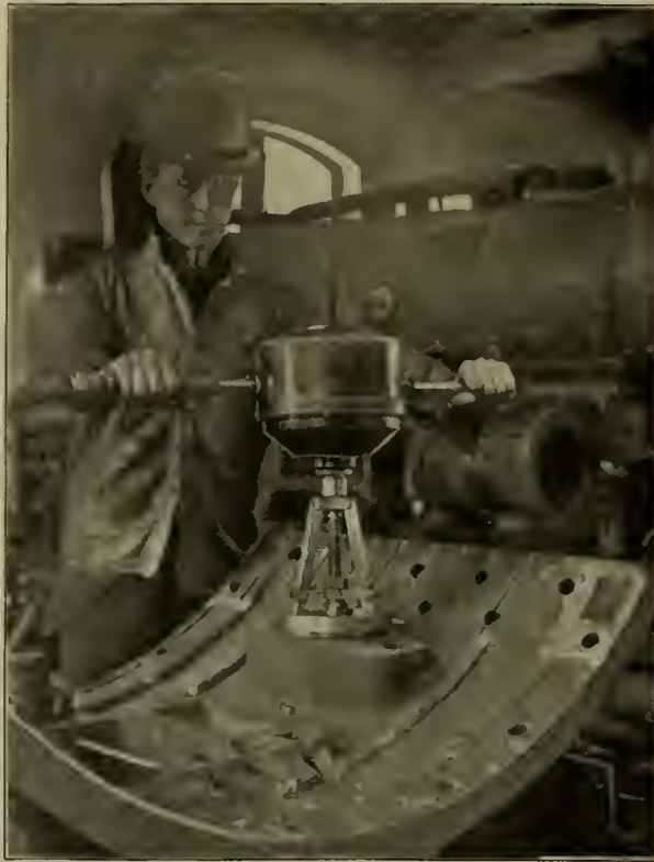
GRINDING STEAM PIPE JOINT IN CYLINDER SADDLE.
