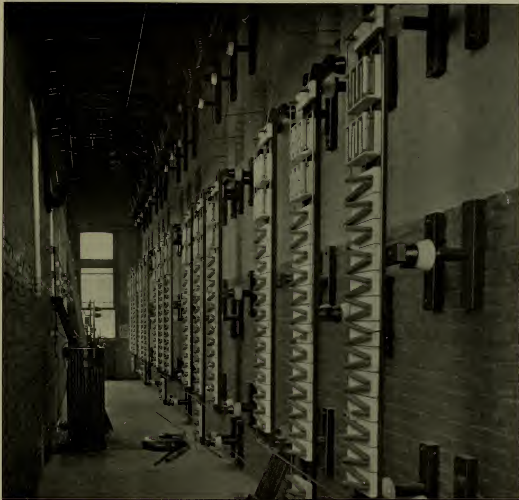
FIG. II.—THE LIGHTNING ARRESTER ROOM IN THE SUB-STATION AT NEWFIELD, SHOWING ALSO THE DISCONNECTING SWITCHES
