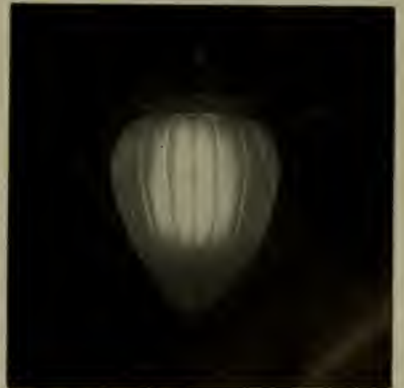
A GLOBE WITH A GROUND GLASS INTERIOR. THIS GIVES A FAIRLY GOOD DIFFUSION
