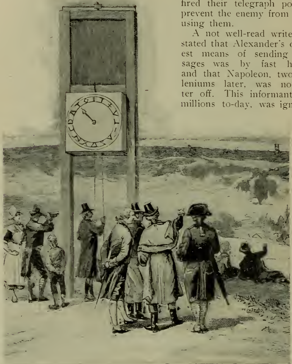
CHAPPE'S FIRST APPARATUS, 1792
