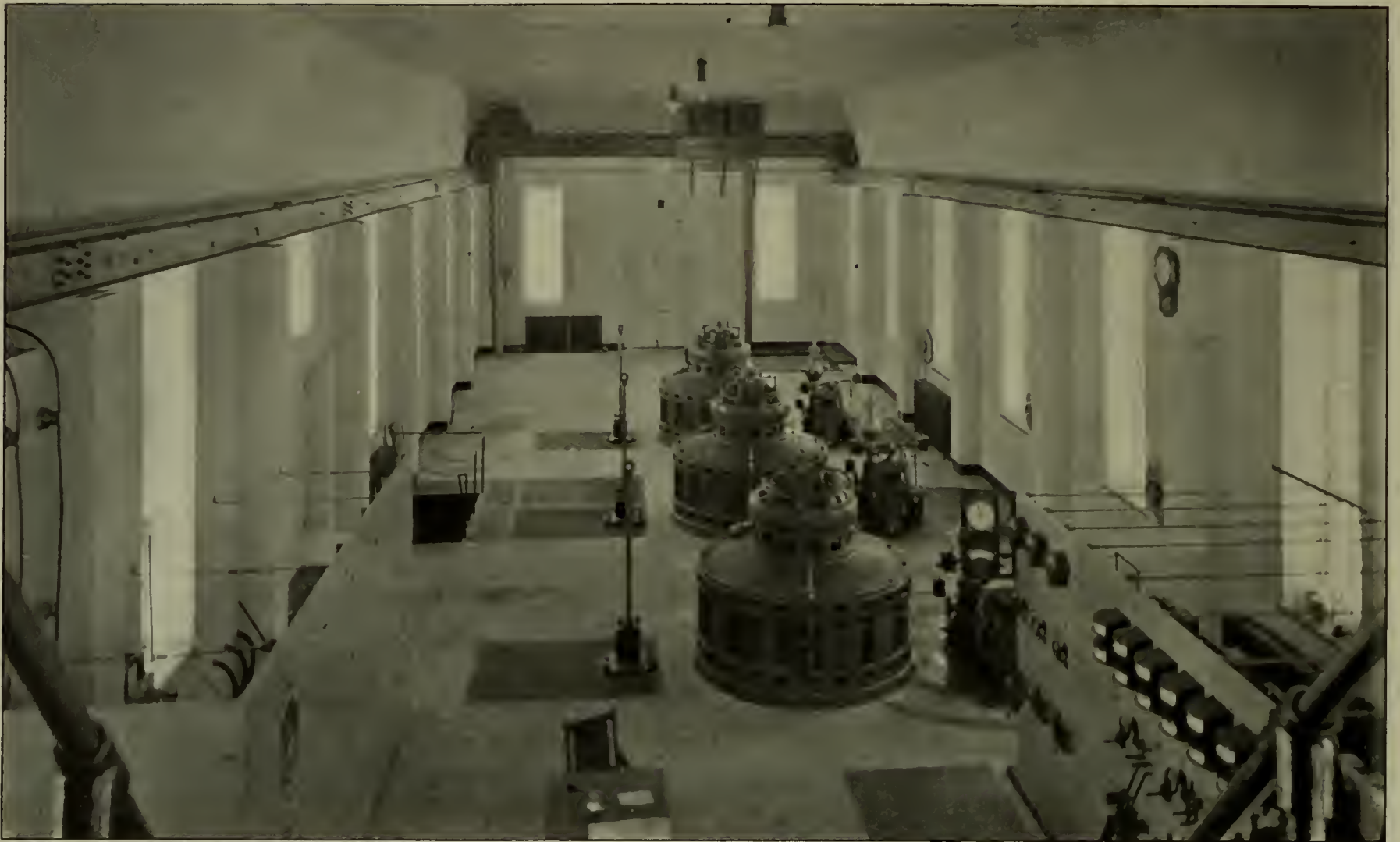
FIG. 2.—INTERIOR OF THE POWER HOUSE OF THE VERMONT MARBLE COMPANY AT PROCTOR. THREE 750-KW., 3-PHASE GENERATORS, BUILT BY THE GENERAL ELECTRIC COMPANY, OF SCHENECTADY, N. Y., ARE DRIVEN BY TURBINES BUILT BY THE I. P. MORRIS COMPANY, OF PHILADELPHIA
