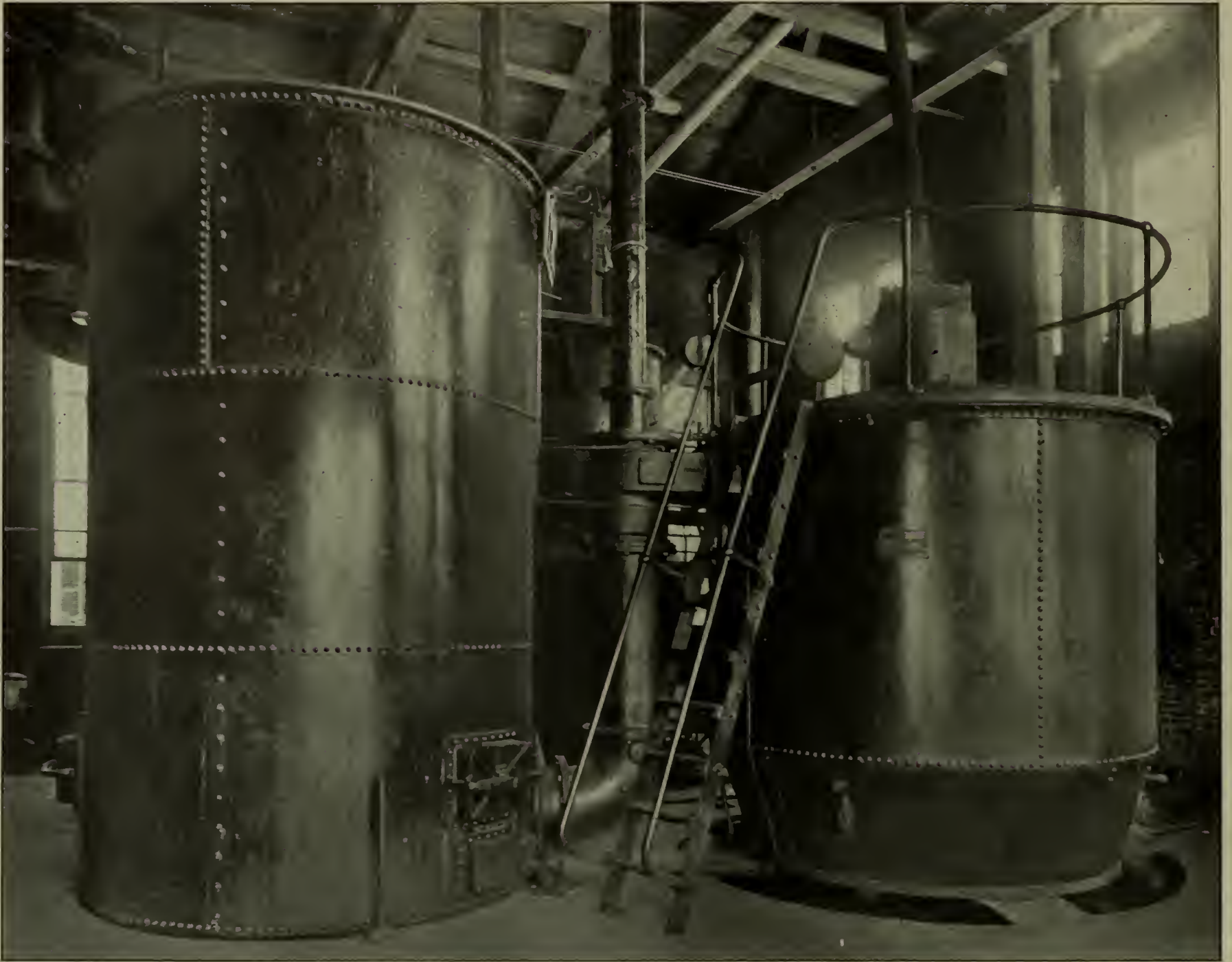
A PART OF THE GAS-PRODUCER PLANT OF THE CITIZENS' ELECTRIC COMPANY. TWO 250-H. P. SETS ARE INSTALLED, ONE BEING SHOWN HERE. ON THE RIGHT IS THE PRODUCER SHELL, WITH THE COAL-CHARGING HOPPER ON TOP. ON THE LEFT IS THE SCRUBBER
