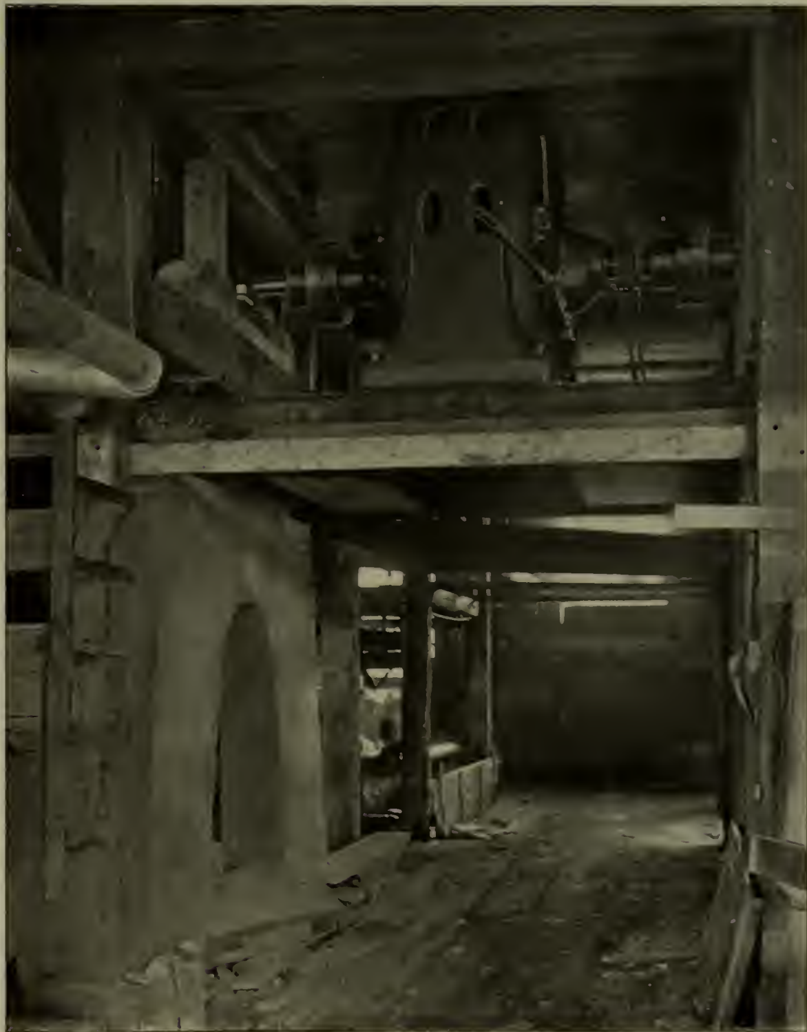
FIG. 5.—A 250-H. P. INDUCTION MOTOR DRIVING A LINE SHAFT IN THE MARBLE-SAWING MILL
