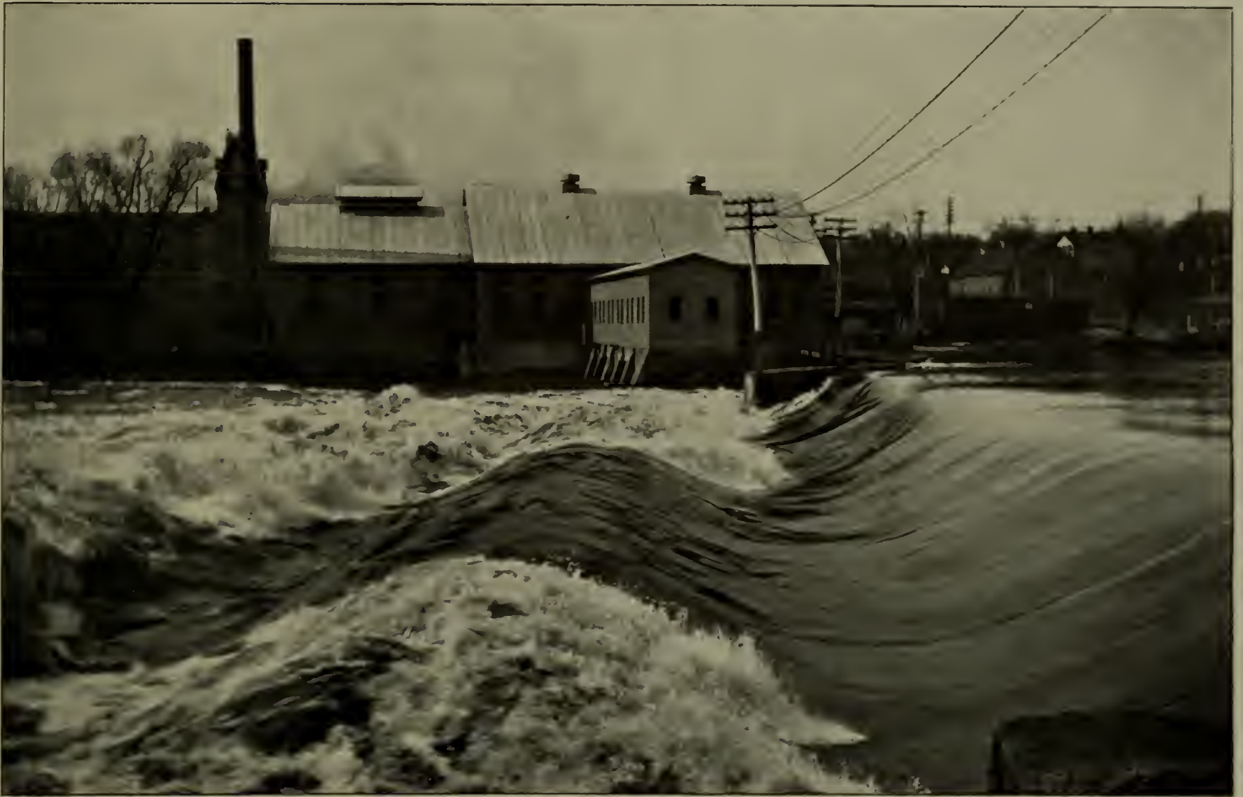
FIG. 5.—THE UPPER DAM AND CENTRAL PLANT OF THE JANESVILLE ELECTRIC COMPANY AFTER COMPLETION
