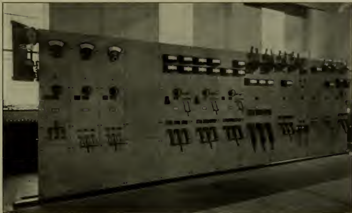
FIG. 4.—THE SWITCHBOARD AT THE PROCTOR POWER HOUSE. SO EXTENSIVE IS THE ELECTRIC EQUIPMENT IN THE COMPANY'S PLANT THAT THIRTEEN PANELS, ONE FOR FUTURE USE, ARE REQUIRED FOR THE INSTRUMENTS AND SWITCHES
