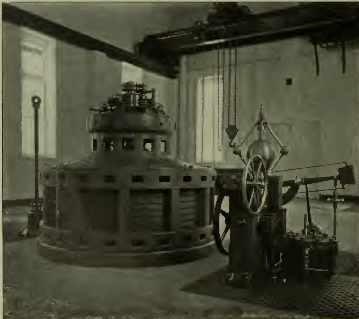
FIG. 3.—A NEARER VIEW OF ONE OF THE GENERATORS AND A WATER-WHEEL GOVERNOR
