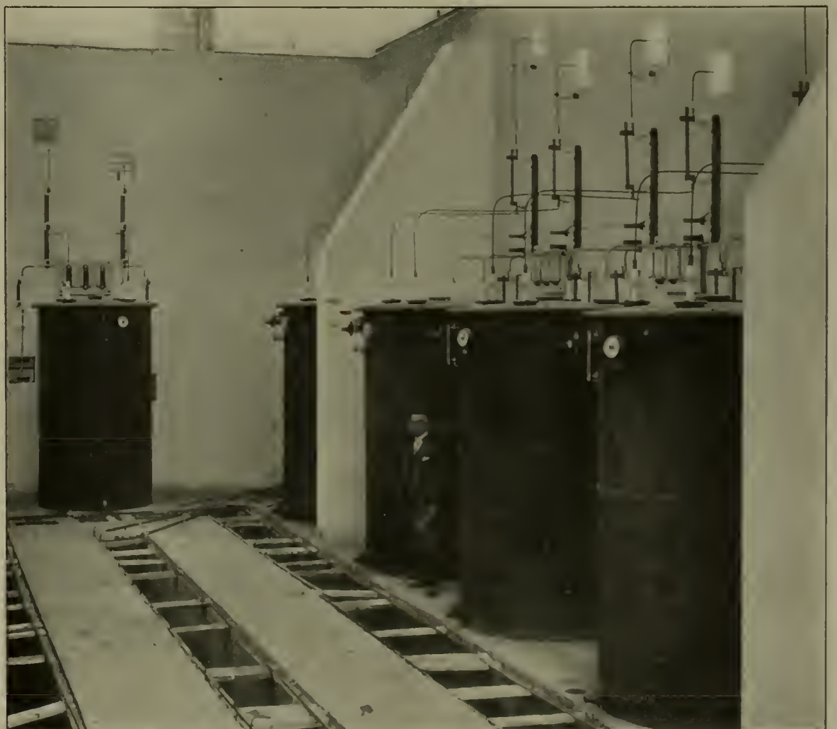
FIG. 9.—SINGLE-PHASE TRANSFORMERS AT THE CELLINA RIVER PLANT FOR RAISING THE PRESSURE FROM 4000 TO 36,000 VOLTS. FIVE GROUPS OF THREE SINGLE-PHASE TRANSFORMERS ARE INSTALLED
