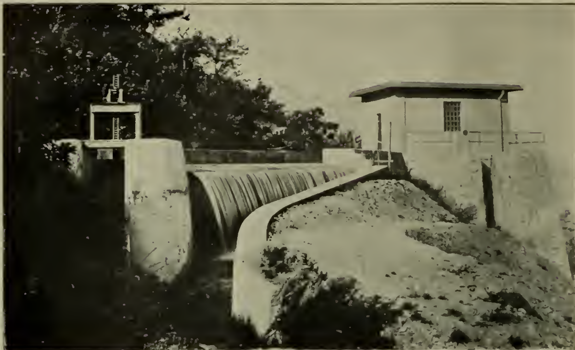
FIG. 4.—THE END OF THE CONDUIT FROM THE MAROEBIA RIVER AND THE GATE HOUSE FROM WHICH THE PENSTOCK CONVEYS THE WATER TO THE POWER PLANT
