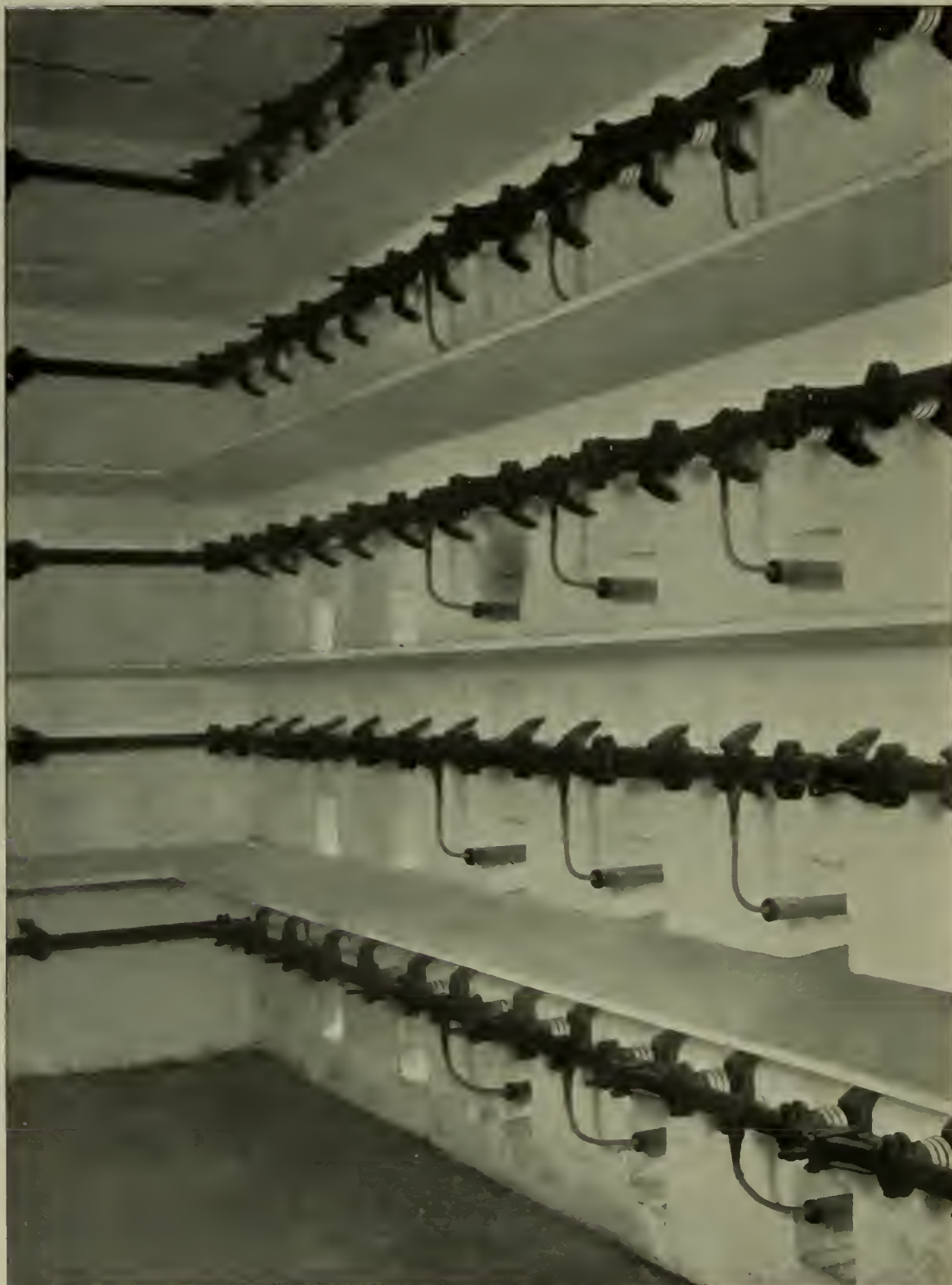
FIG. 5.—BUS-BARS IN THE VENICE SUB-STATION, WHICH RECEIVES CURRENT FROM THE POWER PLANT AT MONTEREALE
