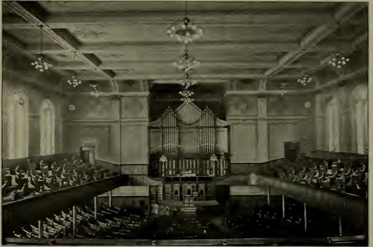
A GOOD CHANDELIER INSTALLATION IN A CHURCH
