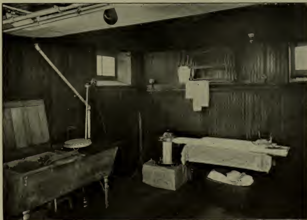
THE LAUNDRY, SHOWING FLATIRON, WASH-BOILER AND IMMERSION-COIL HEATER
