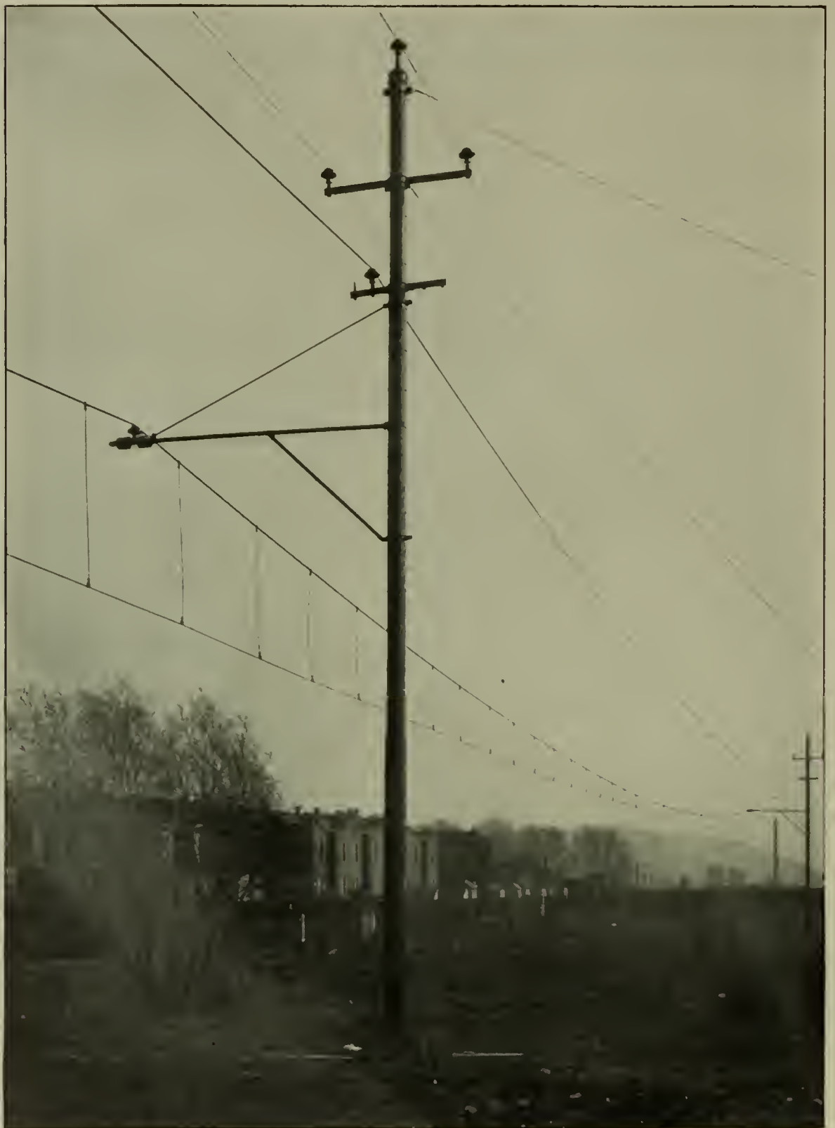
FIG. 1.—GENERAL VIEW OF THE EXPERIMENTAL LINE FOR TESTING OVERHEAD CATENARY CONSTRUCTION, ERECTED BY ELMER P. MORRIS, NEW YORK, REPRESENTING THE ELECTRIC RAILWAY EQUIPMENT COMPANY, CINCINNATI, OHIO
