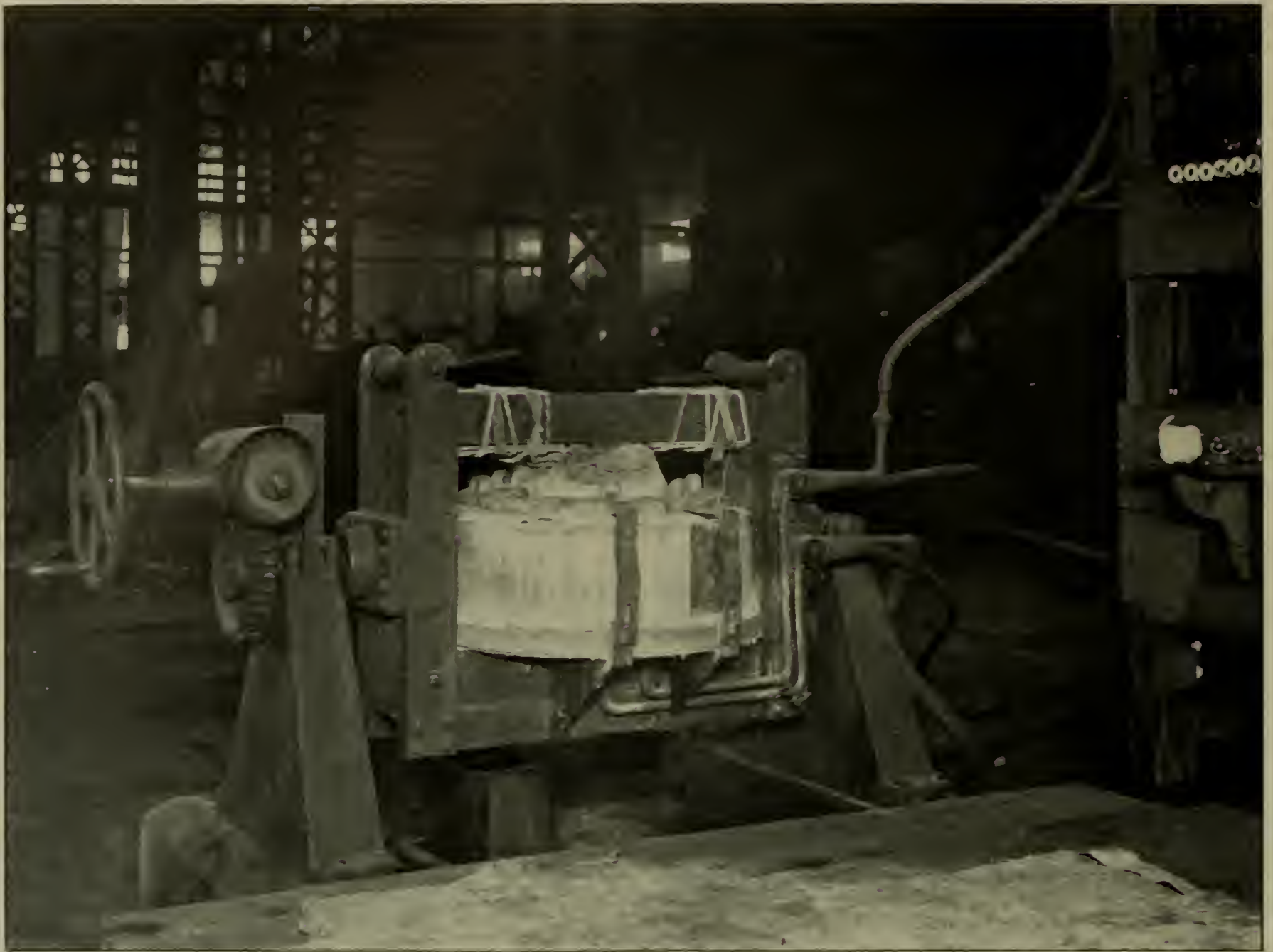
FIG. 1.—AN ELECTRIC STEEL FURNACE OPERATED ON CENTRAL STATION CURRENT. IT IS OF THE INDUCTION TYPE AND OF 131-KILOVOLT-AMPERE CAPACITY. SINGLE-PHASE, 60-CYCLE CURRENT IS SUPPLIED AT 240 VOLTS
