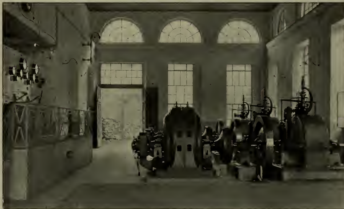
FIG. 2.—INTERIOR OF THE HYDRO-ELECTRIC PLANT ON THE MAROBBIA RIVER IN SWITZERLAND. CURRENT IS GENERATED BY THREE 490-KW. MACHINES AT 5350 VOLTS
