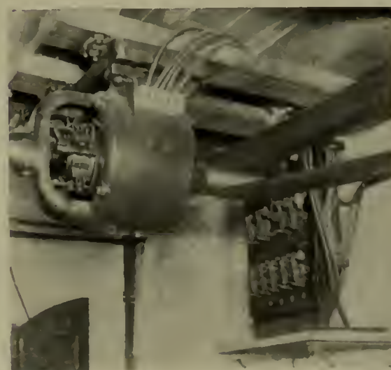
AN ELEVATOR CONTROLLER ATTACHED TO A SIDE WALL
