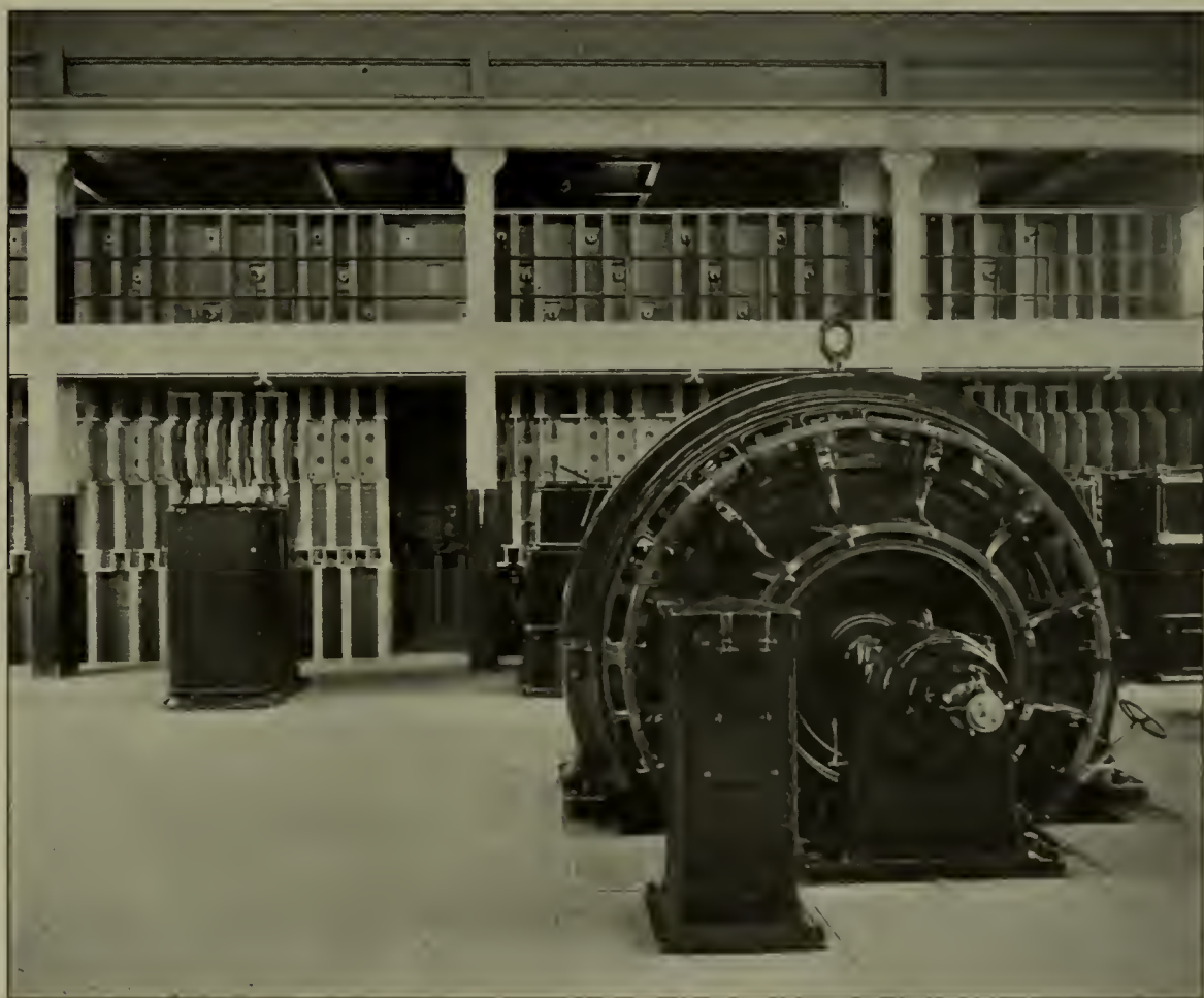
FIG. 12.—AN INTERIOR VIEW OF PART OF THE SUB-STATION AT WOODHAVEN JUNCTION LOOKING TOWARD THE HIGH-TENSION GALLERY
