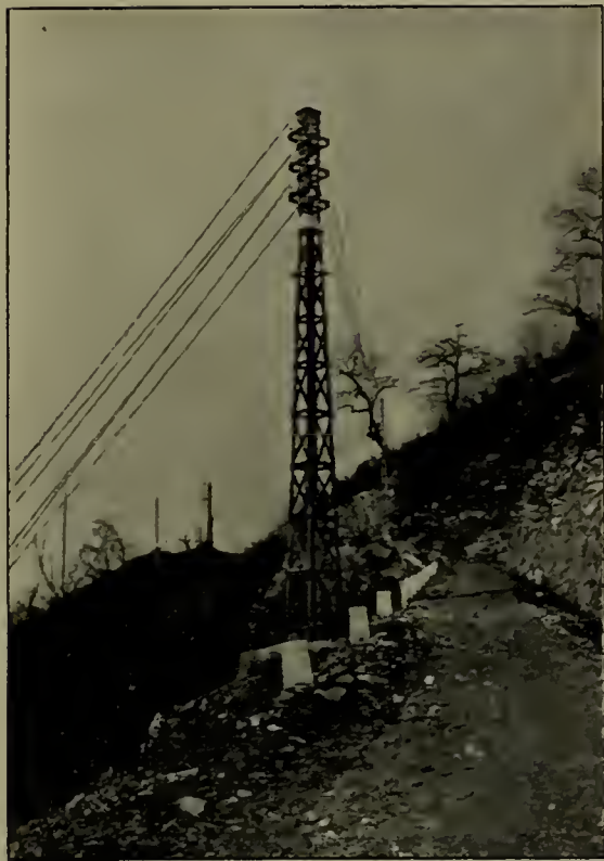
FIG. 1.—PART OF THE TRANSMISSION LINE IN SWITZERLAND, FROM GIUBIASCO TO BELLINZONA
