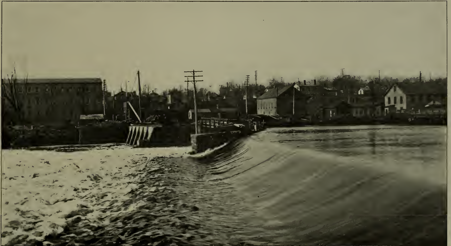
FIG. 1.—VIEW OF THE UPPER DAM WHILE THE CENTRAL PLANT OF THE JANESVILLE ELECTRIC COMPANY WAS BEING CONSTRUCTED. THIS IS ONE OF THREE PLANTS OWNED BY THE COMPANY, TWO BEING USED FOR NORMAL SERVICE AND ONE FOR PEAK LOADS
