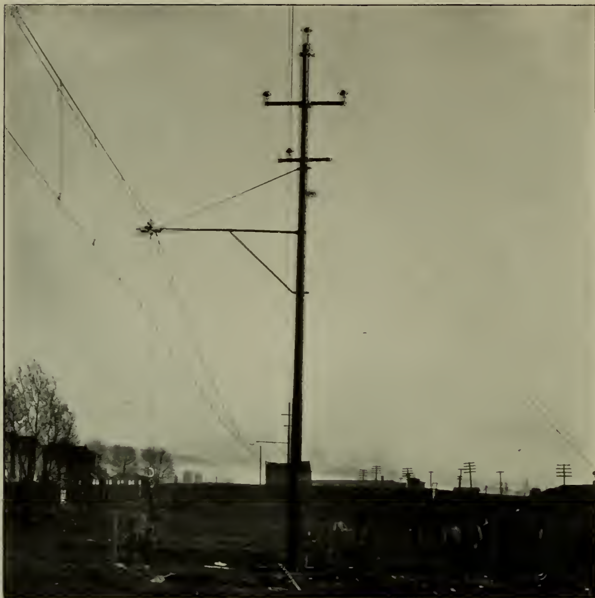
FIG. 4.—APPEARANCE OF THE EXPERIMENTAL LINE UNDER A DOWNWARD STRAIN OF 2000 POUNDS ON THE END OF THE BRACKET
