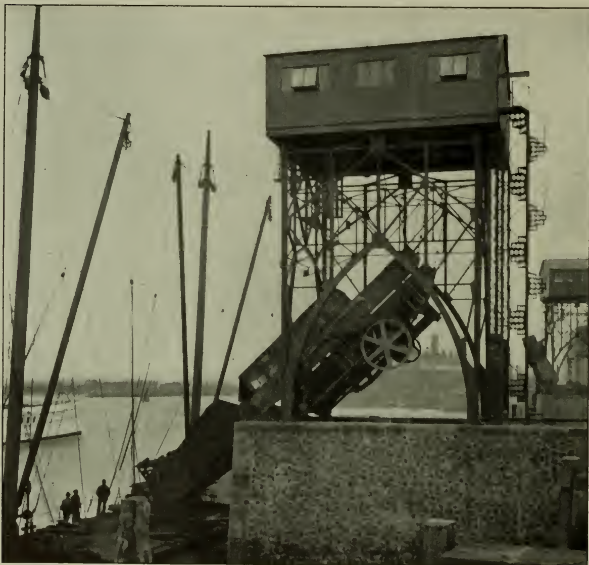
FIG. 3.—FOR HIGH-WATER LEVELS, THE TIP IS OPERATED BY ELECTRICITY
