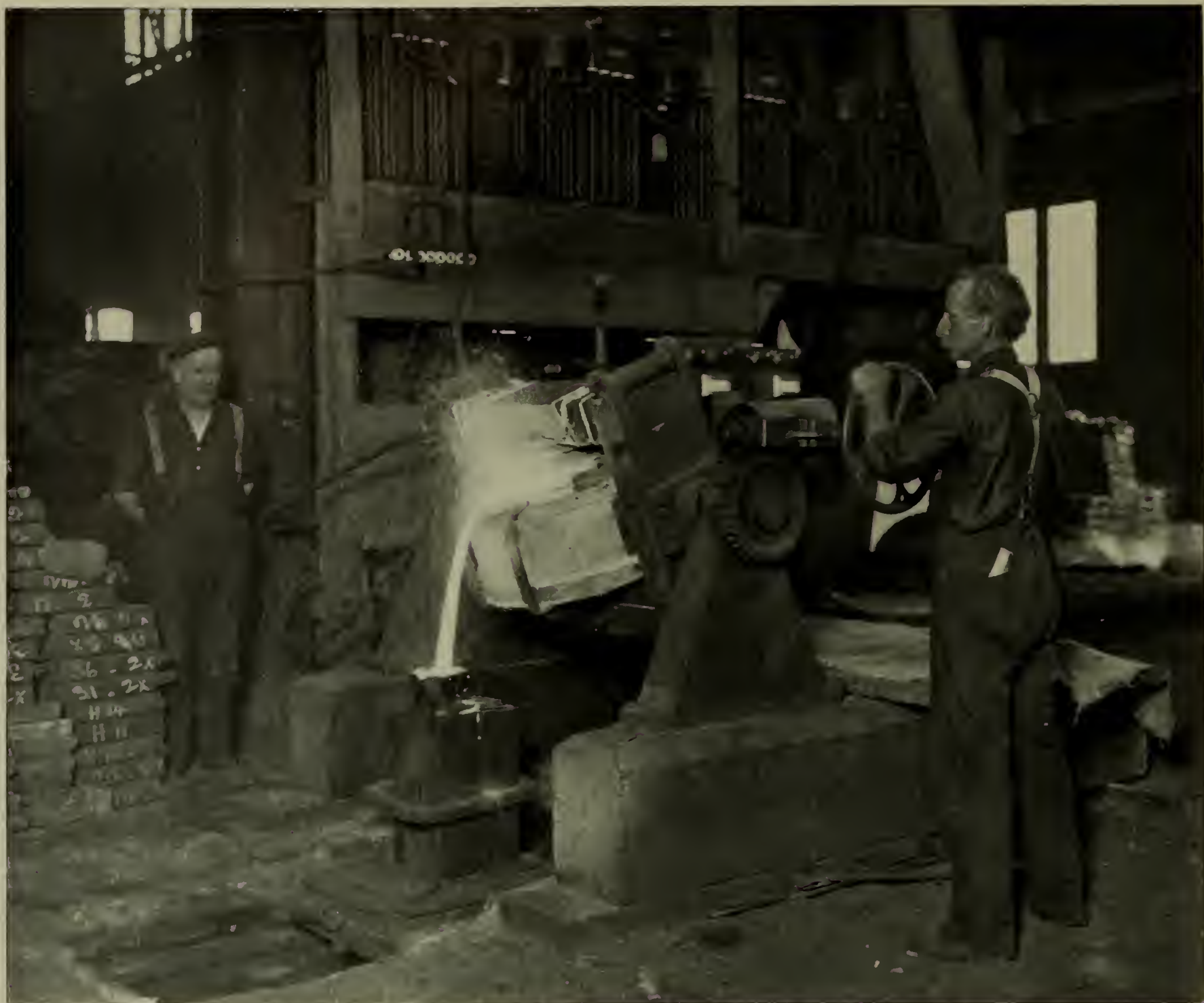
FIG. 3.—POURING MOLTEN STEEL FROM THE ELECTRIC FURNACE SHOWN IN FIG. 1.
