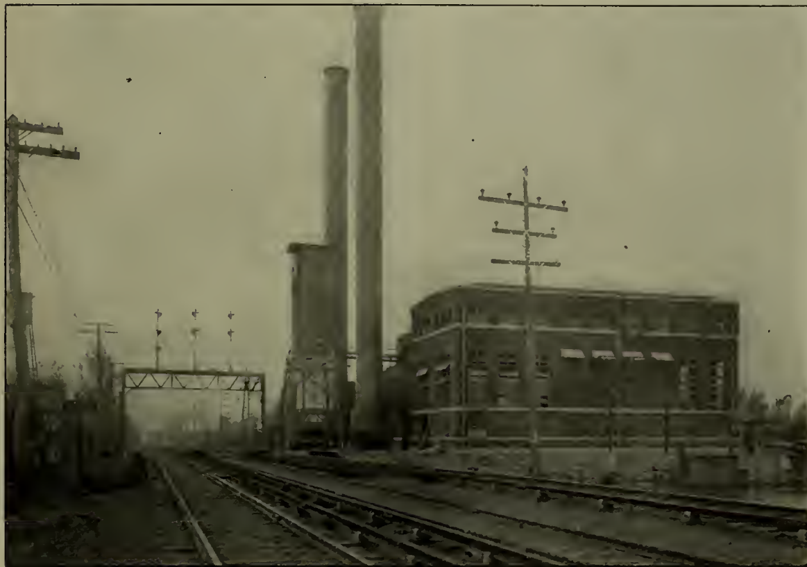
FIG. 1.—THE POWER HOUSE OF THE WEST JERSEY & SEASHORE RAILROAD AT WESTVILLE, N. J.
