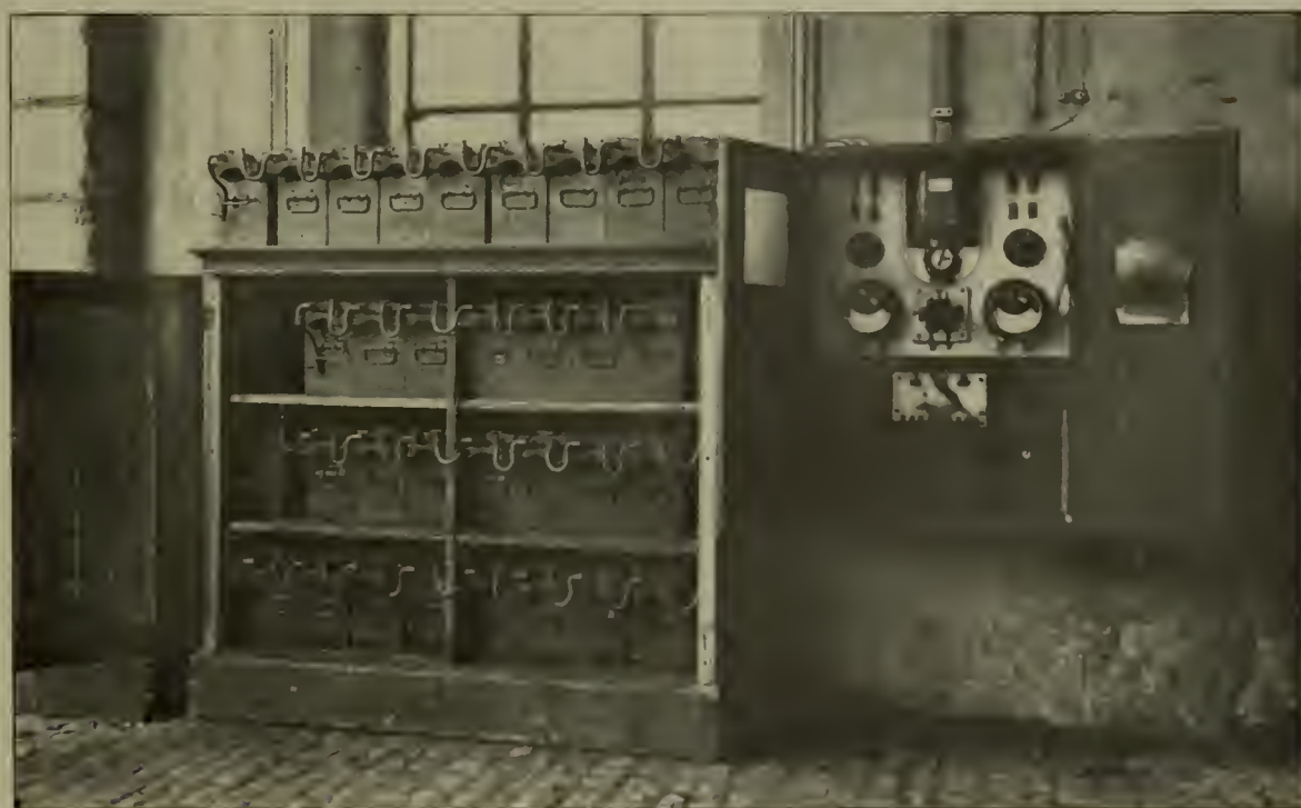
FIG. 2.—INTERIOR OF CAR LIGHTING STORAGE BATTERY CHARGING STATION AT PRAGUE
