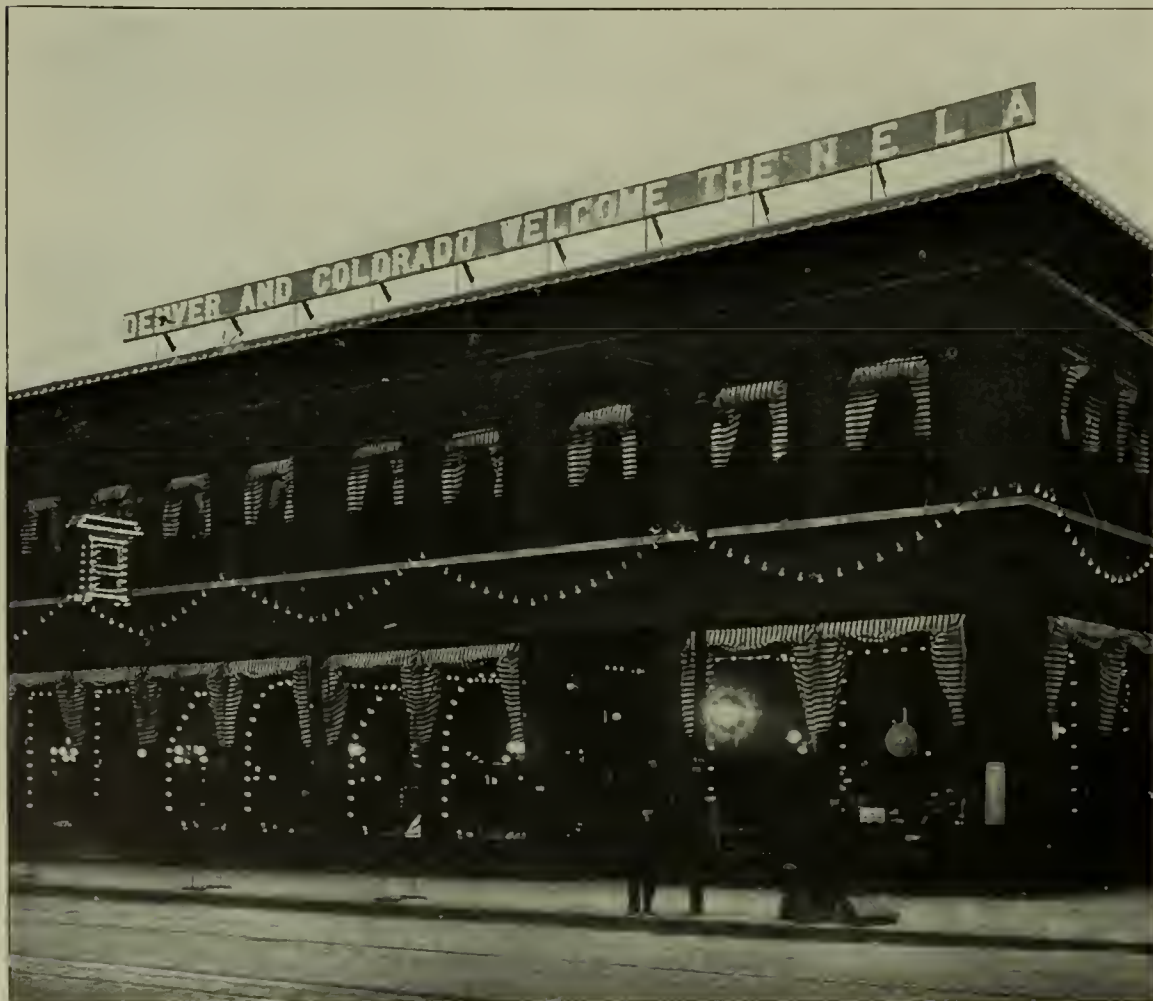
A SIGN BUILT BY THE MOBILE ELECTRIC COMPANY, OF NEWARK, N. J., AND PLACED ON THE ROOF OF THE DENVER GAS & ELECTRIC COMPANY'S BUILDING DURING THE NATIONAL ELECTRIC LIGHT CONVENTION LAST YEAR
