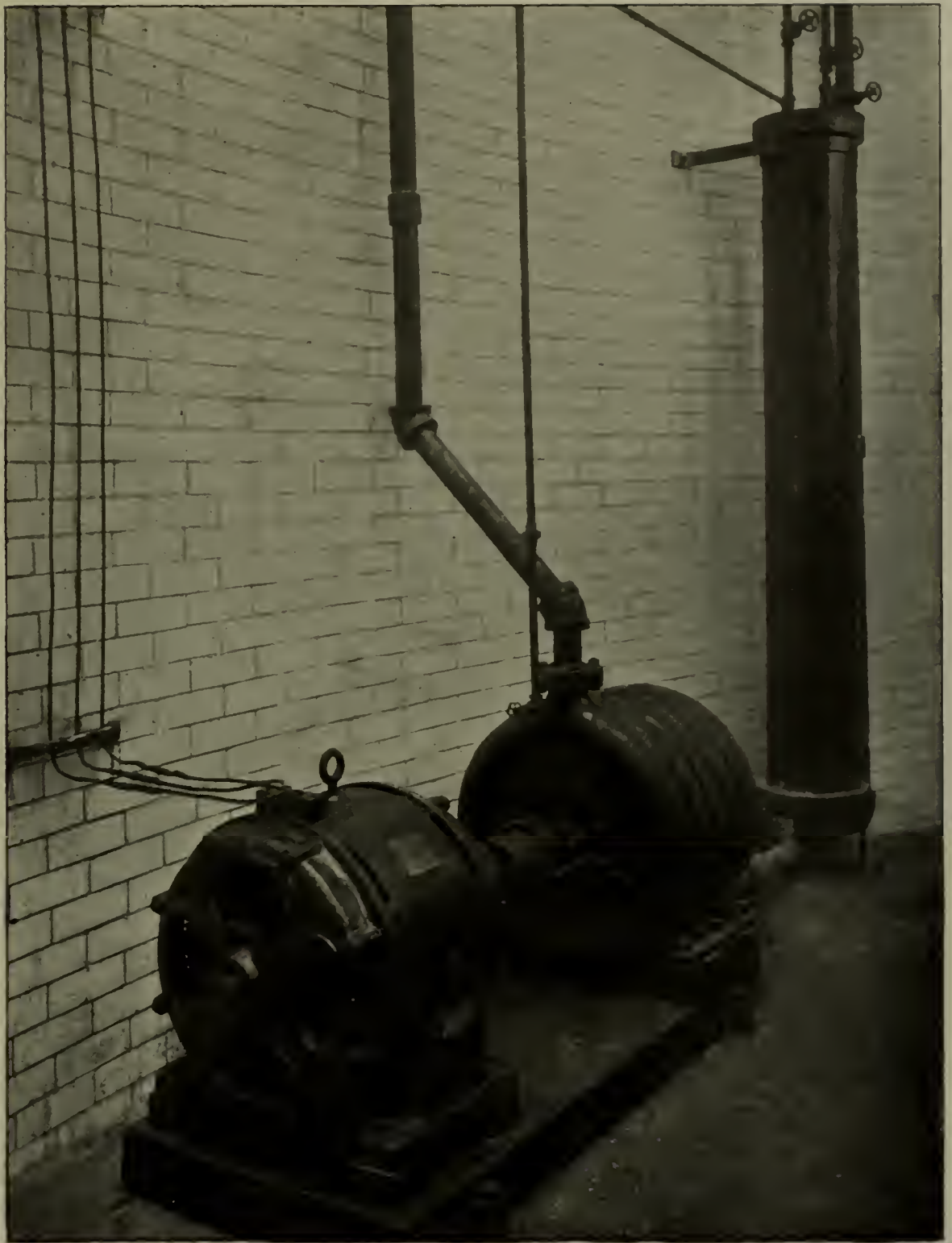
FIG. 3.—A 5-STAGE MOTOR-DRIVEN WORTHINGTON PUMP SUPPLYING WATER AT 200 POUNDS PRESSURE FOR OPERATING THE HYDRAULIC VALVES
