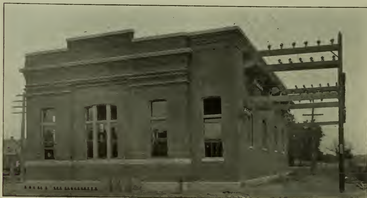
FIG. 10.—EXTERIOR OF THE SUB-STATION AT GLASSBORO
