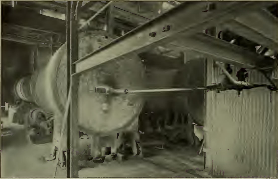
A MOTOR-DRIVEN KILN. THE PIPE EXTENDING INTO THE OPENING IN FRONT IS FOR FEEDING PULVERIZED COAL
