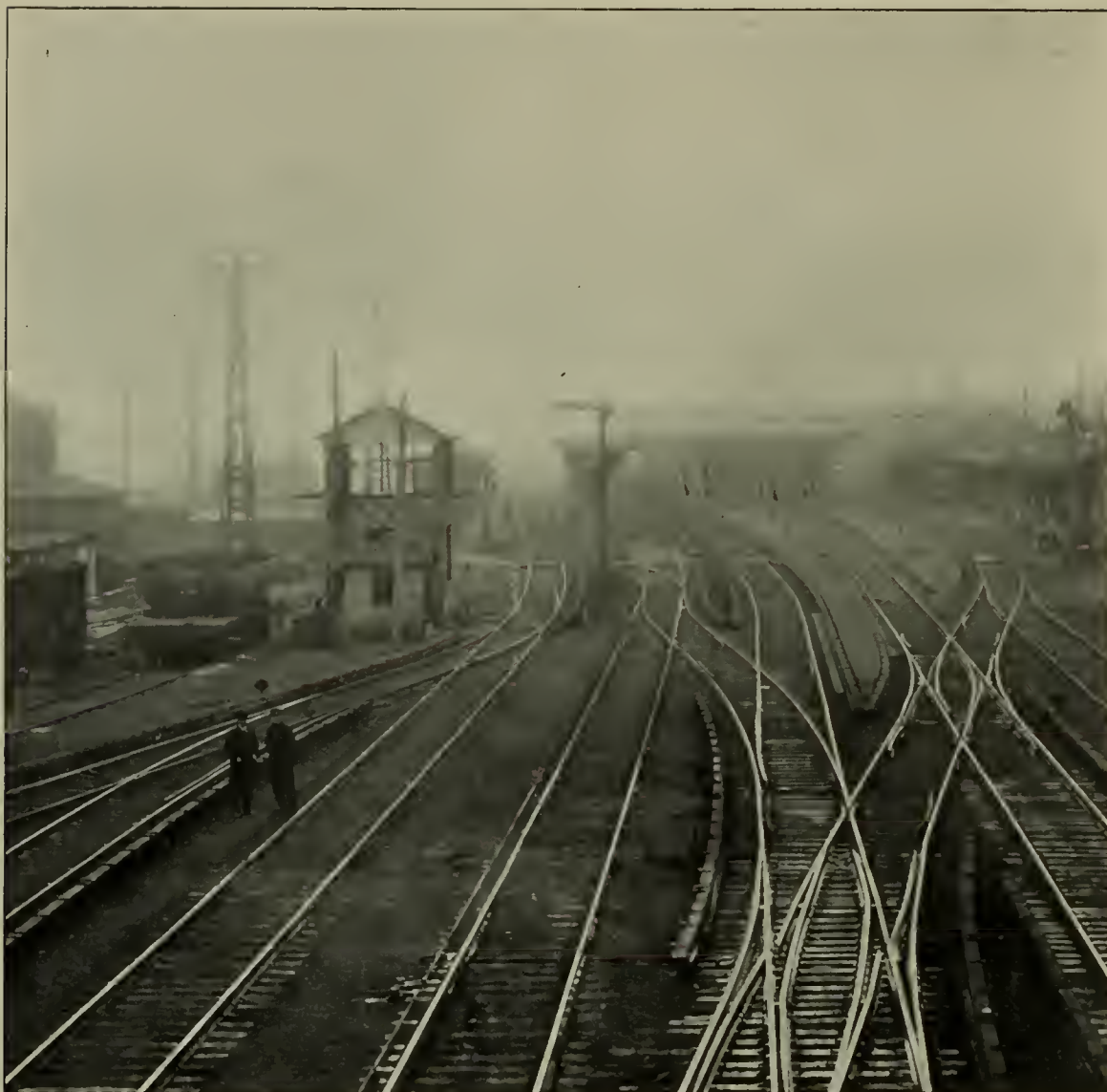
FIG. 8.—VIEW NEAR JAMAICA STATION, SHOWING THE THIRD RAIL AT AN INTERLOCKING JOINT
