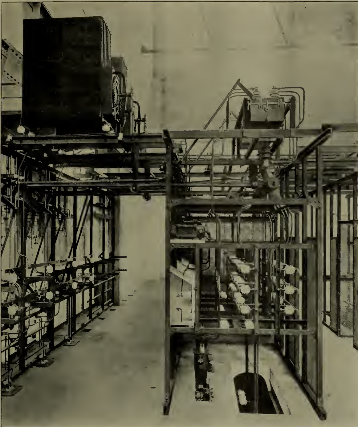
FIG. 22.—OIL SWITCHES IN THE GLOMMEN RIVER PLANT
