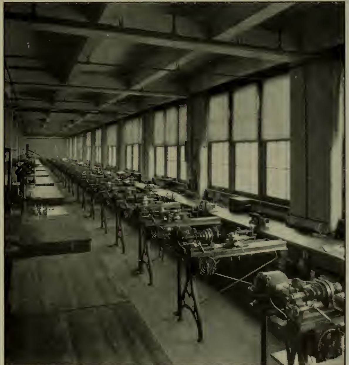
TWO VIEWS OF THE BRASS DEPARTMENT OF THE BAUSH, LOMB, SAEGMULLER COMPANY, OF ROCHESTER, N. Y., SHOWING THE INCREASED LIGHT AND CLEANLINESS, DUE TO THE MACHINES BEING DRIVEN BY MOTORS BUILT BY THE ROCHESTER ELECTRIC MOTOR COMPANY
