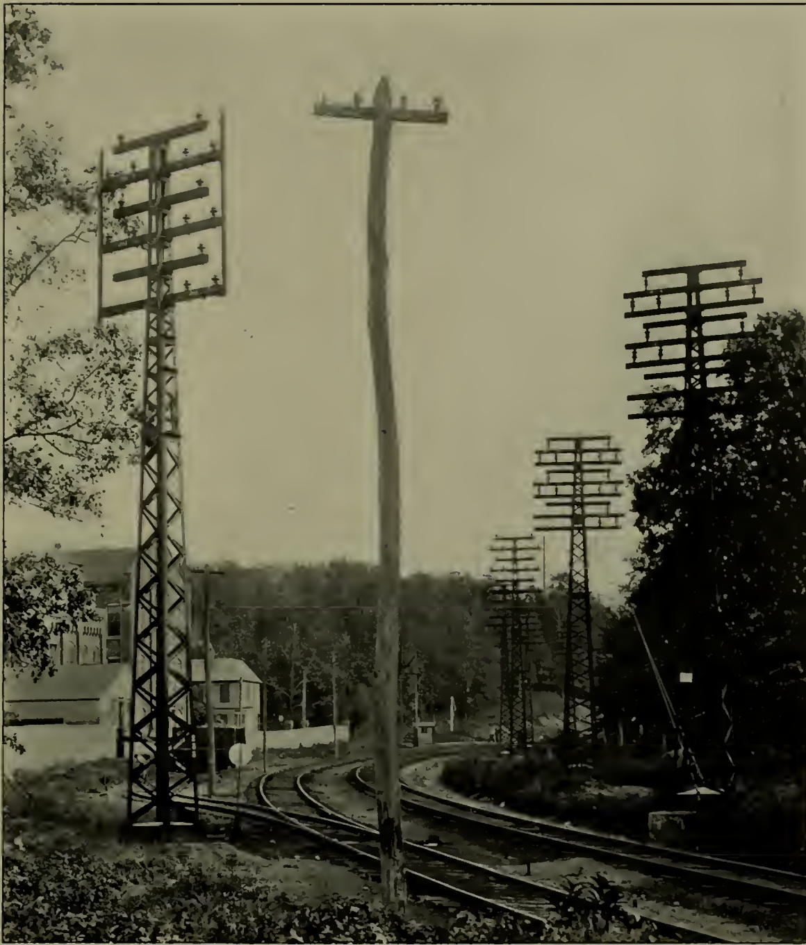
FIG. 1.—THE TRANSMISSION LINE OF THE LONG ISLAND RAILROAD CROSSING A TRACK. THE CABLE RETAINERS ARE SHOWN ON THE POLE AT THE LEFT
