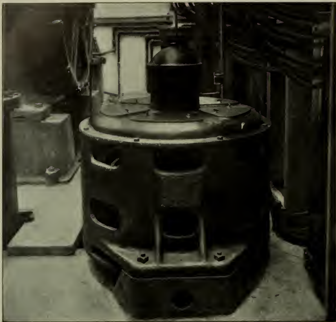
FIG. 4.—A 75-H. P. VERTICAL MOTOR DRIVING A DRAINAGE PUMP
