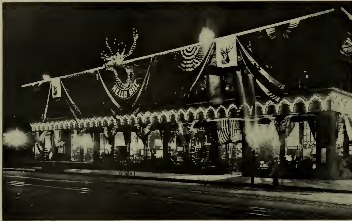
ILLUMINATION OF THE OFFICES OF THE DENVER GAS &amp; ELECTRIC COMPANY
