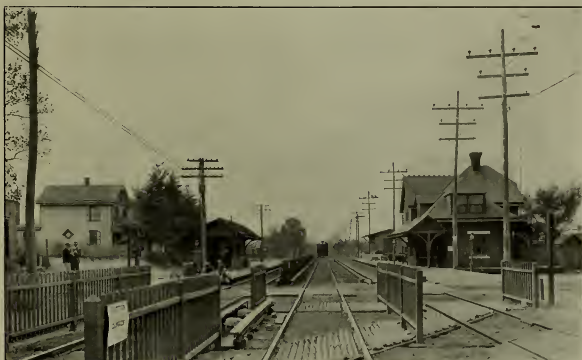
FIG. 2.—THE STATION AT WESTVILLE, SHOWING CATTLE GUARDS, JUMPER BOXES, AND THIRD-RAIL COVERING
