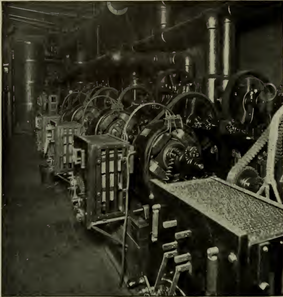
THE REFRIGERATING APPARATUS IS DRIVEN BY WESTINGHOUSE MOTORS
