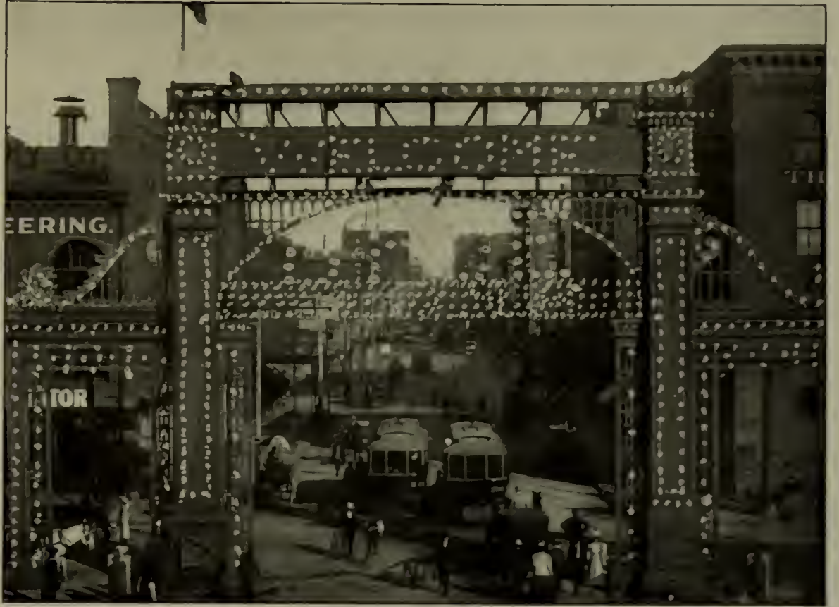
AN ELECTRIC ARCH IN COURSE OF ERECTION BY THE DENVER GAS & ELECTRIC COMPANY FOR THE "ELKS" CONVENTION AT DENVER
