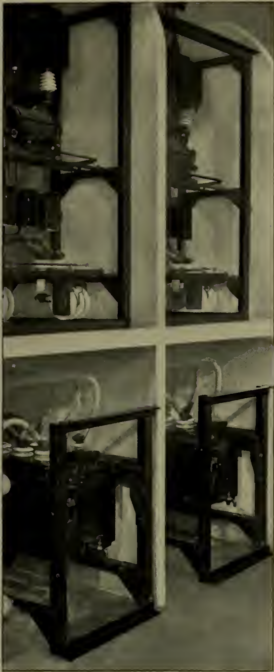
FIG. 7.—OIL SWITCHES AND TRANSFORMERS FOR SUPPLYING CURRENT TO SWITCHBOARD INSTRUMENTS IN THE PLANT AT MONTEREALE
