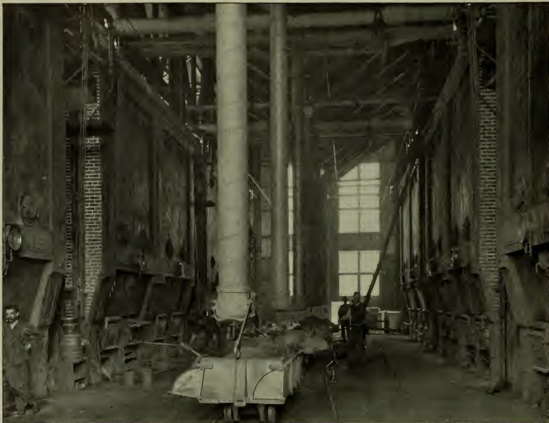
FIG. 6.—THE BOILER ROOM IN THE WESTVILLE POWER STATION. TWELVE WATER-TUBE BOILERS BUILT BY THE STIRLING CONSOLIDATED BOILER COMPANY, NEW YORK, AND PROVIDED WITH SUPERHEATERS, GENERATE STEAM AT 175 POUNDS
