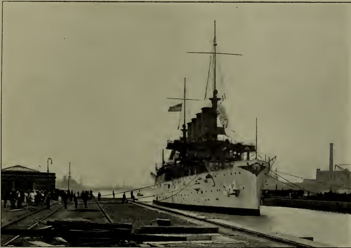
FIG. 1.—THE UNITED STATES CRUISER "MARYLAND" ENTERING THE NEW DRY DOCK IN THE BOSTON NAVY YARD. THE BUILDING IN WHICH THE PUMPING PLANT IS HOUSED IS SHOWN AT THE LEFT
