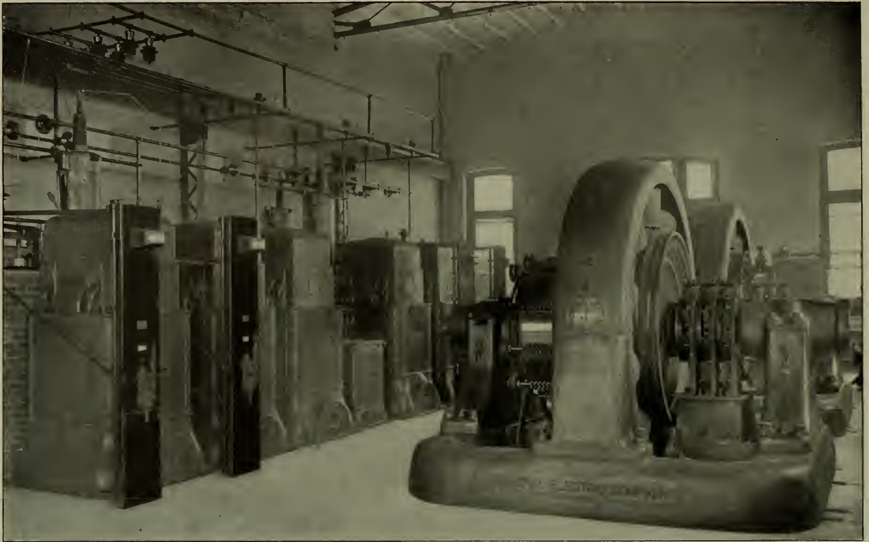
FIG. 12.—INTERIOR OF THE ATLANTIC CITY SUB-STATION. THE HIGH-TENSION, 3-PHASE CURRENT IS REDUCED IN PRESSURE AND CONVERTED TO DIRECT CURRENT AT 650 VOLTS BY SIX AIR-COOLED TRANSFORMERS AND TWO 750-KW. ROTARY CONVERTERS
