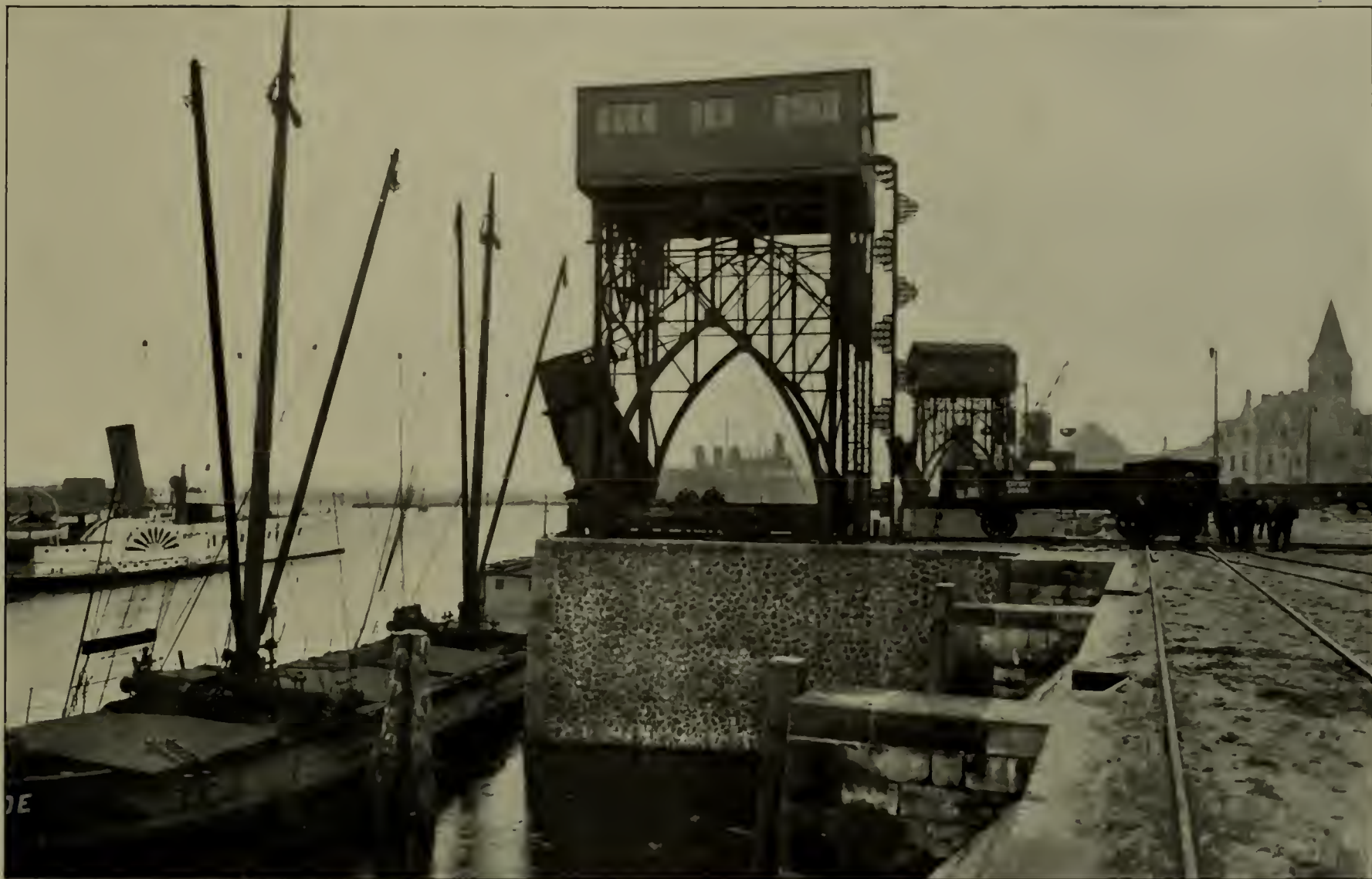
FIG. 1.—TWO ELECTRICALLY OPERATED COAL TIPS IN HAMBURG HARBOUR, GERMANY
