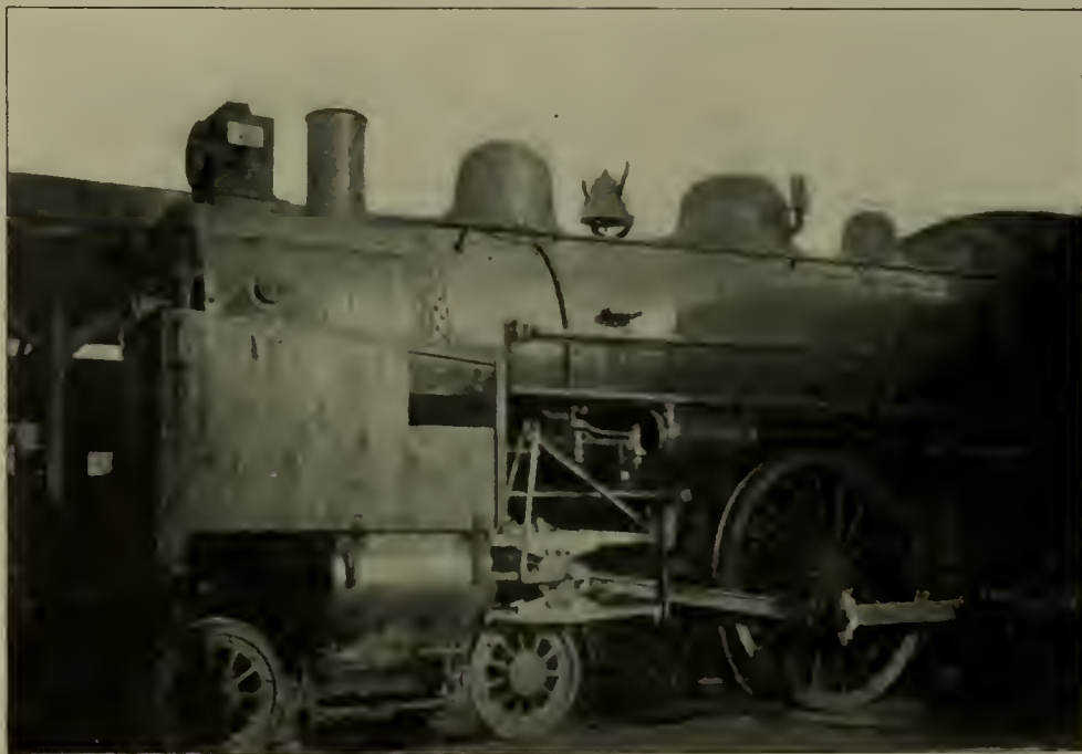
A LOCOMOTIVE FITTED WITH A WIND SHIELD FOR PROTECTION WHILE INDICATOR CARDS WERE TAKEN
