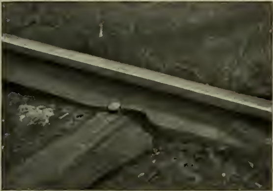
FIG. 5.—IN THIS CASE THE RAIL FLANGE WAS EATEN ENTIRELY THROUGH. THE SPIKE SHOWN IS A NEW ONE, PLACED FURTHER ALONG ON THE EDGE OF THE TIE
