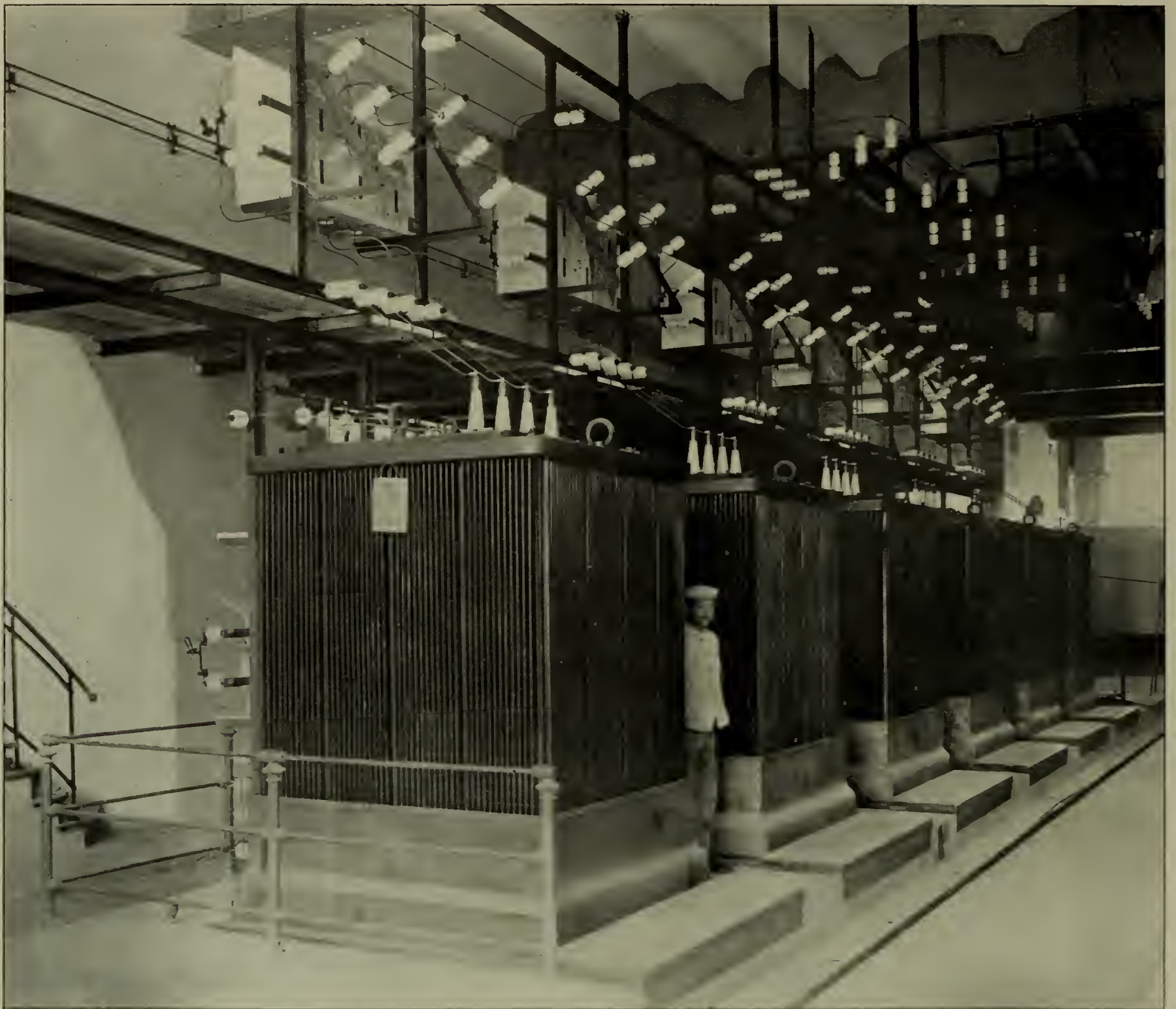
FIG. 21.—TRANSFORMERS IN THE GLOMMEN RIVER POWER PLANT. CURRENT IS GENERATED AT 5000 VOLTS AND RAISED TO 20,000 VOLTS
