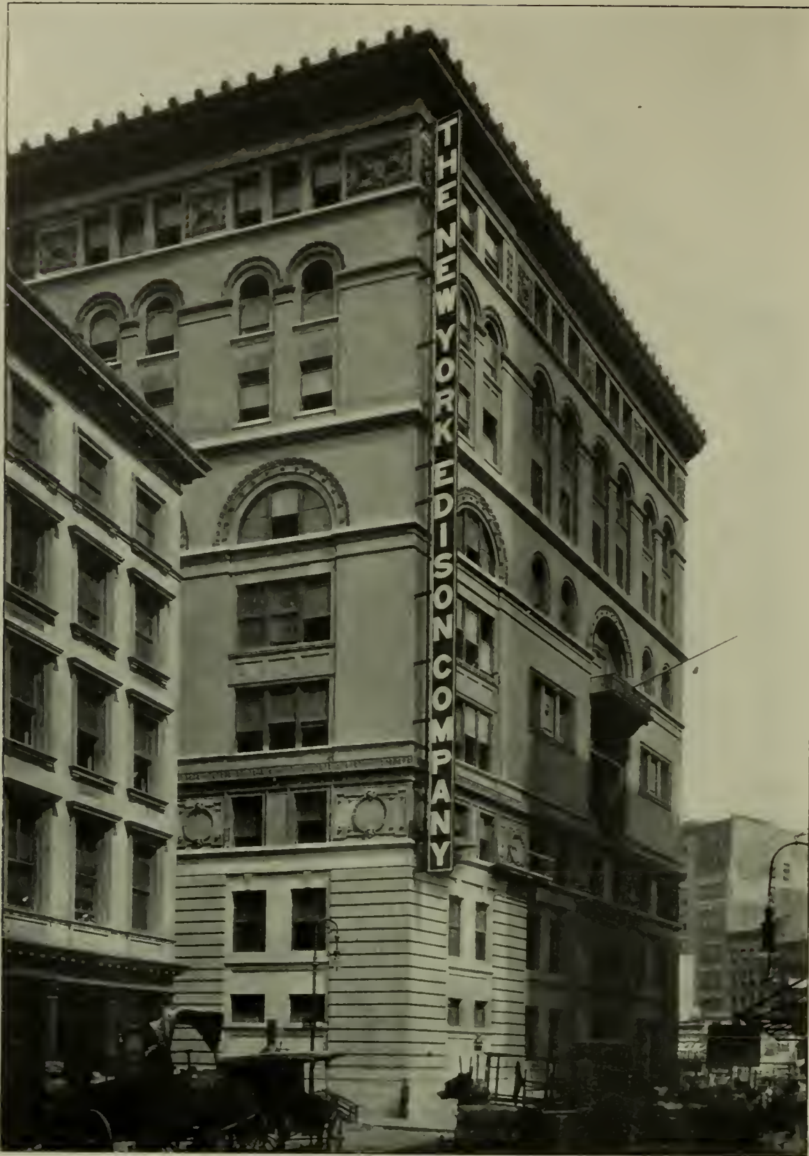
THE LARGEST VERTICAL SIGN IN THE WORLD. IT IS 100 FEET LONG, AND WAS BUILT BY THE METROPOLITAN ENGINEERING COMPANY, OF BROOKLYN, FOR THE DUANE STREET STATION OF THE NEW YORK EDISON COMPANY
