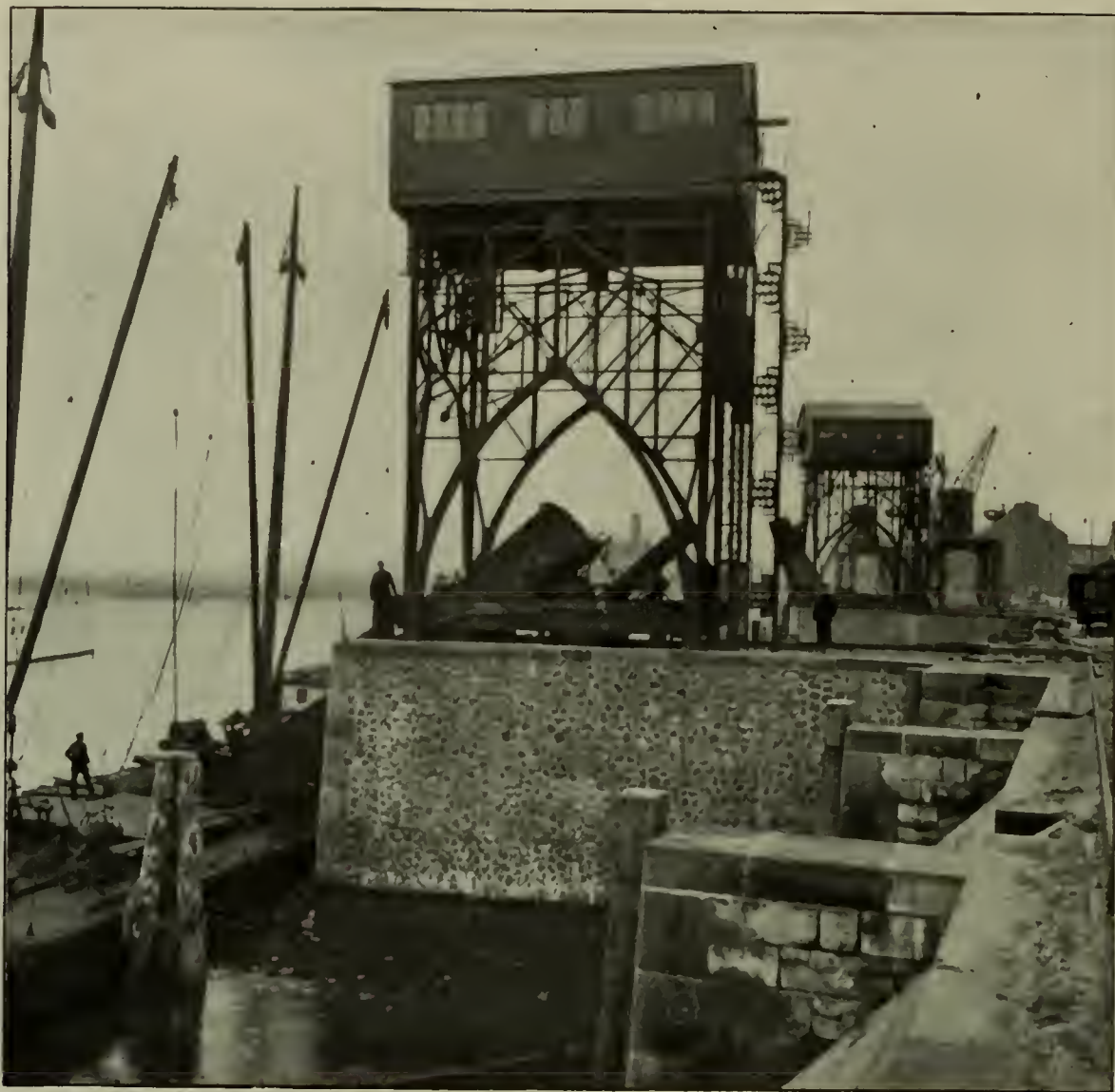
FIG. 2.—FOR LOW-WATER LEVELS, THE TIP IS OPERATED AUTOMATICALLY BY THE WEIGHT OF THE LOADED CAR
