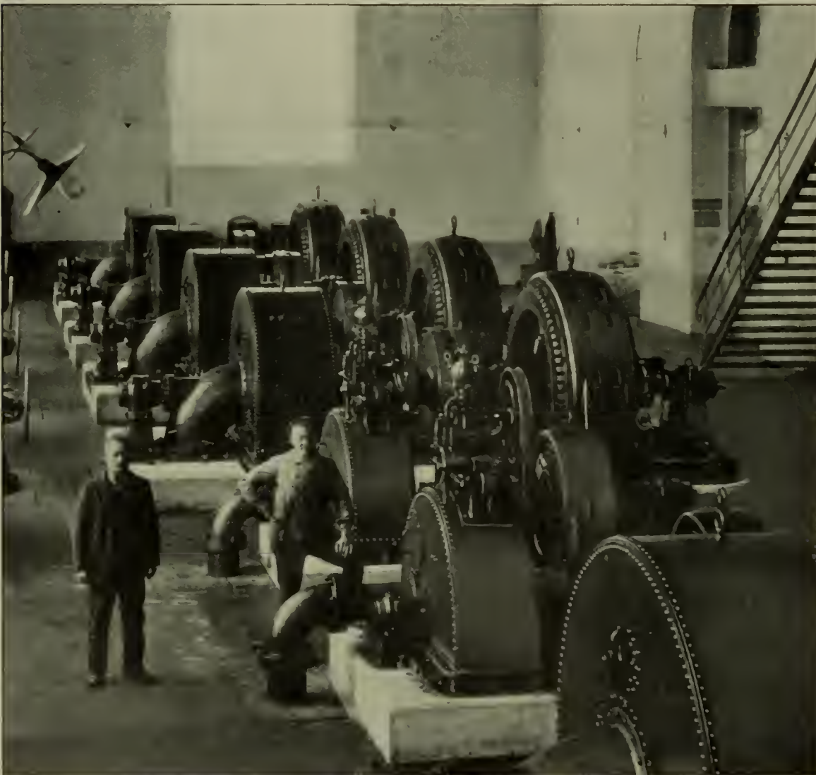
FIG. 11.—INTERIOR OF THE TUSCIANO RIVER PLANT IN ITALY, SHOWING FIVE 1400-H. P. UNITS AND TWO 150- H. P. EXCITER UNITS
