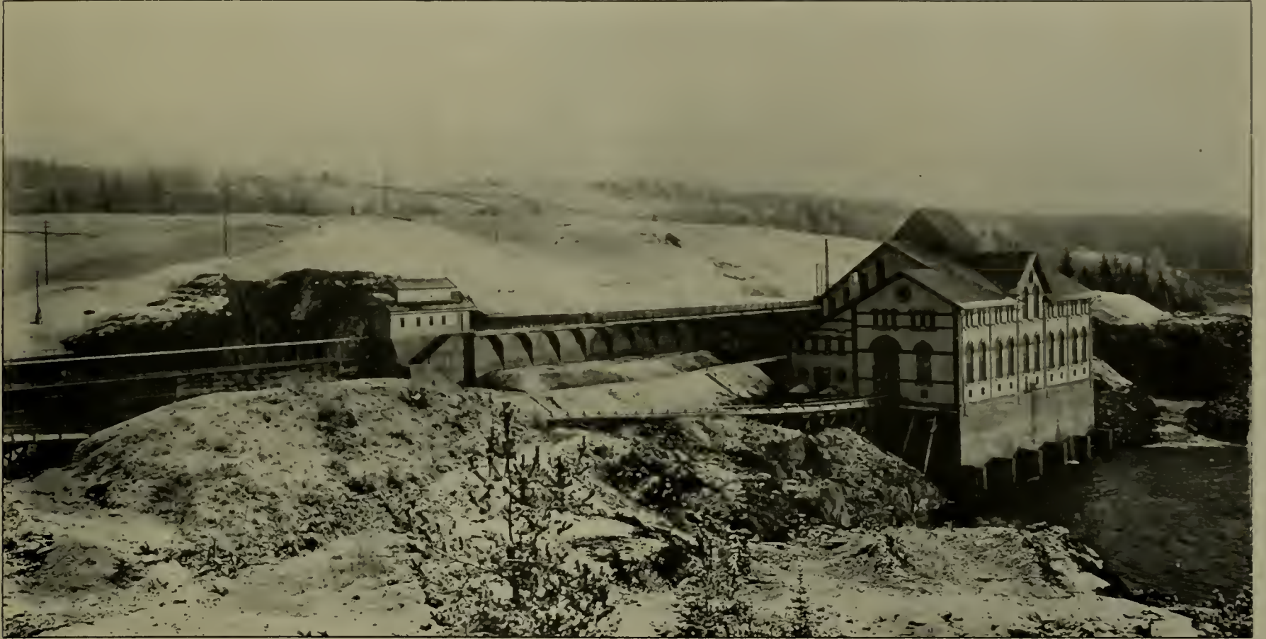
FIG. 19.—A HYDRO-ELECTRIC PLANT ON THE GLOMMEN RIVER, IN SOUTHEASTERN NORWAY
