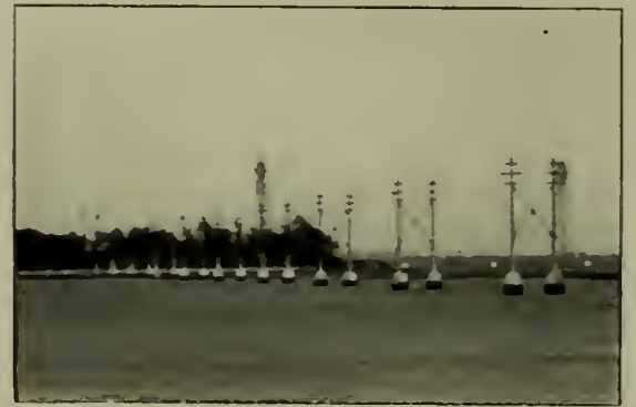
FIG. 12.—PART OF THE TRANSMISSION LINE FROM MONTEREALE TO VENICE. FOUR THREE-PHASE CIRCUITS ARE MOUNTED ON DOUBLE POLES
