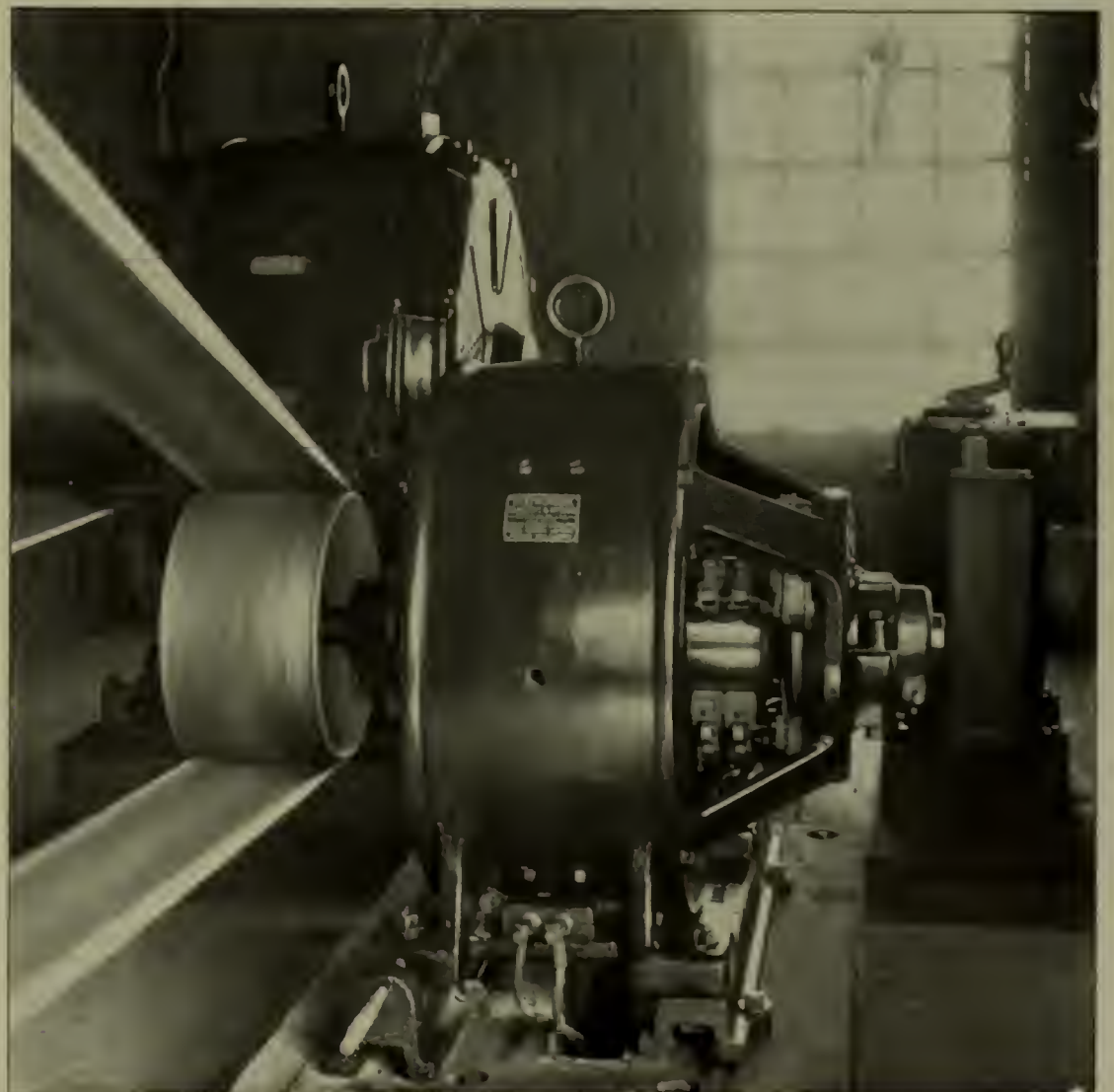
IN THE BACKGROUND IS A 100-H. P INDUCTION MOTOR OPERATING KILNS. IN THE FOREGROUND IS A 22½-KW. EXCITER
