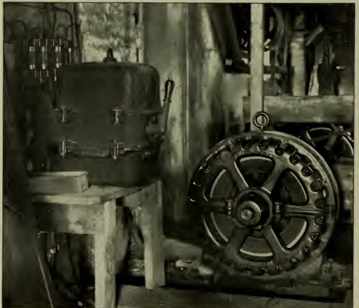
ONE OF TWO 50-H. P. INDUCTION MOTORS INSTALLED BY THE WESTINGHOUSE ELECTRIC & MANUFACTURING COMPANY, OF PITTSBURG, IN THE PLANT OF THE SPRINGFIELD, OHIO, METALLIC CASSET COMPANY
