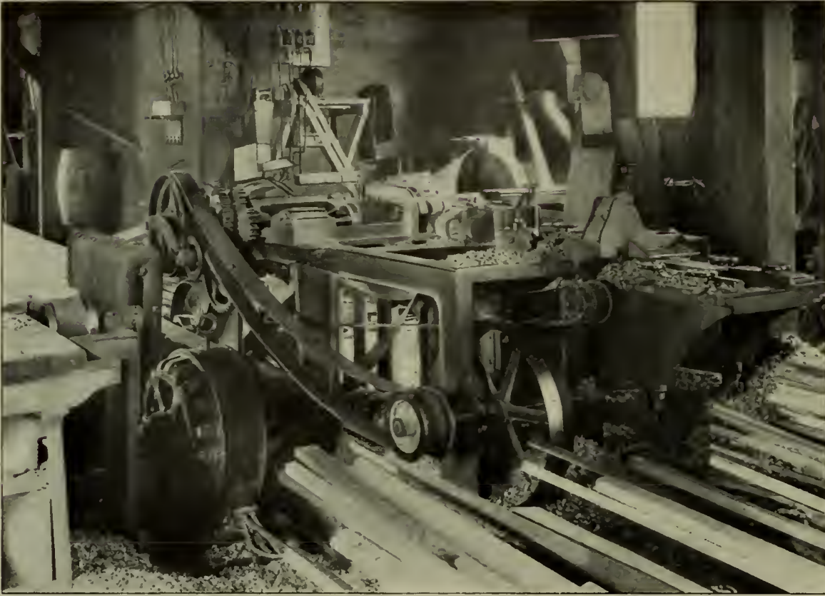
A MOULDING MACHINE DRIVEN BY A 15-H. P. WESTINGHOUSE INDUCTION MOTOR IN THE EGGERS & GRAHAM LUMBER MILL
