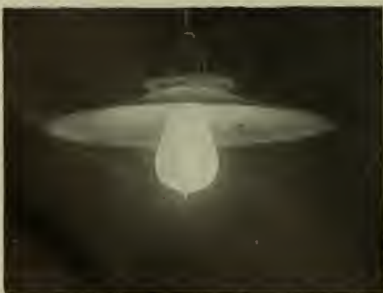
A WHITE PORCELAIN SHADE. POOR FOR READING
