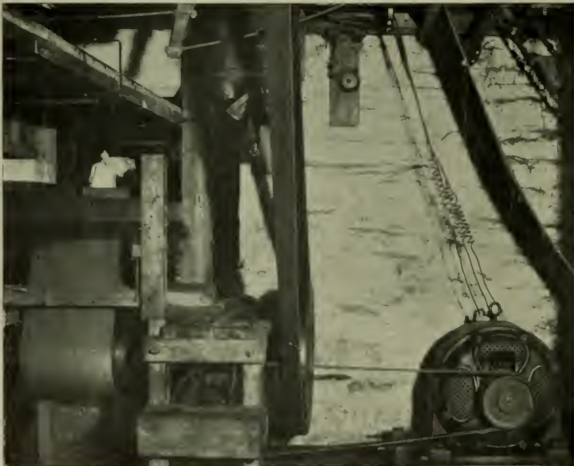
A MOTOR DRIVING A PARCELS CONVEYOR, WHICH TAKES PARCELS FROM SALESROOMS TO ASSORTING SECTION PRIOR TO SHIPMENT. THIS MOTOR ALSO DRIVES A BARREL HOIST
