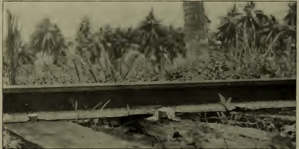
FIG. 3.—ANOTHER SPIKE HEAVILY INCRUSTED BY ELECTROLYTIC ACTION
