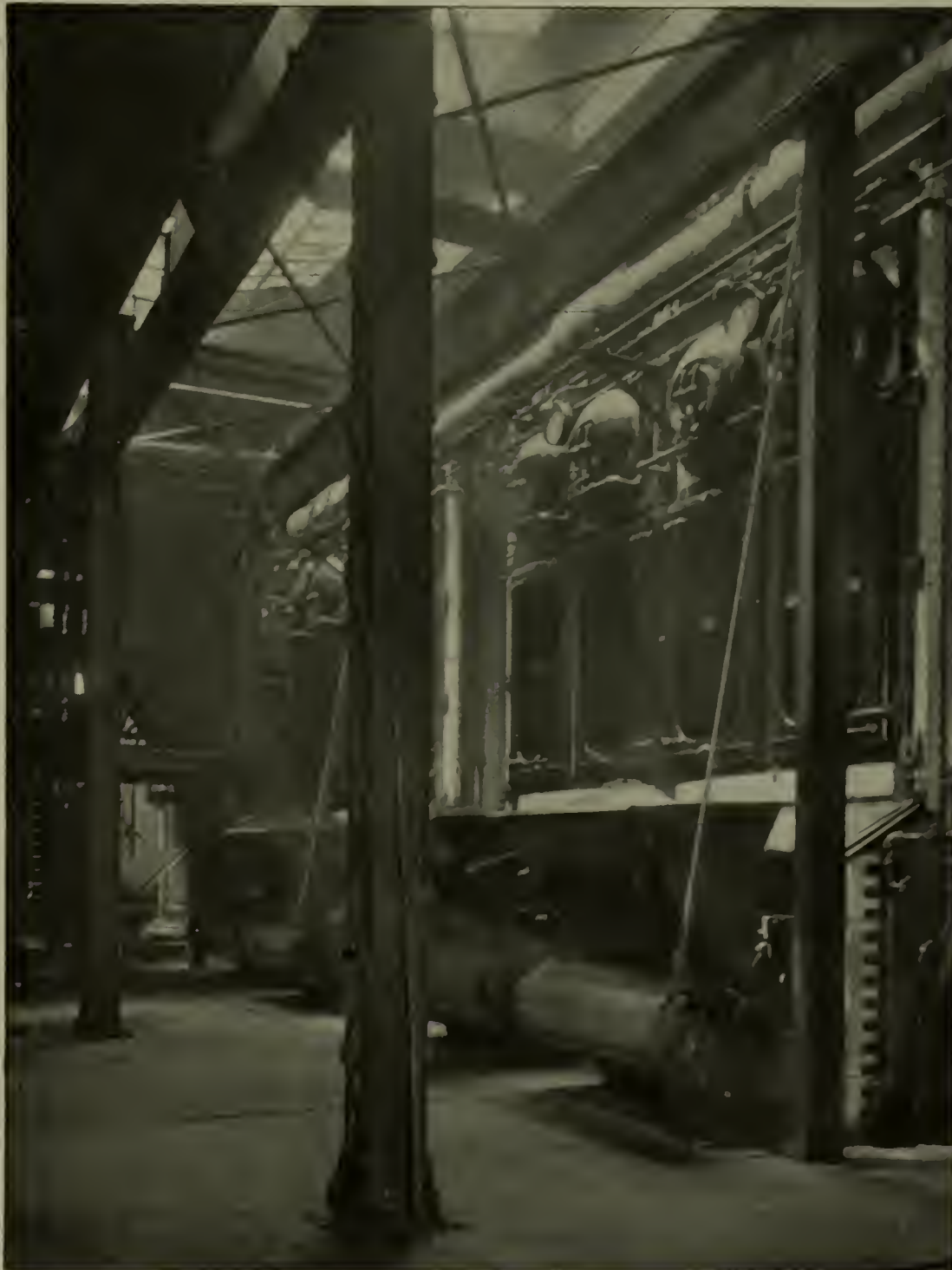
THE BABCOCK & WILCOX BOILERS IN THE CENTRAL POWER PLANT OF THE ESTATE OF HENRY W. OLIVER, PITTSBURG, PA., ARE PROVIDED WITH CHAIN GRATES MADE BY THE GREEN ENGINEERING COMPANY, CHICAGO
