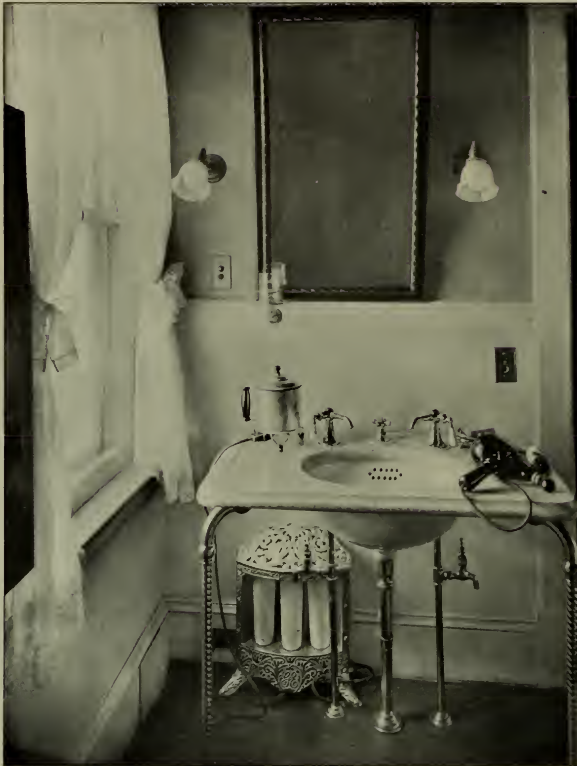
A PART OF THE BATH-ROOM, WITH RADIATOR, MASSAGE VIBRATOR AND WATER-HEATER FOR SHAVING
