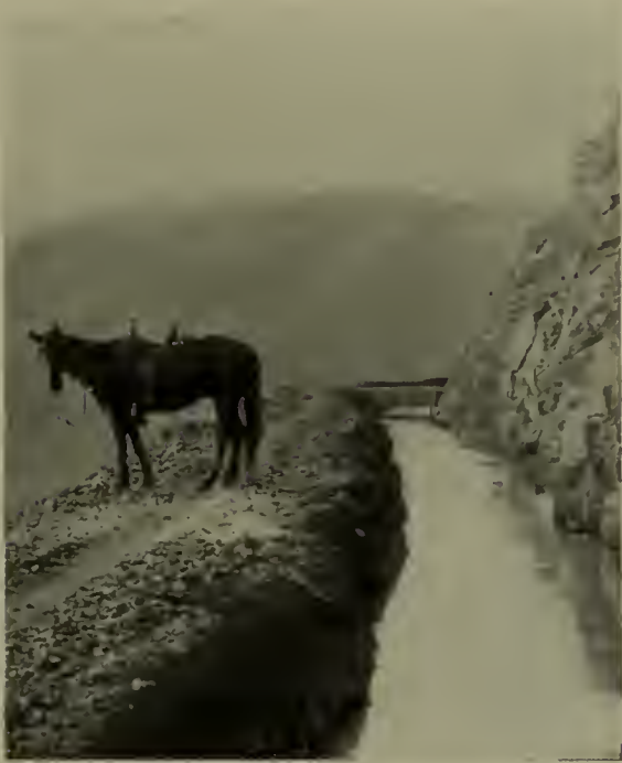
THE DITCH THROUGH WHICH THE WATER IS DIVERTED TO THE PLANT OF THE NORTH MOUNTAIN POWER COMPANY
