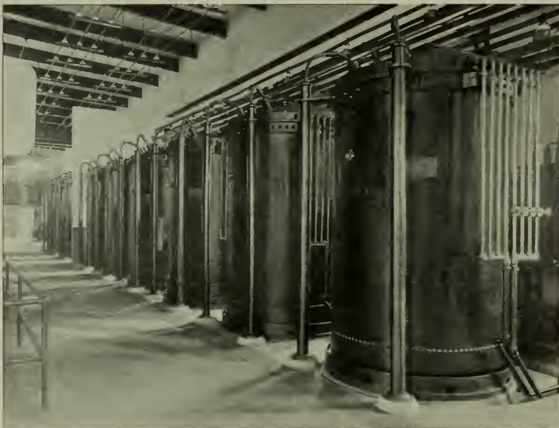
THREE BANKS OF 2250-KW. TRANSFORMERS IN THE TERMINAL HOUSE
