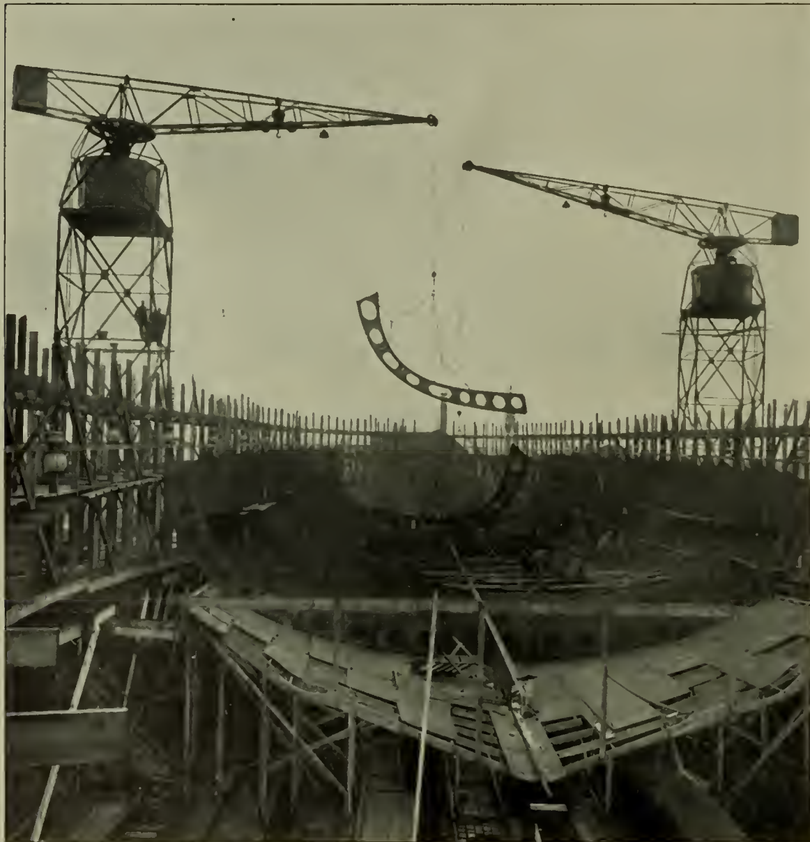
FIG. 17.—TWO ROTARY TOWER CRANES AT THE IMPERIAL SHIP WORKS AT WILHELMHAVEN
