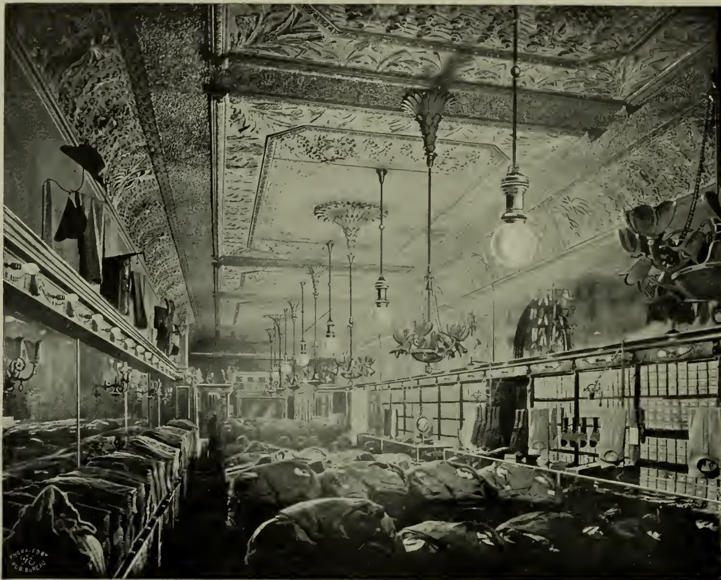
FIG. 5.—A CLOTHING STORE LIGHTED BY GENERAL ELECTRIC SUSPENDED ARC LAMPS AND INCANDESCENT LAMPS AT THE SIDES
