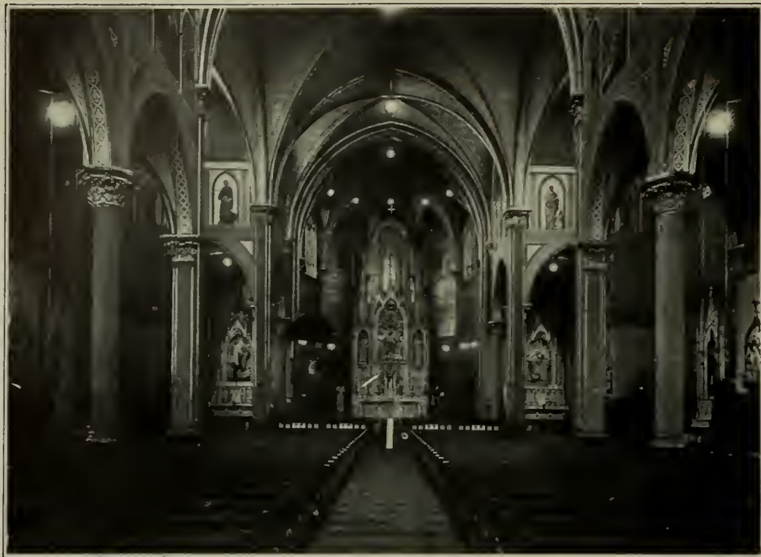
FIG. 8.—NERNST LAMPS IN THE INTERIOR OF HOLY TRINITY CATHOLIC CHURCH, PITTSBURG
