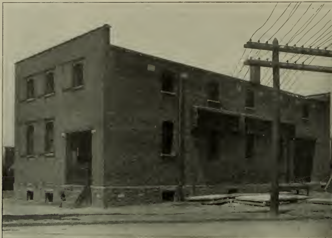
STATION NO. 4, SHOWING THE 2200-VOLT LINES LEAVING THE BUILDING
