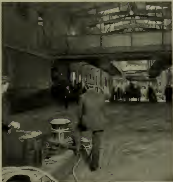
AN ELECTRIC WINDLASS AT THE DESBROSSES STREET FERRY, IN NEW YORK, OF THE PENNSYLVANIA RAILROAD
