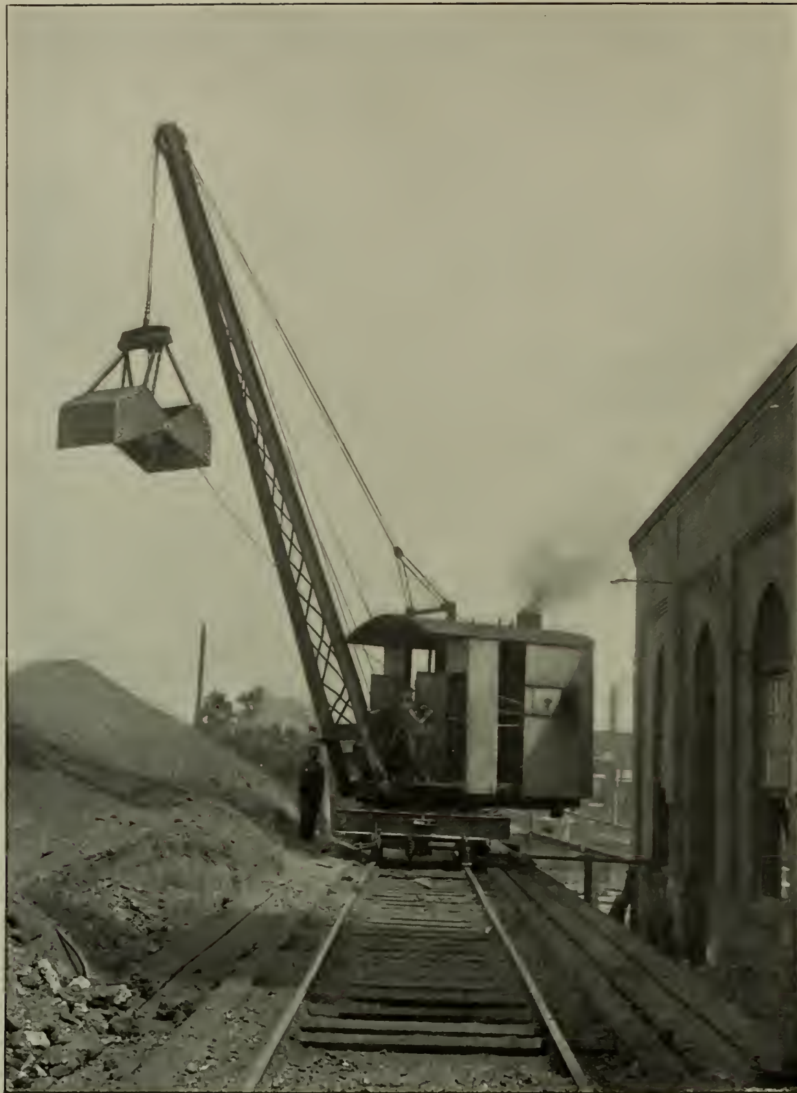
A LOCOMOTIVE CRANE BUILT BY THE BROWNING ENGINEERING COMPANY, CLEVELAND, OHIO, FOR HANDLING COAL AND ASHES
