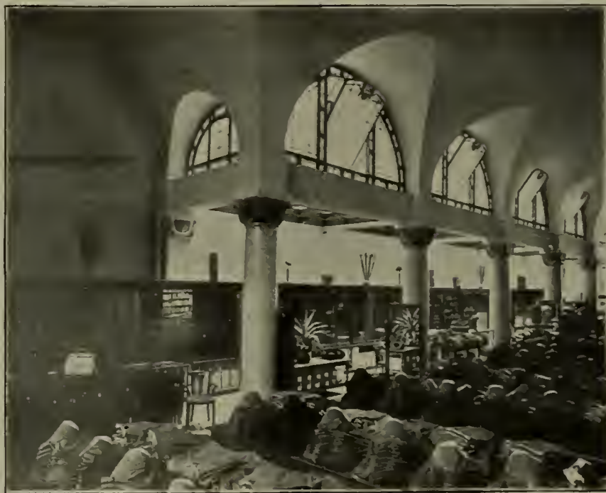
FIG. 3.—THE MAIN FLOOR OF THE REED BUILDING ON THE EAST SIDE. THE SIDE SKYLIGHTS ADMIT THE LIGHT FOR THE ILLUMINATION OF THE CENTRAL PART OF THE FLOOR
