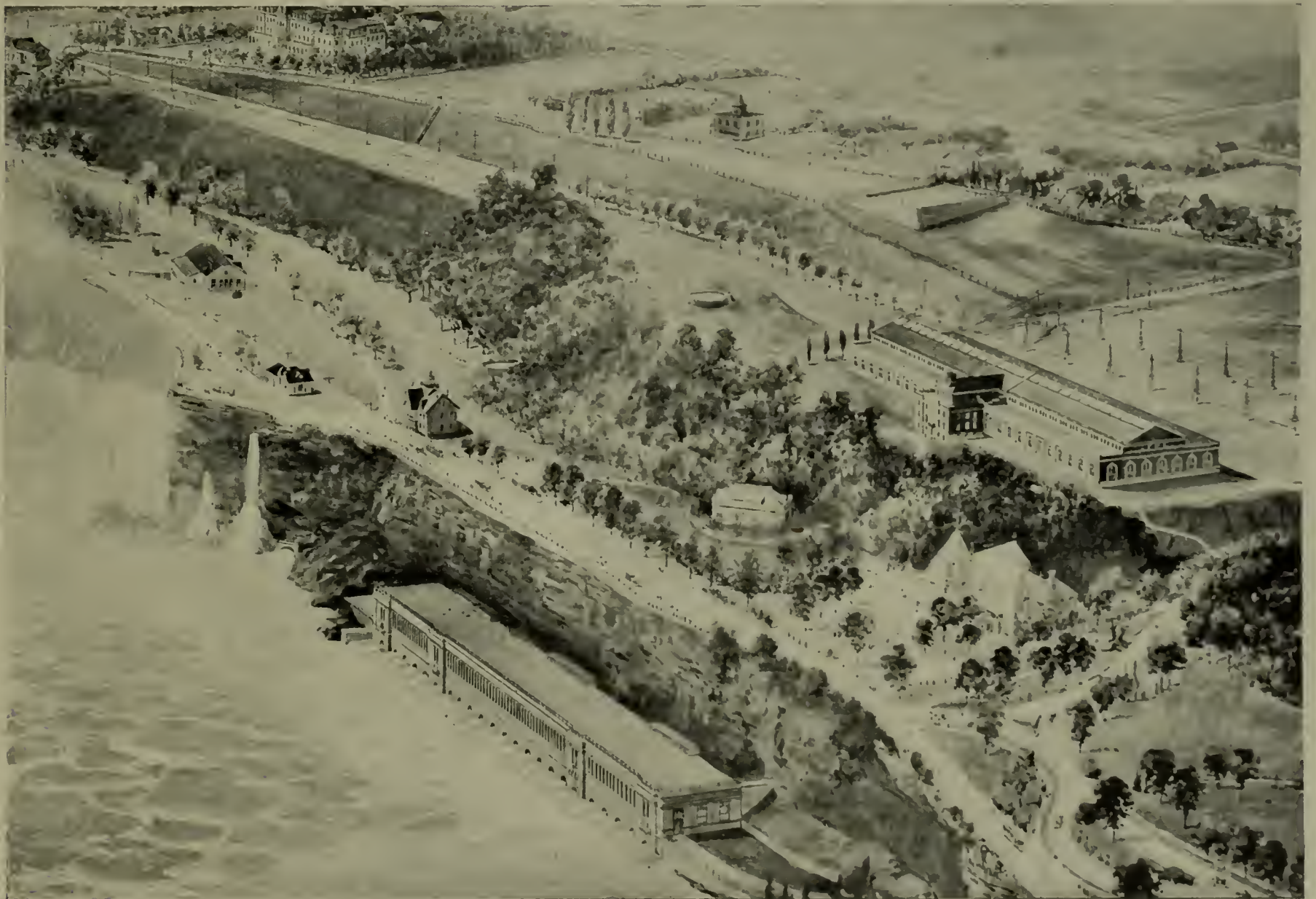
BIRD'S EYE VIEW, SHOWING GENERATING AND DISTRIBUTING STATIONS COMPLETE FOR 200,000 HORSE POWER
