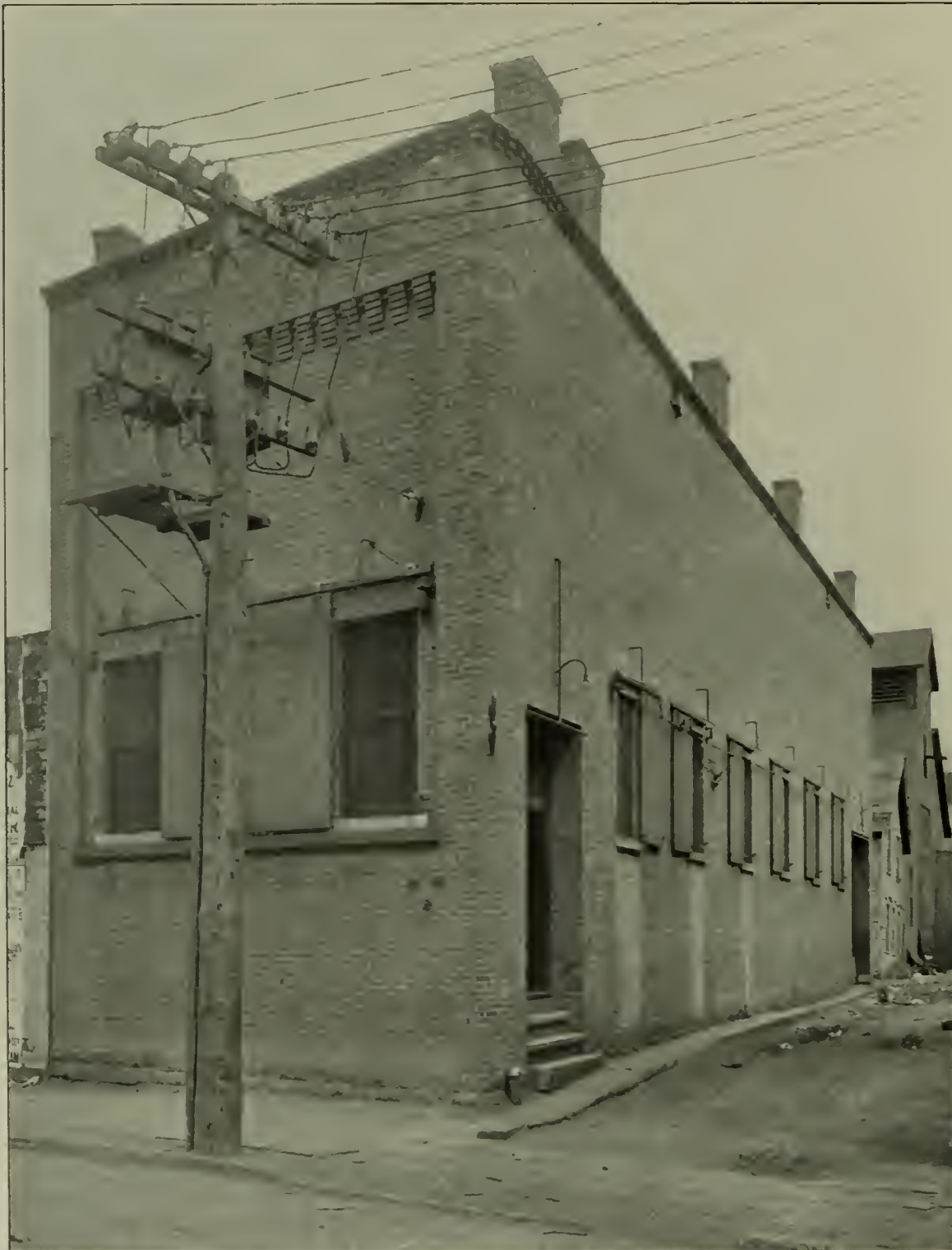
STATION NO. 2, SHOWING ALSO THE 2200-VOLT FEEDERS LEAVING THE TERMINAL POLE
