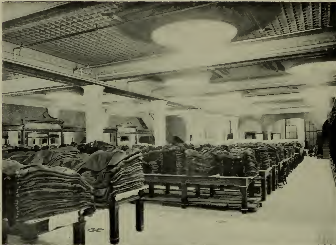
FIG. 10.—A CLOTHING STORE ILLUMINATED WITH LIGHT-BALANCING, SELECTIVE-DIFFUSER CEILINGS
