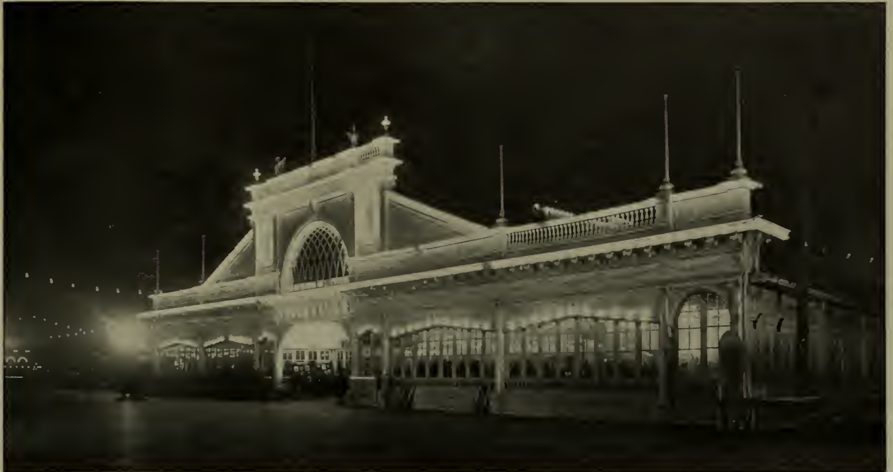
NIGHT VIEW OF THE ENTRANCE TO YOUNG'S PIER, ATLANTIC CITY. IT IS ON THIS PIER THAT THE MEMBERS OF THE NATIONAL ELECTRIC LIGHT ASSOCIATION ARE TO MEET IN CONVENTION
