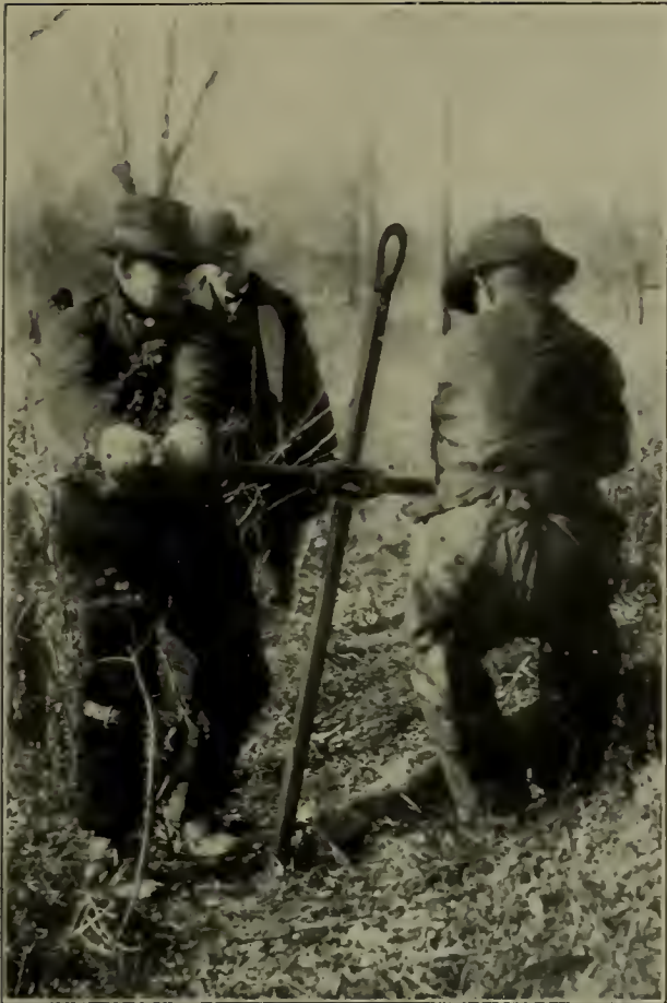
METHOD OF PLACING THE NEW STOMBAUGH GUY ANCHOR MADE BY W. N. MATTHEWS & BRO., ST. LOUIS
