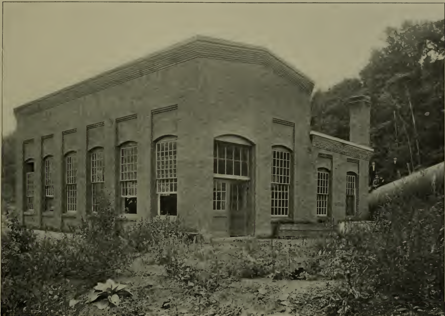
A CLOSER VIEW OF THE POWER HOUSE. CURRENT IS CARRIED TO THE MILLS THROUGH AN UNDERGROUND LINE, CONSISTING OF CABLES RUN IN TILE DUCT LAID IN CONCRETE
