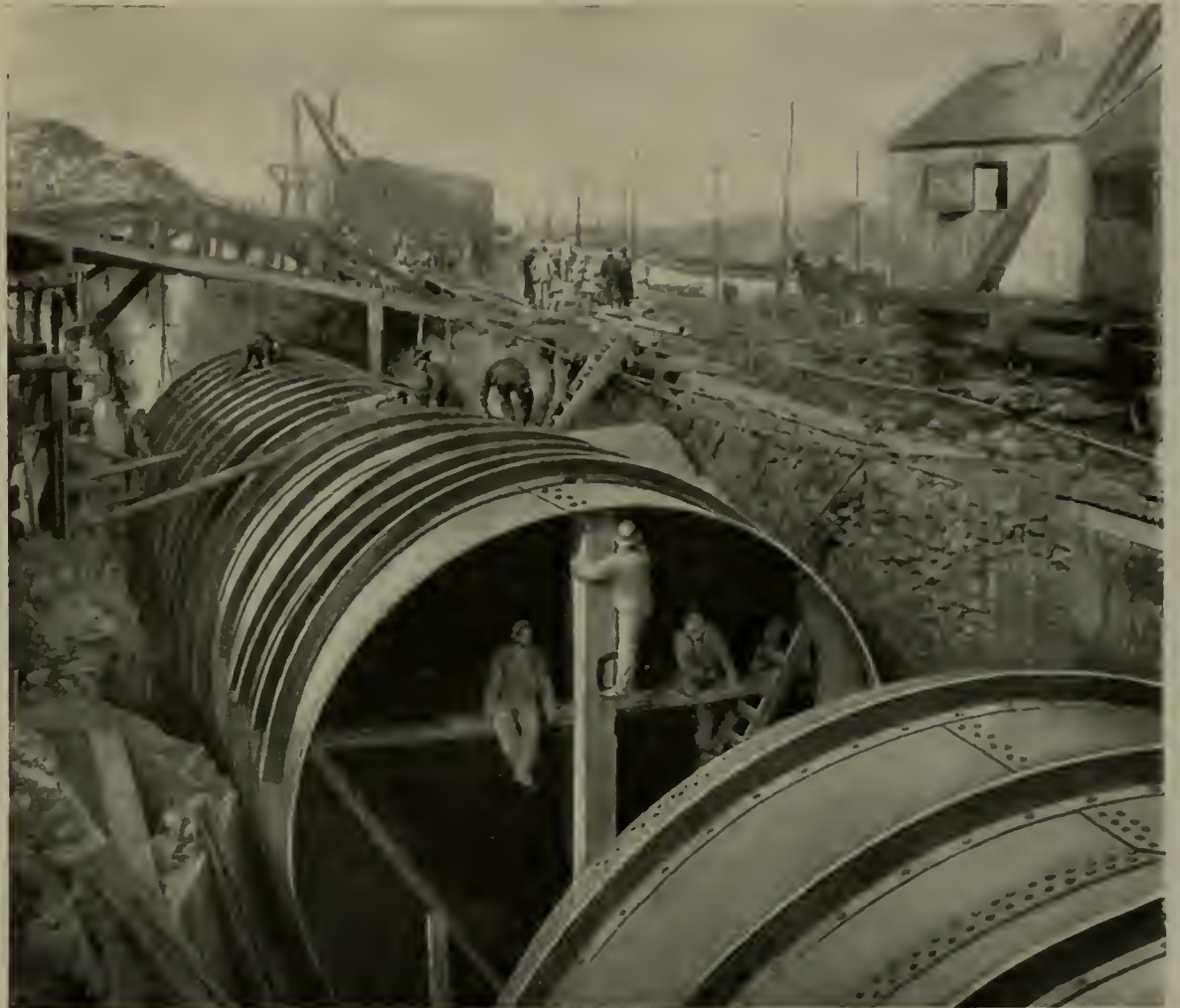
MAIN CONDUIT DURING CONSTRUCTION
