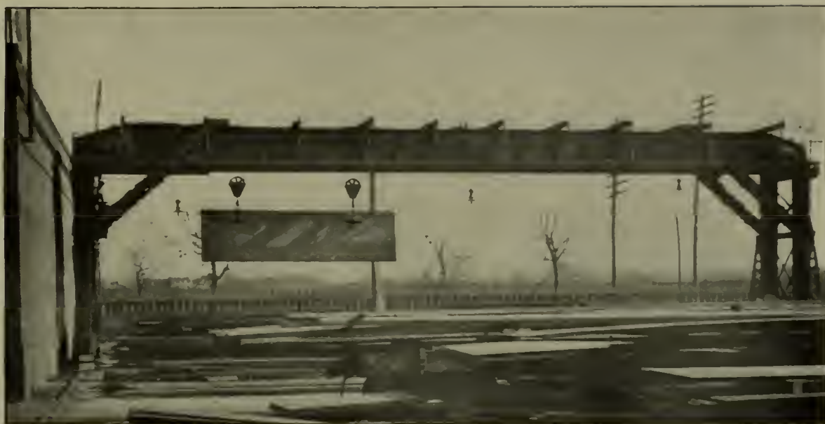
AN 88-FOOT SPAN GANTRY CRANE, WITH LIFTING MAGNETS FOR HANDLING PLATES
