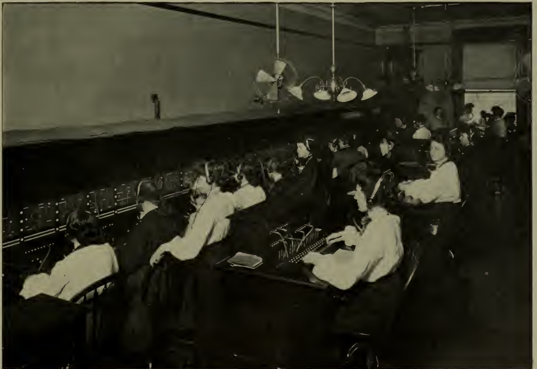
THE OPERATING ROOM MAINTAINED BY THE NEW YORK TELEPHONE COMPANY FOR THE INSTRUCTION OF STUDENT OPERATORS
