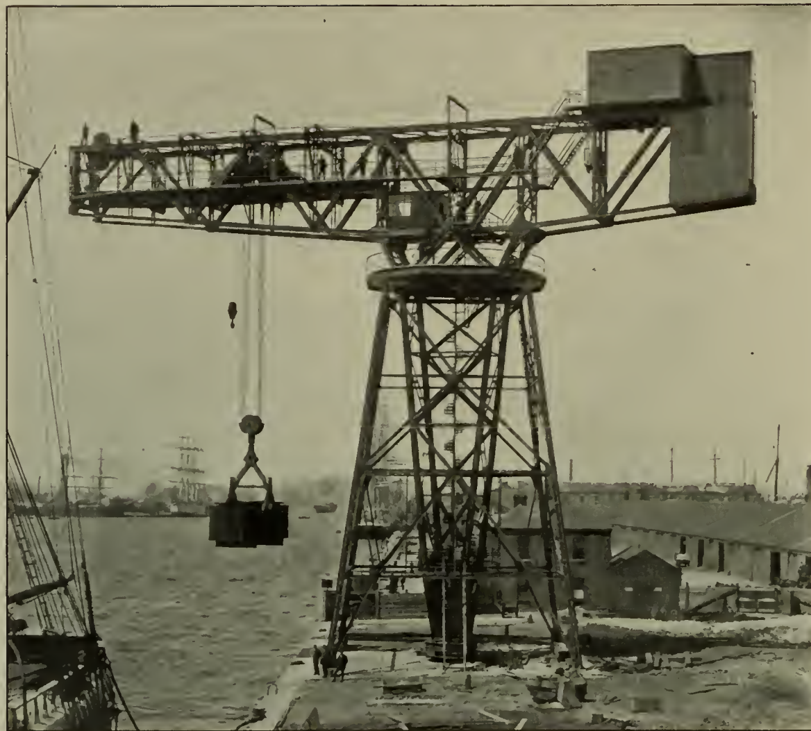
FIG. 9.—A 100-TON ROTARY-TOWER CRANE AT DUBLIN, IRELAND
