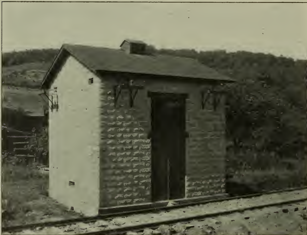
TRANSFORMER STATIONS ARE BUILT OF CONCRETE BLOCKS, AND CONTAIN TWO 150-KW., 22,000-3300-VOLT TRANSFORMERS, OF THE OIL-IMMERSED, SELF-COOLING TYPE
