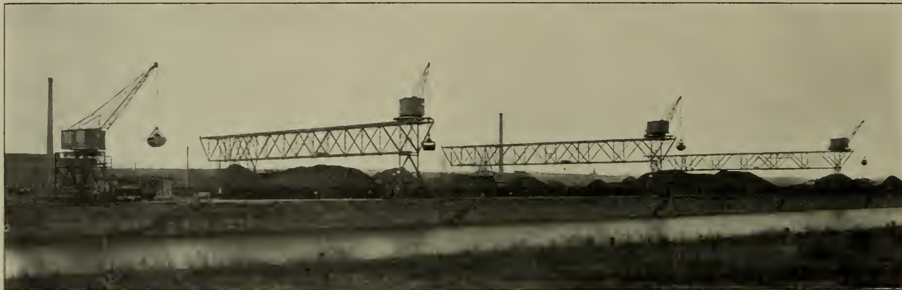
FIG. 13.—AT THE HARBOUR OF OFFENBACH, THREE TRANSPORTABLE LOADING BRIDGES AND A TRANSPORTABLE GANTRY CRANE ARE USED FOR COAL HANDLING
