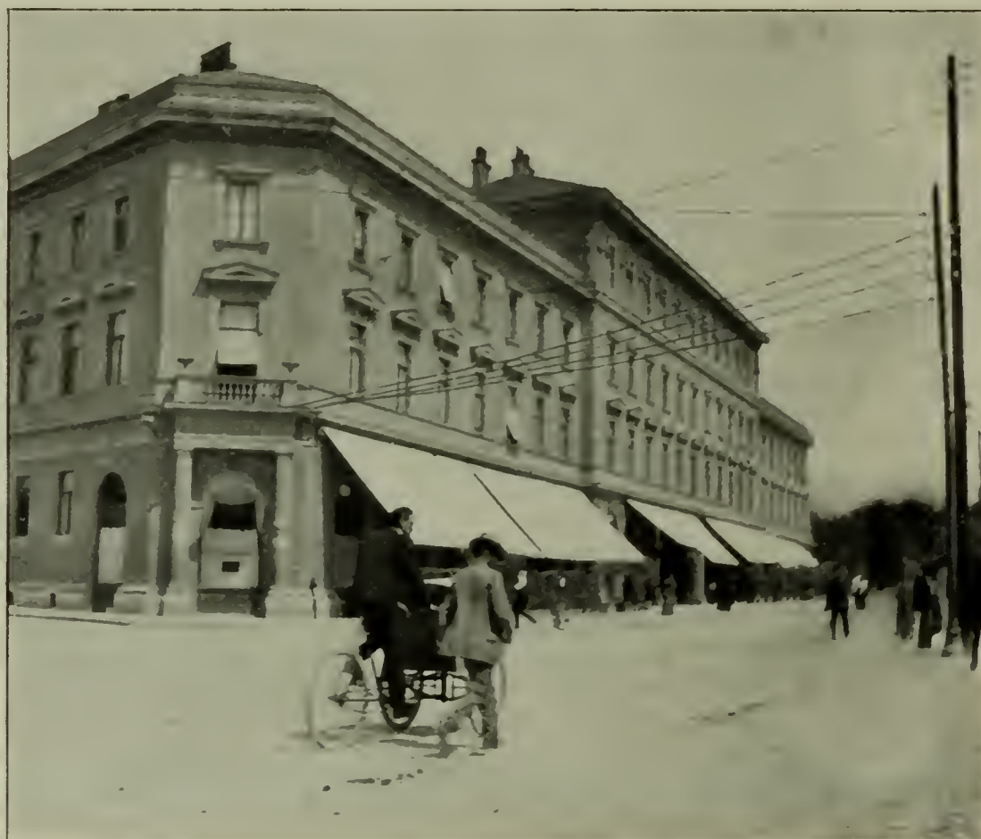
THE TELEPHONE WIRES IN SARAJEVO, THE CAPITAL OF BOSNIA, ARE ONE OF MANY INDICATIONS OF THE USE OF ELECTRICITY
