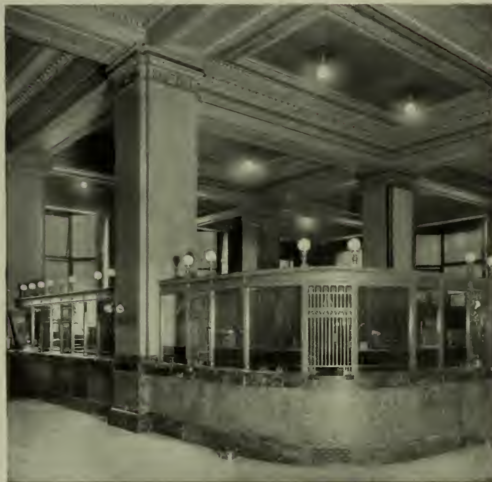
FIG. 6.—NERNST LAMPS ARE ALSO USED IN THE UNION SAVINGS BANK, PITTSBURG
