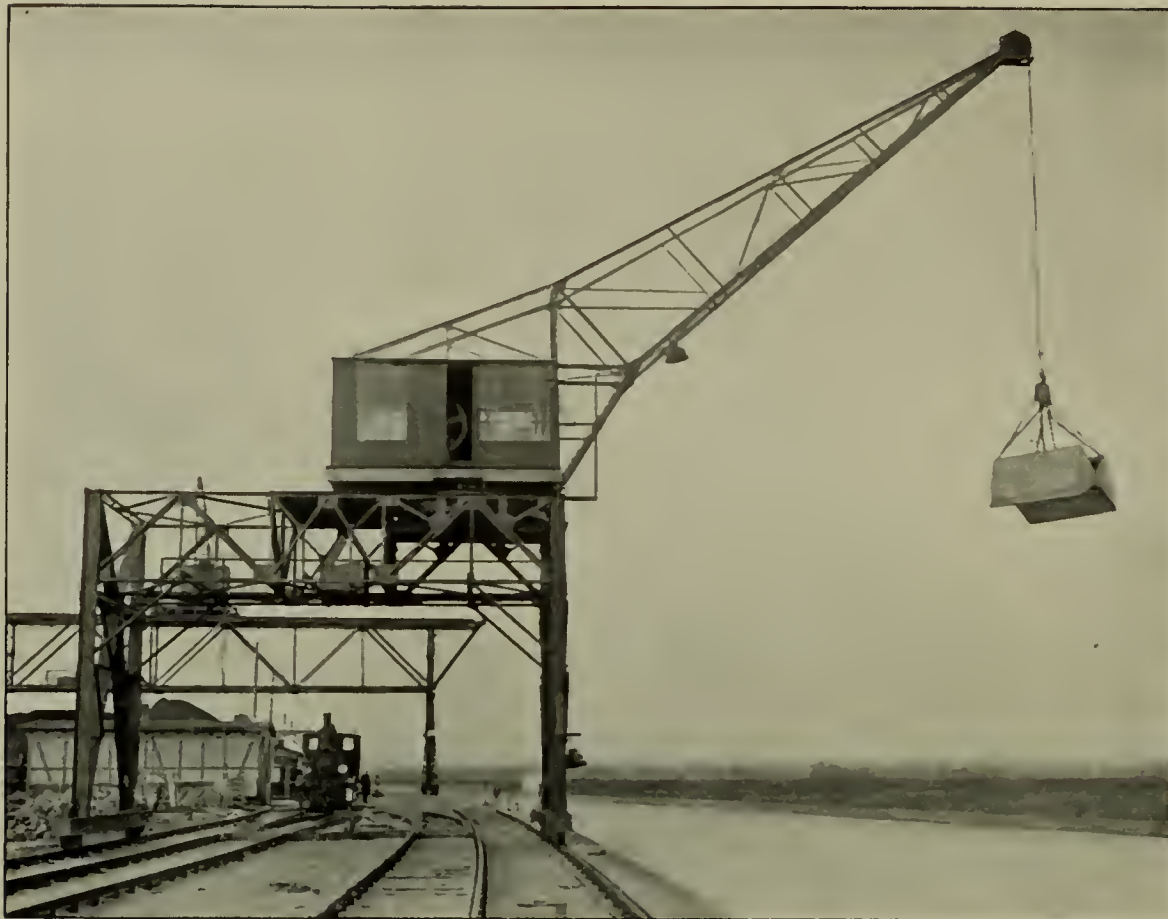
FIG. 16.—A TRANSPORTABLE GANTRY CRANE USED FOR HANDLING COAL AT OFFENBACH
