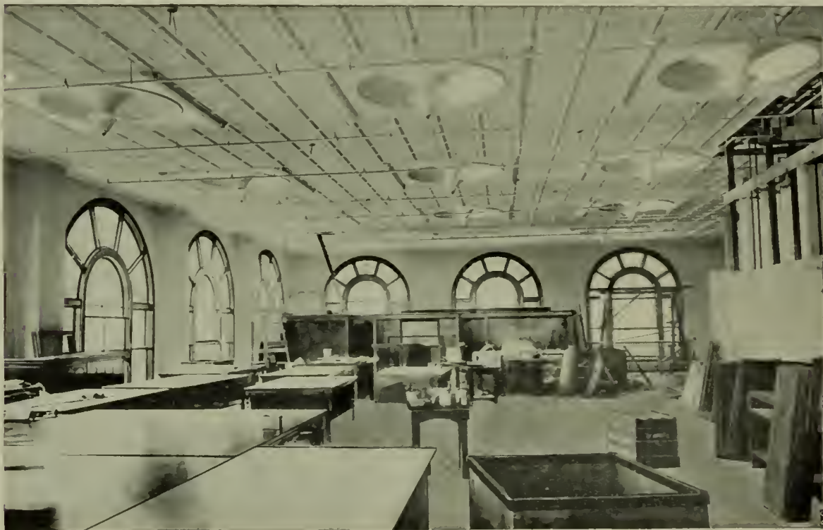
FIG. 11.—RECESSED TYPE OF LIGHT-BALANCING, SELECTIVE-DIFFUSER CEILING IN A CLOTHING STORE
