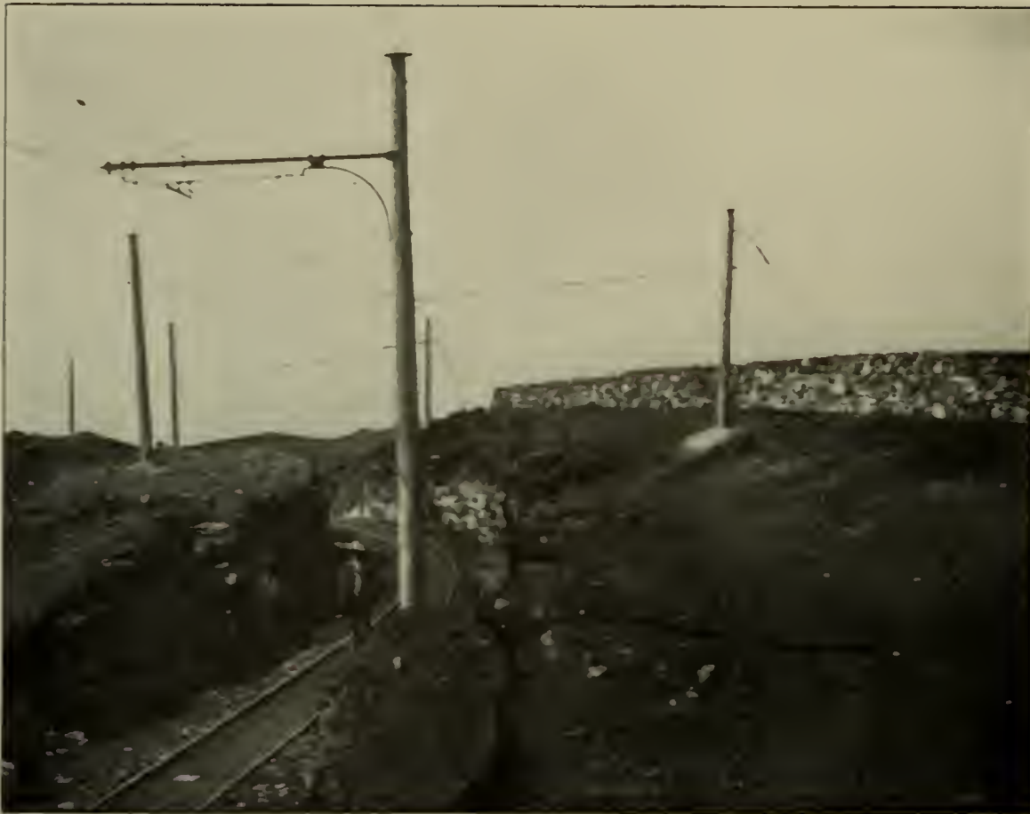
A PART OF THE ELECTRIC RAILWAY ON VESUVIUS. AT THE RIGHT IS SHOWN A WALL BUILT TO PROTECT THE LINE FROM MOLTEN LAVA
