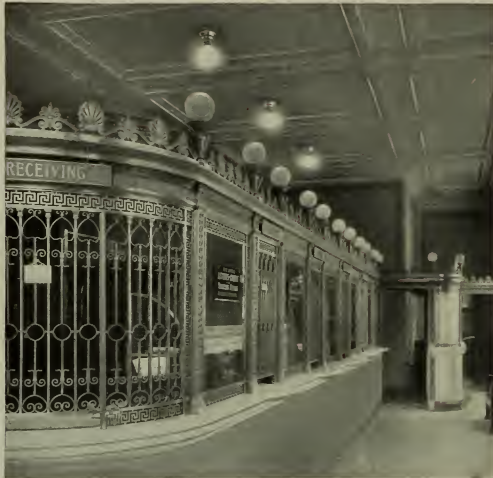
FIG. 5.—A PART OF THE GERMANIA SAVINGS BANK, PITTSBURG, LIGHTED BY NERNST LAMPS
