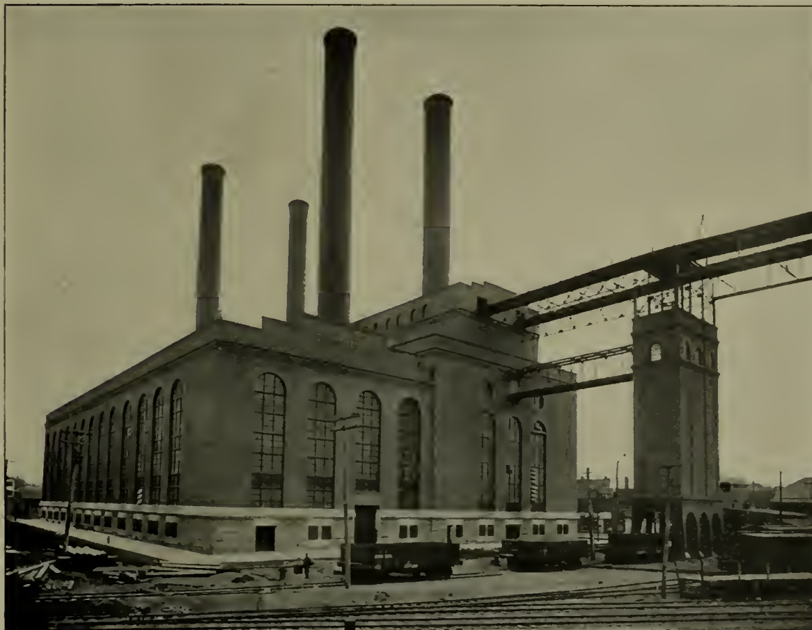
THE LONG ISLAND CITY POWER STATION OF THE PENNSYLVANIA RAILROAD. THE ASH TOWER AND A PART OF THE CABLE RAILWAY STRUCTURE ARE ALSO SHOWN
