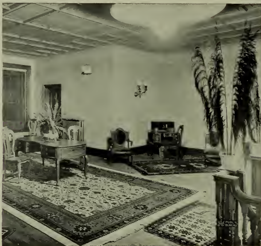
FIG. 8.—THE RECEPTION ROOM OF A MILLINERY STORE ILLUMINATED BY LIGHT-BALANCING, SELECTIVE-DIFFUSER CEILINGS. THE FURNISHINGS OF THE ROOM APPEAR TO AS GOOD ADVANTAGE AS THOUGH ILLUMINATED BY BROAD DAYLIGHT
