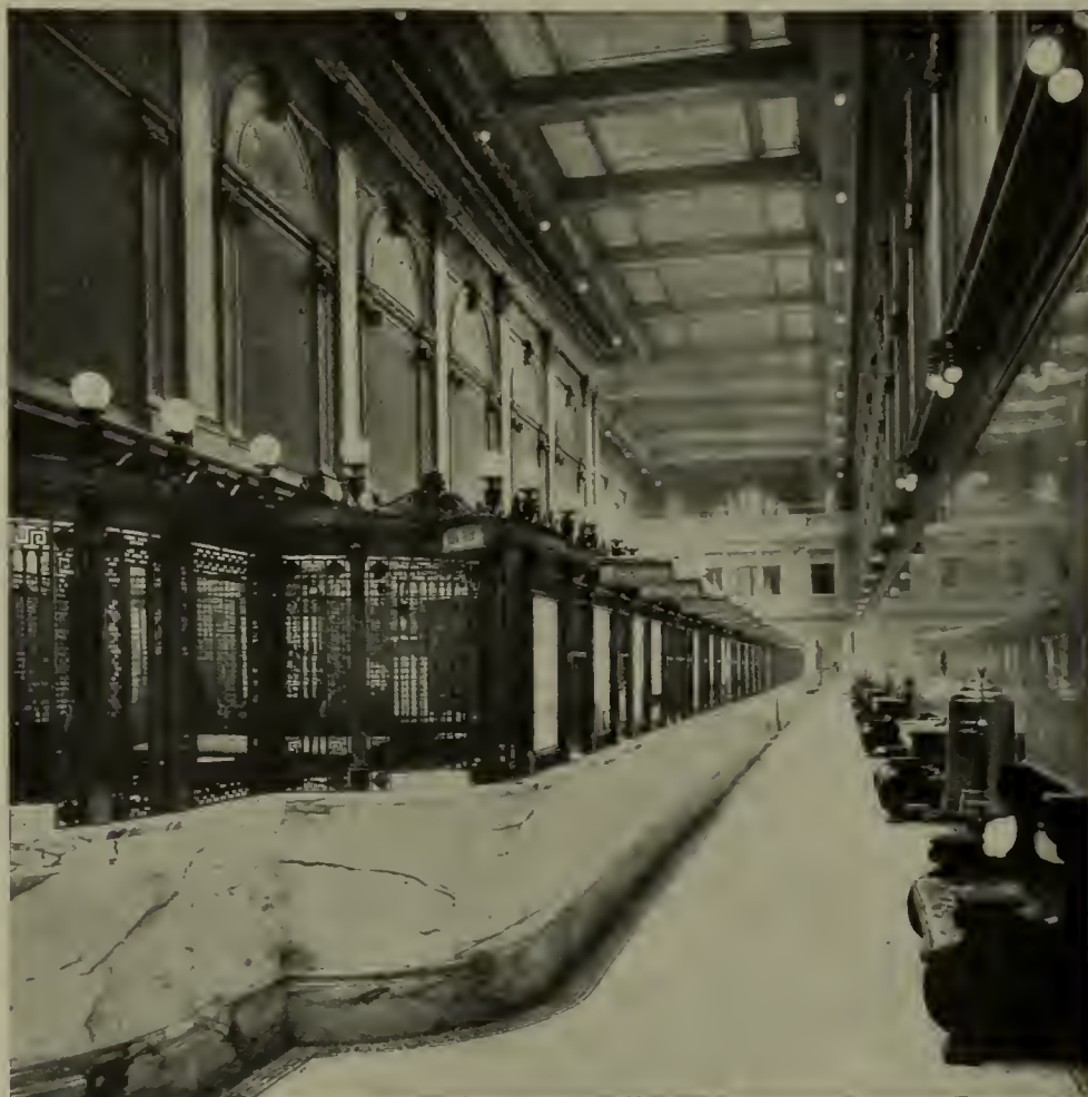
FIG. 7.—ANOTHER EXAMPLE OF BANK ILLUMINATION BY NERNST LAMPS. THE COLONIAL TRUST COMPANY, PITTSBURG
