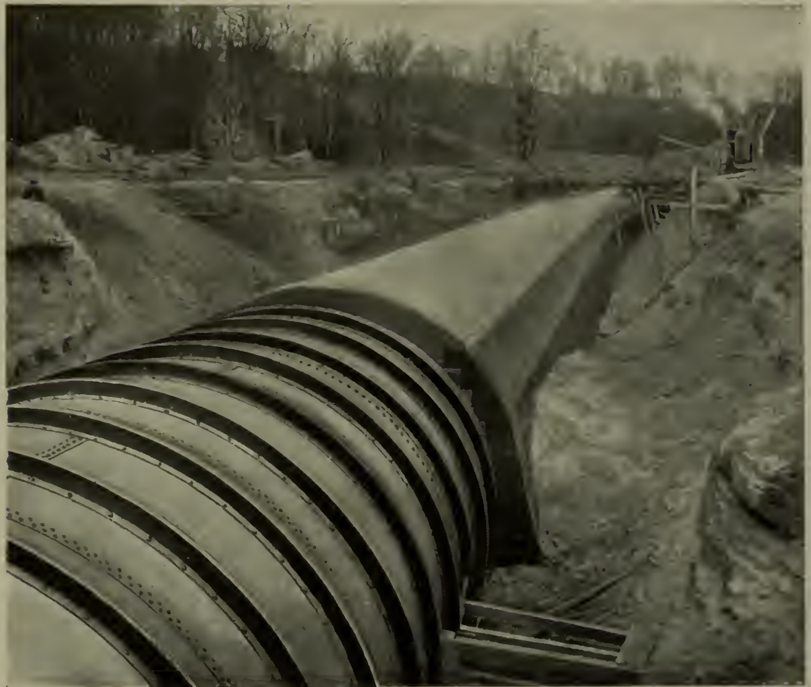
EIGHTEEN-FOOT DIAMETER CONDUIT, SHOWING CONCRETE ENVELOPE
