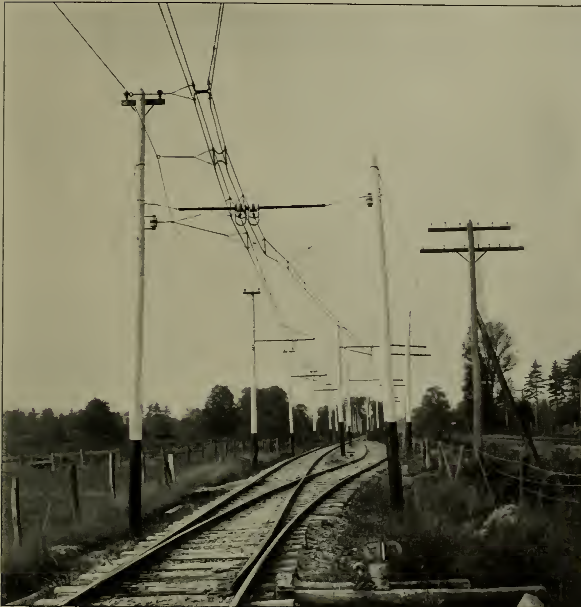
THE CATENARY OVERHEAD CONSTRUCTION AT A TURN-OUT
