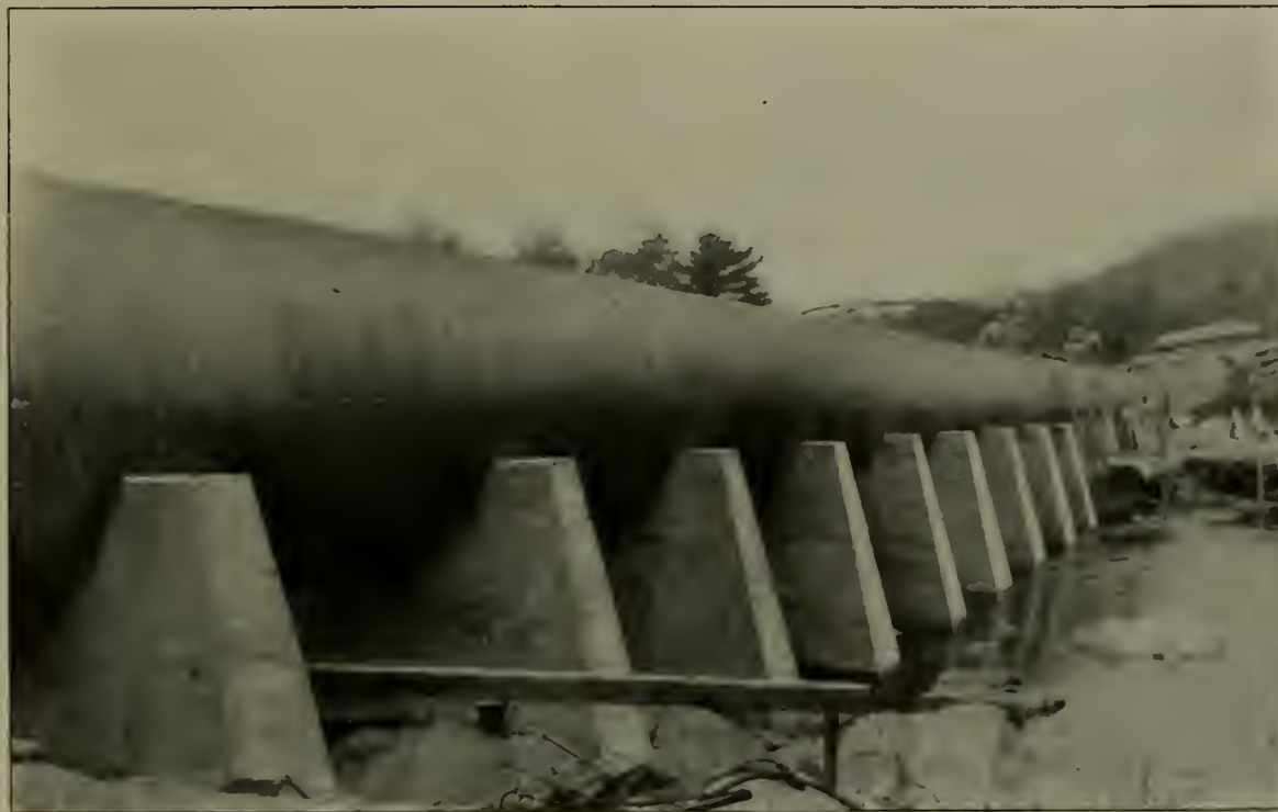
THE WATER RUNS TO THE POWER HOUSE OF THE WORONOCO PAPER COMPANY THROUGH A STEEL PENSTOCK 550 FEET LONG, BUILT IN SECTIONS AND SUPPORTED ON REINFORCED CONCRETE PIERS
