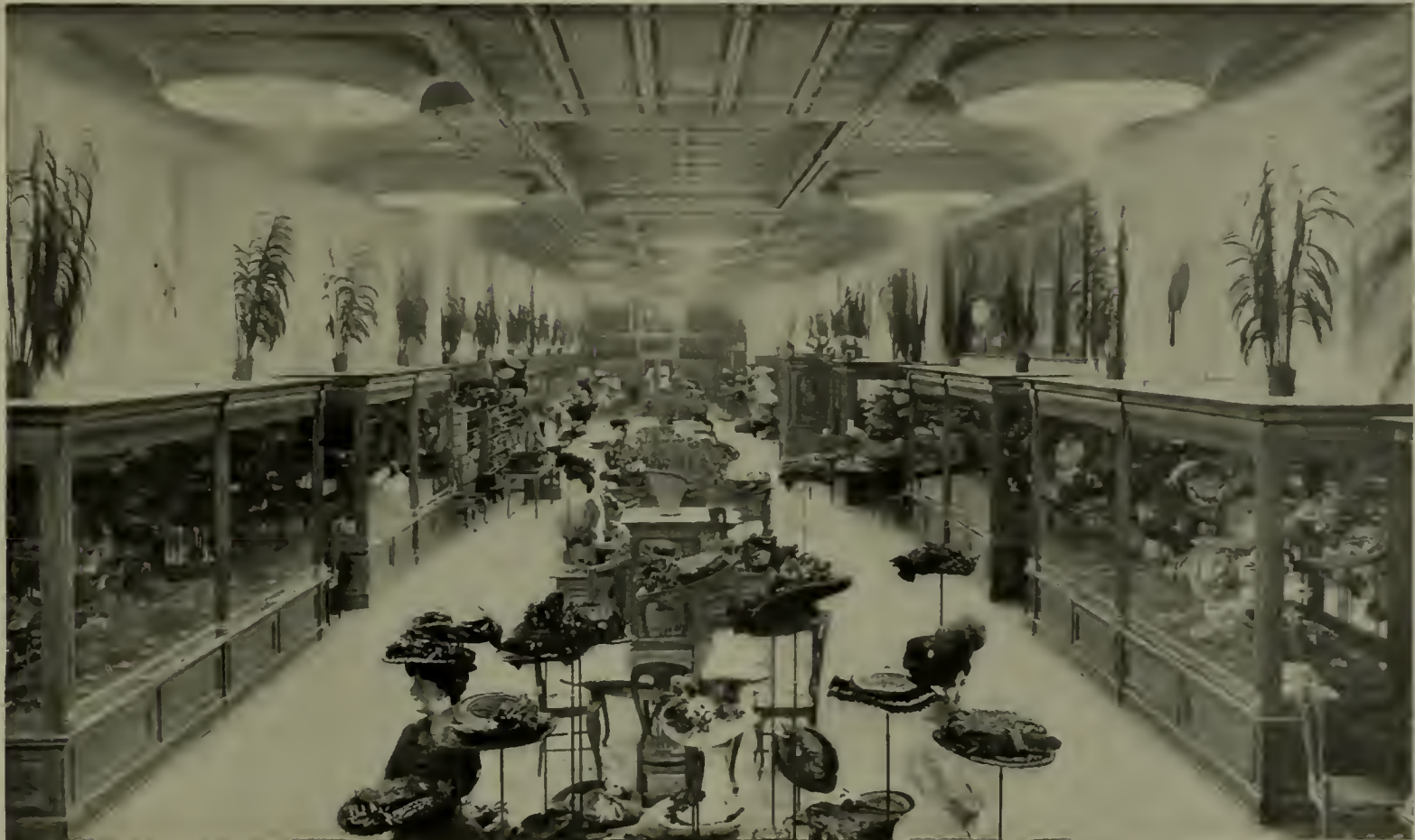
FIG. 9.—A NIGHT VIEW OF A MILLINERY STORE LIGHTED BY GENERAL ELECTRIC LIGHT-BALANCING, SELECTIVE-DIFFUSER CEILINGS
