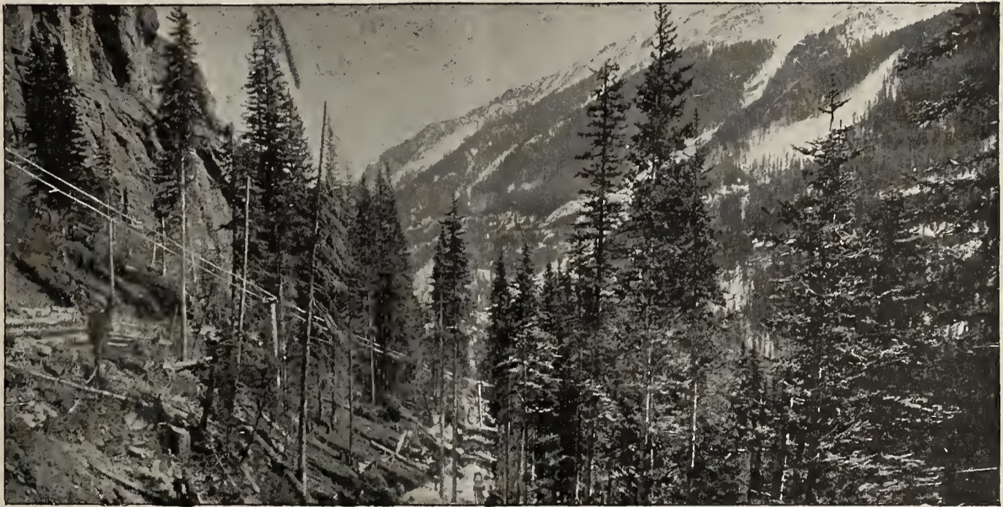
EDISON POWER PLANT IN THE MOUNTAINS.
