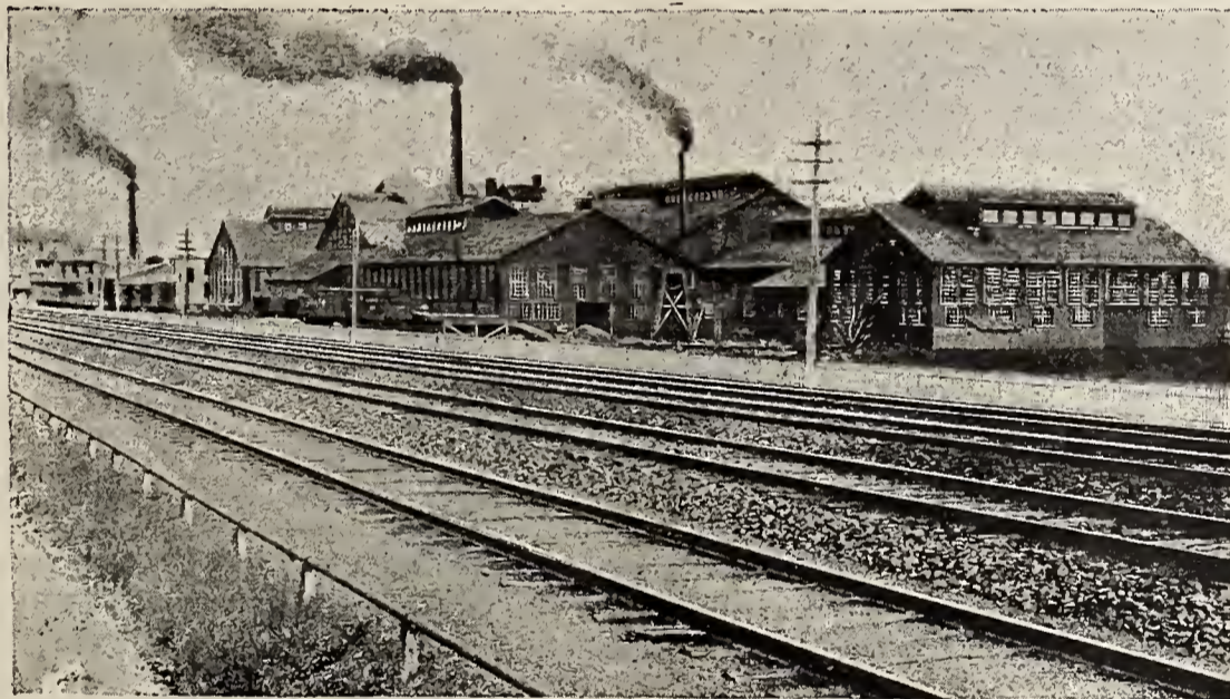
PROXIMITY TO RAILROAD.
