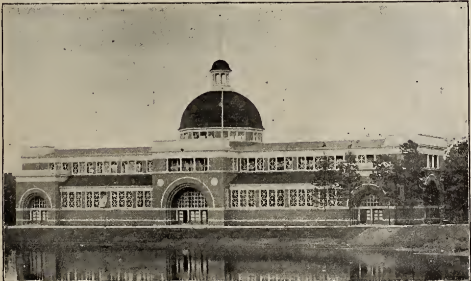
ELECTRICAL BUILDING, ATLANTA EXPOSITION, OPENED SEPT. 18, 1895.
