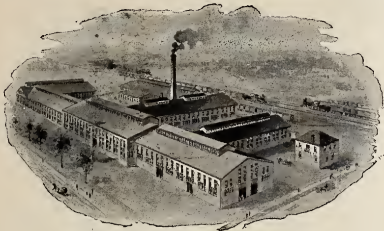
FACTORY OF C. & C. ELECTRIC CO.
