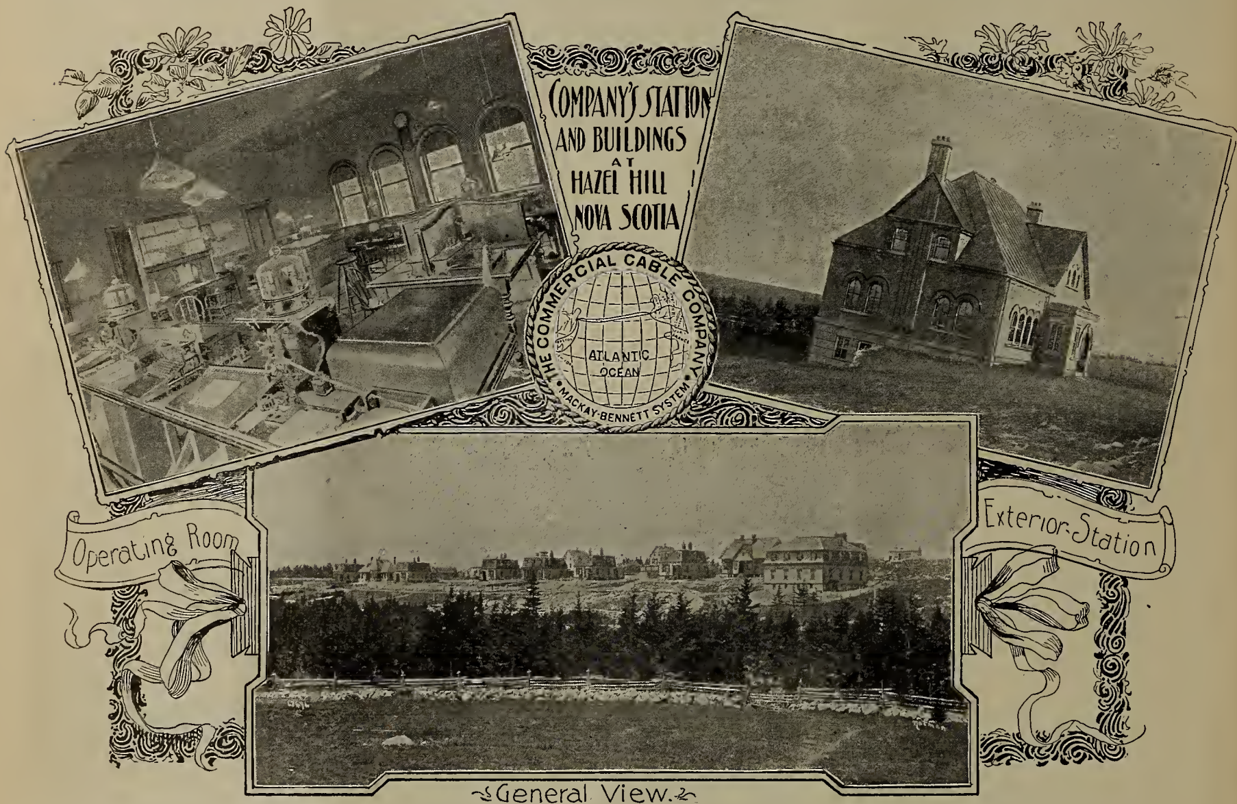
COMMERCIAL CABLE CO.'S STATION AT CANSO, NOVA SCOTIA.
