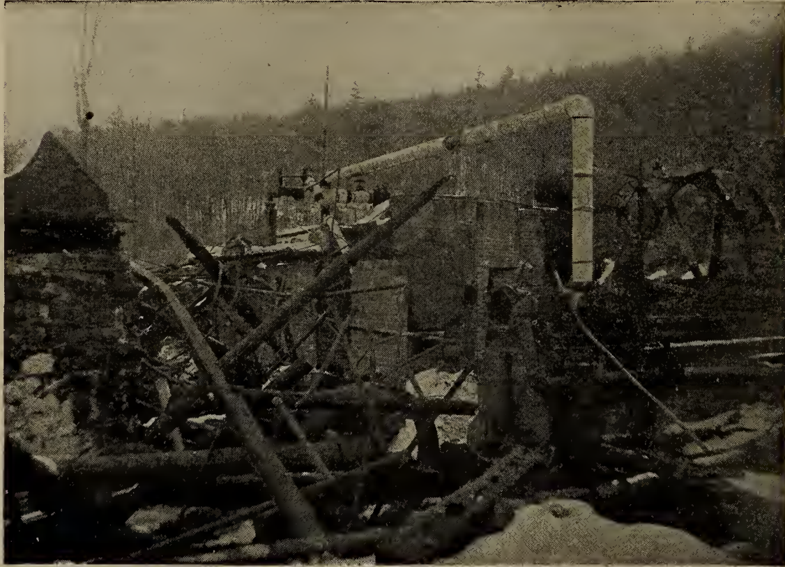
FIG. 2—MAGNESIA COVERED PIPE AFTER FIRE.
