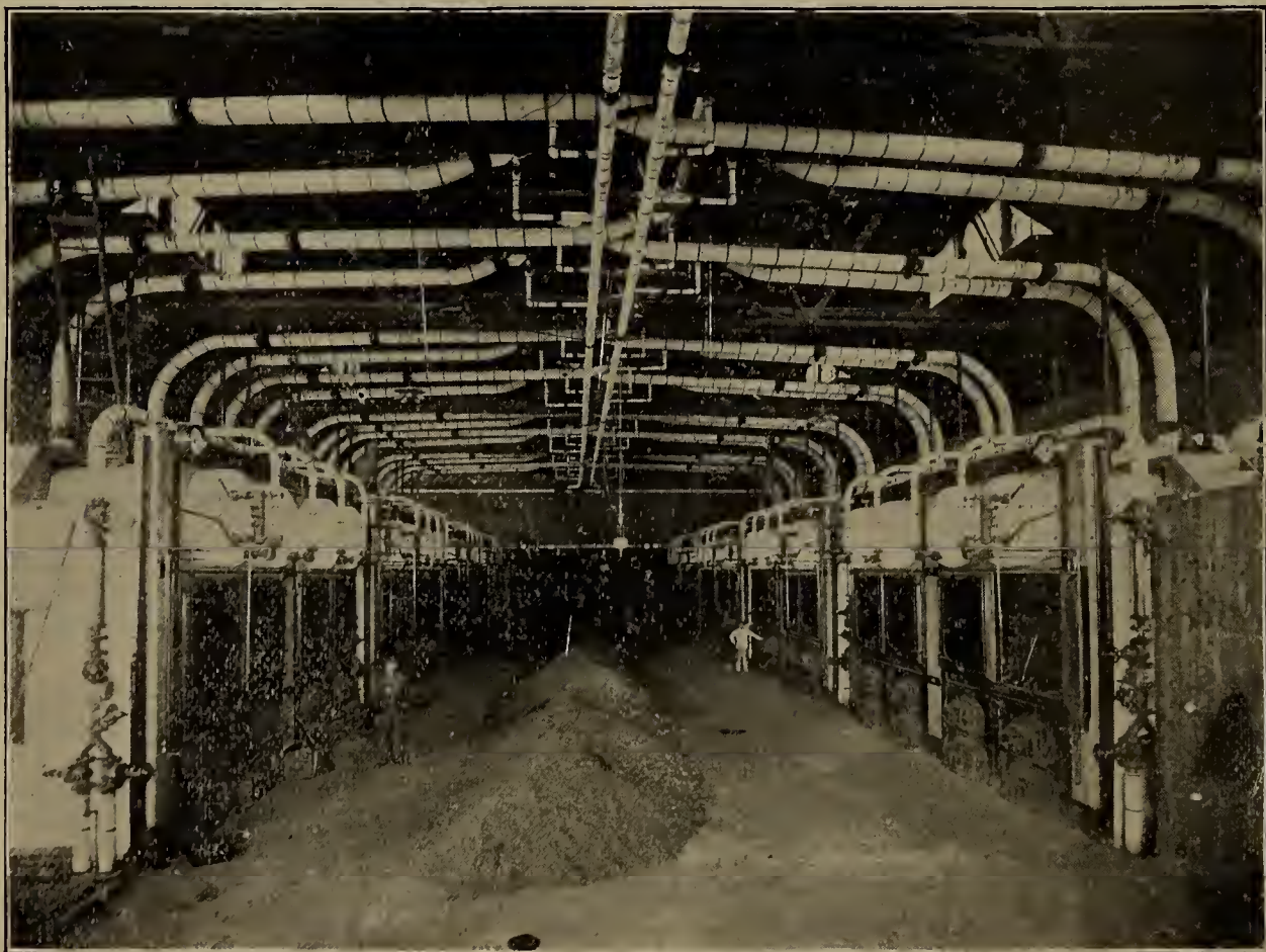
FIG. 3—MAGNESIA COVERED PIPES, BROOKLYN CITY RAILWAY PLANT.
