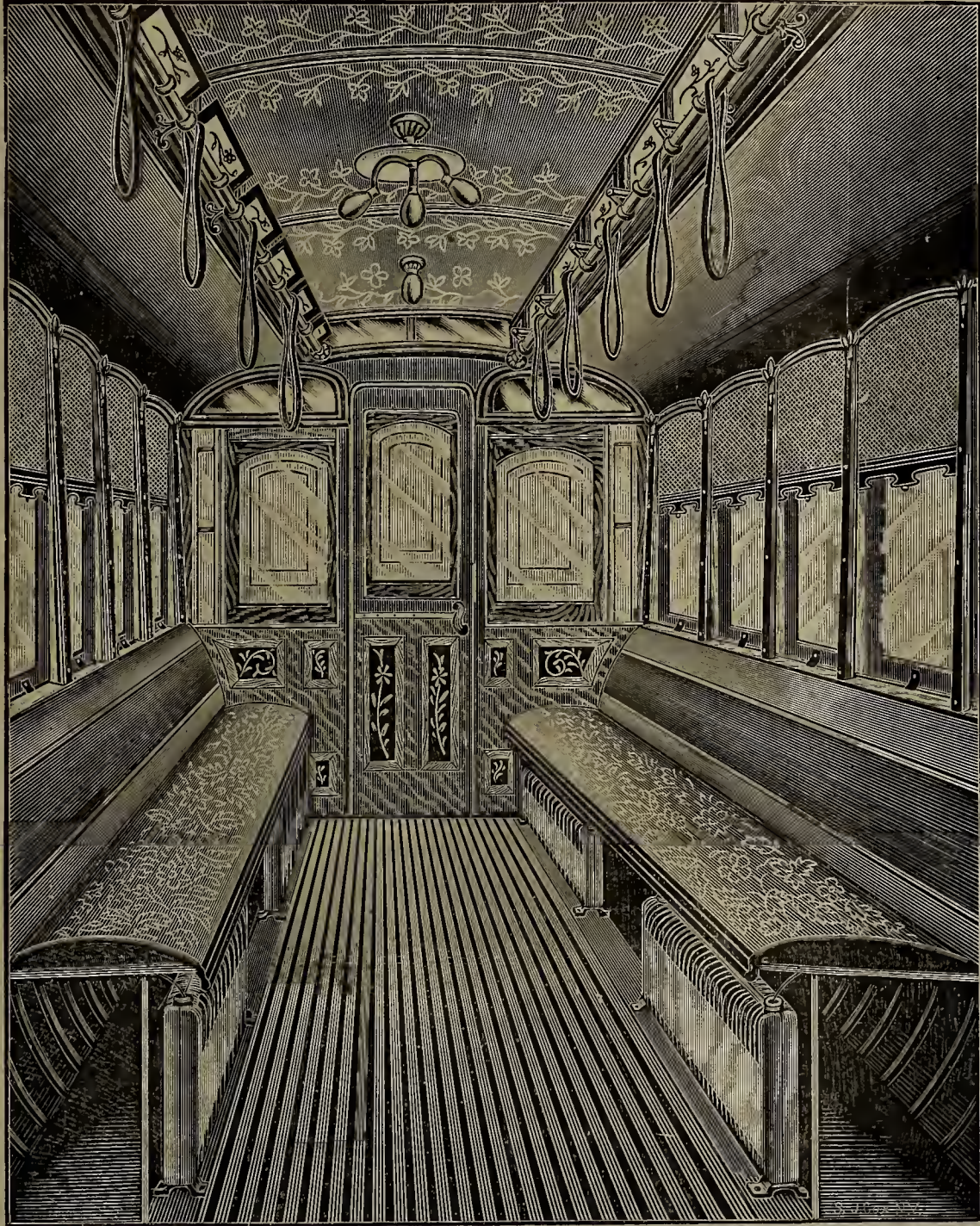
FIG. 3.—INTERIOR VIEW OF CAR EQUIPPED WITH AMERICAN ELECTRIC HEATERS.
