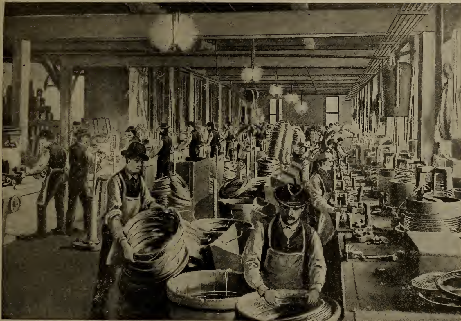
INTERIOR VIEW OF WIRE DRAWING SHOP.
