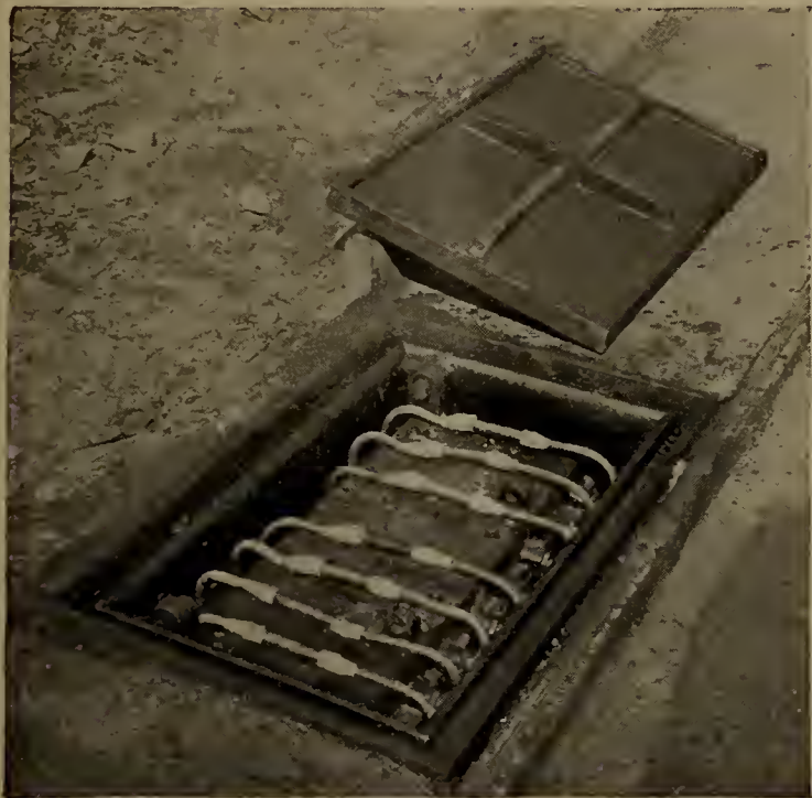
SWITCHBOX, WITH COVER REMOVED.
