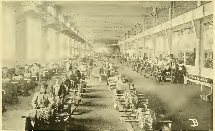
WINDING STREET RAILWAY ARMATURES.
