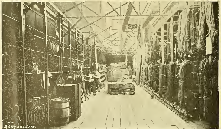
FIG. 11.—STOREROOM—BERLIN IRON BRIDGE WORKS.
