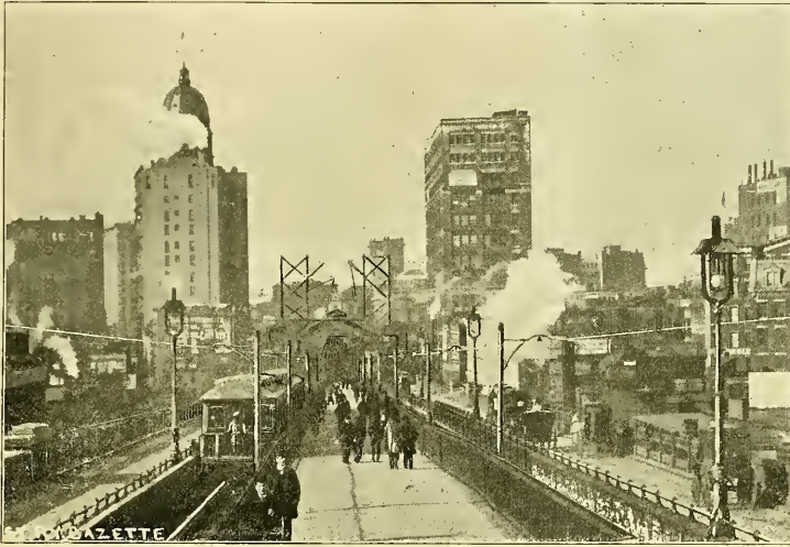
FIG. 1.—NEW YORK AND BROOKLYN BRIDGE—APPROACH ON THE NEW YORK SIDE, SHOWING POLES FOR NEW CAR LIGHTING SYSTEM.
