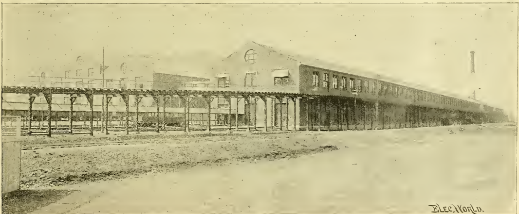
WESTINGHOUSE FACTORIES—VIEW FROM THE NORTHWEST.
