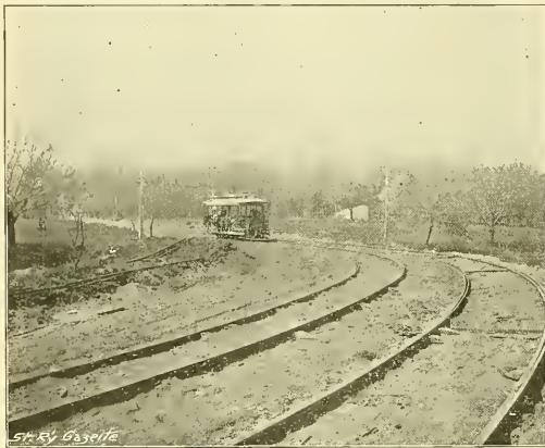
FIG. 5.—FIFTY-FOOT RADIUS CURVE SHOWING GUARD RAILS.
