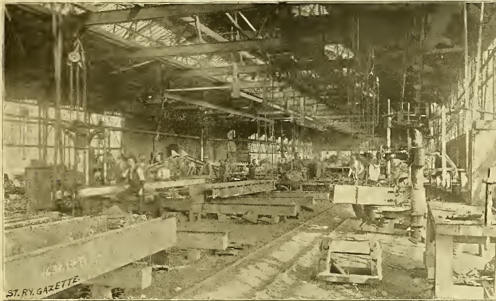
FIG. 6.—INTERIOR OF TRUSS SHOP,—BERLIN IRON BRIDGE WORKS.
