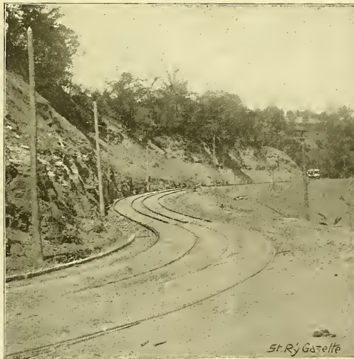
FIG. 1.—REVERSE CURVE ON BRIDGE APPROACH.
