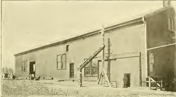
FIG. 4.—PRESENT POWER HOUSE OF THE LENOX AVENUE CONDUIT RAILWAY.
