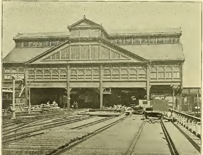
FIG. 4.—SOUTH FACE OF TERMINAL BUILDING.
