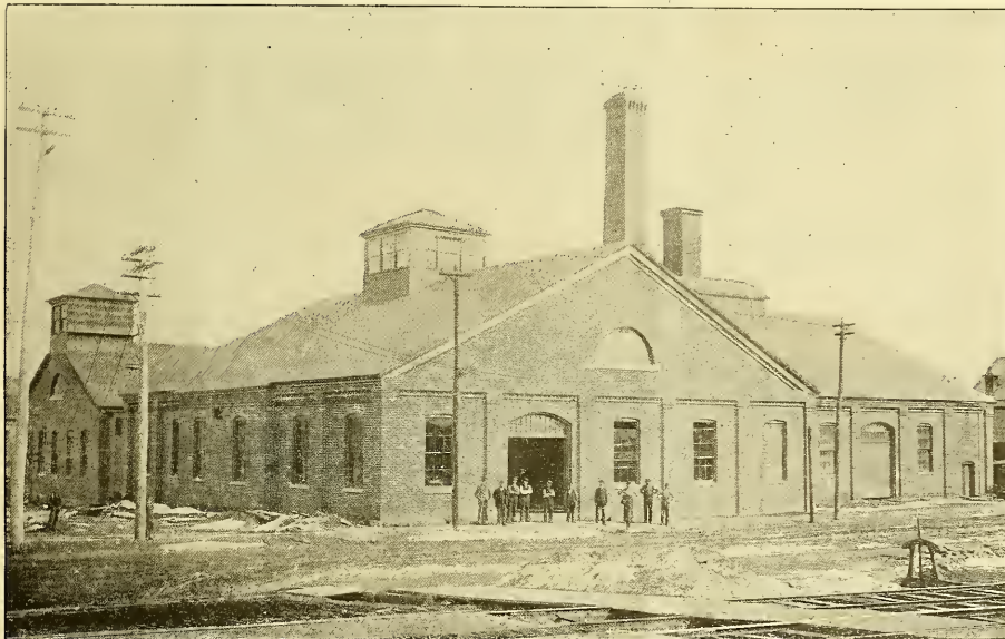
ELECTRIC RAILWAY POWER STATION IN ALLENTOWN, PA.
