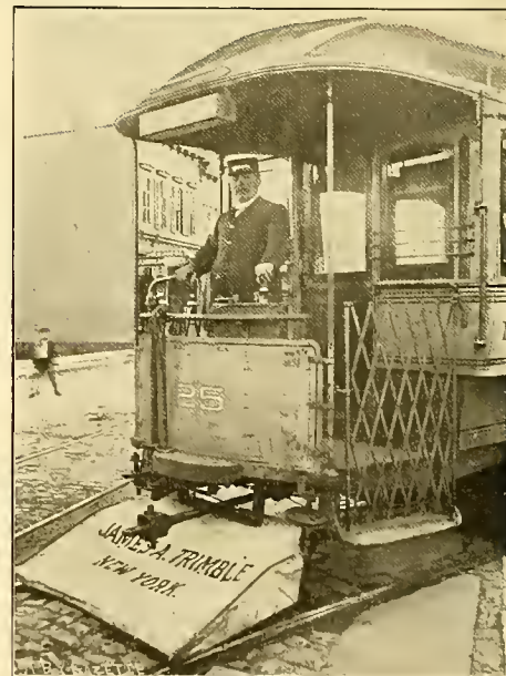
Fender in Position.
