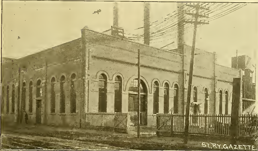
FIG. 1. RIDGEWOOD POWER STATION.
