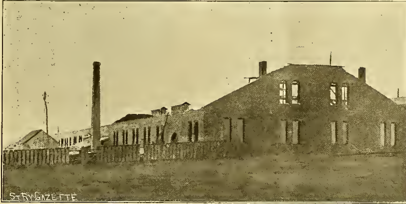
DAMAGED CAR HOUSE IN TRENTON.
