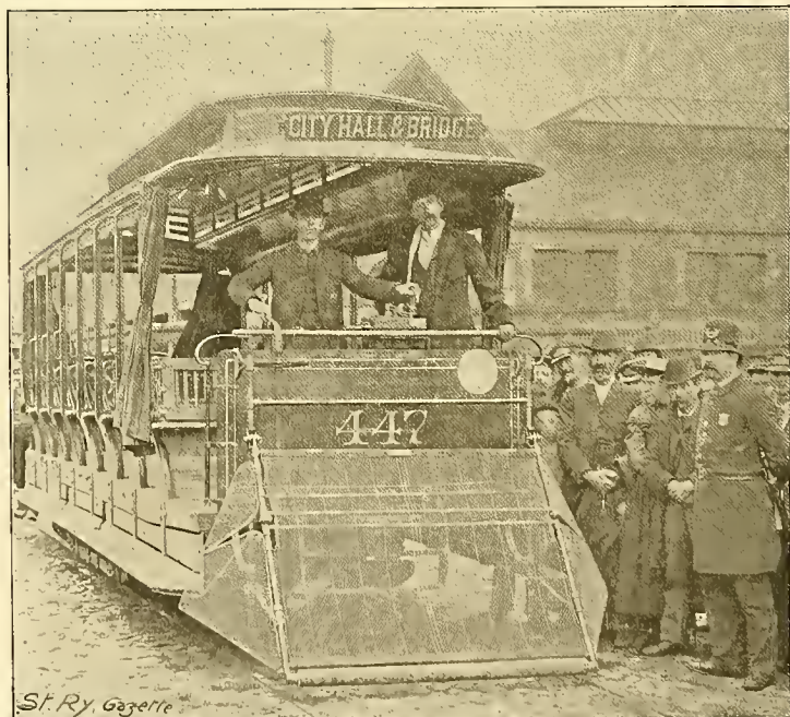
FIG. 1.—THE FENDER IN POSITION READY FOR USE.
