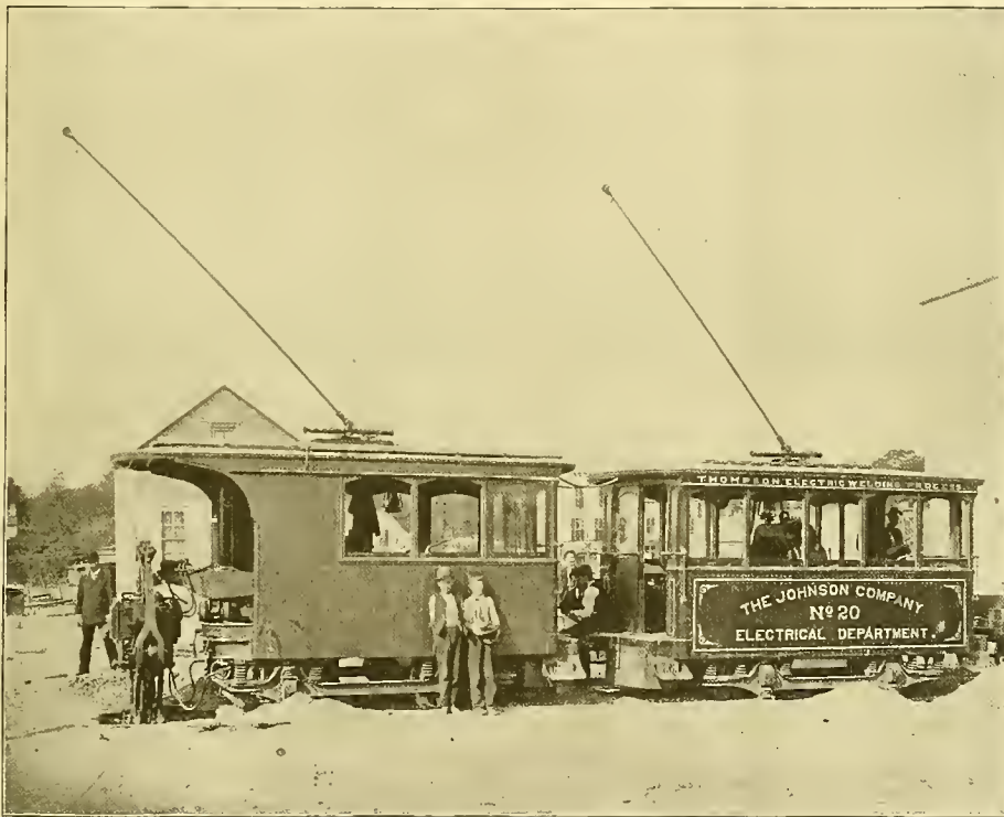
WELDING TRAIN IN SOUTH BROOKLYN.
