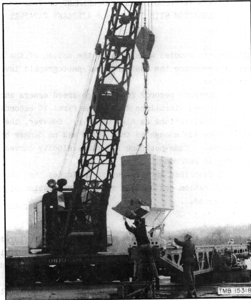
Figure 1 - Deadweight Load Being Lowered into Launching Position on the Catapult
