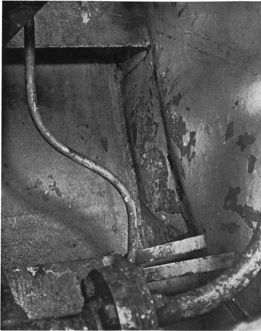
Fig. 18 Bulkhead buckling due to inboard deflection of longitudinals
