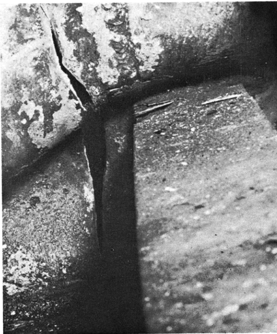
Fig. 23 Bulkhead buckling and rupture resulting from inboard motion of bottom longitudinal
