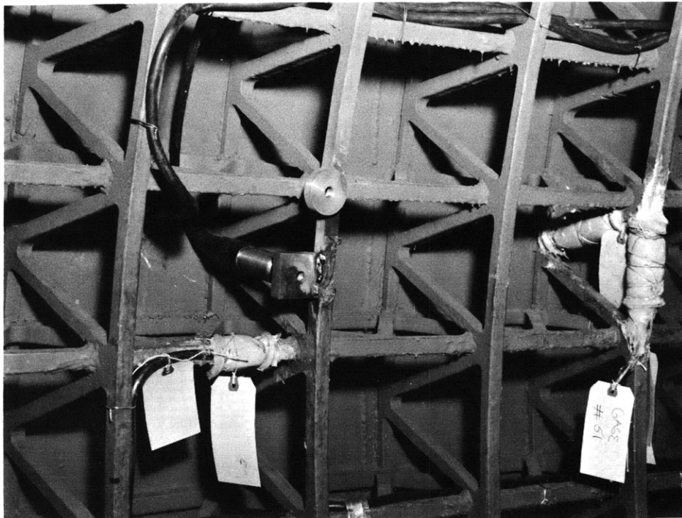
Figure 3 – Closeup of Trusswork in Dome
