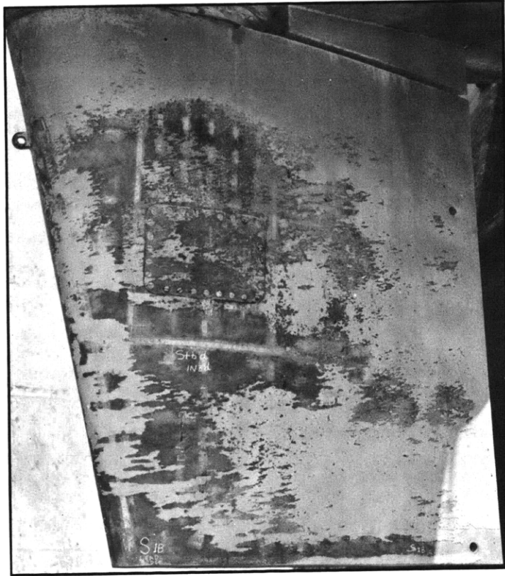
Figure 18 – Inboard Side of Starboard Rudder
