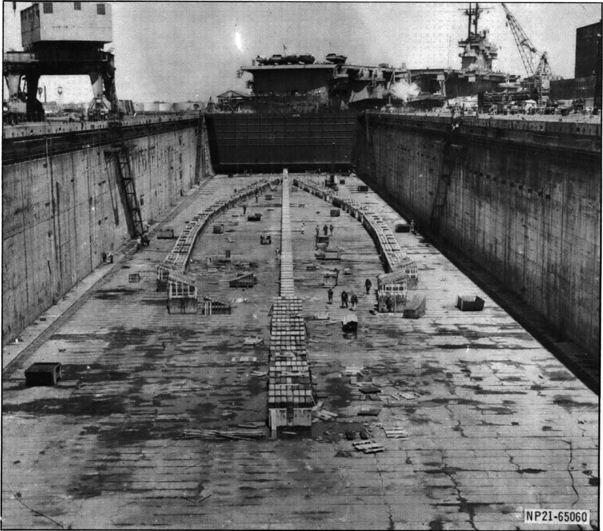
Figure 3 - Drydock Setup Prior to Docking USS FORRESTAL (CVA 59)
