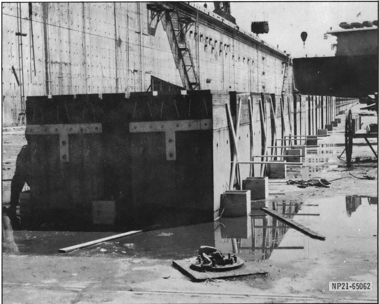
Figure 5 - View of Stern Blocks Used under USS FORRESTAL (CVA 59)
