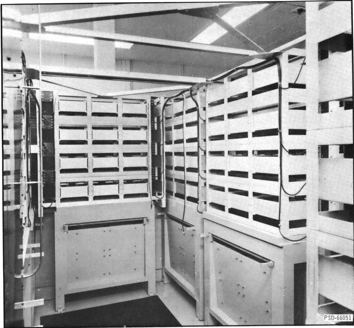
Figure 6 – Interior of Network Analyzer
