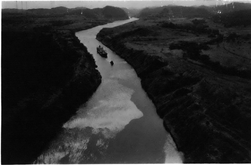
Figure 12 – Another View of Gaillard Cut Showing a Tugboat on a Hawser Ahead of a Ship
