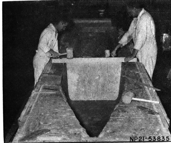
Figure 5 - Molding Clay Bin in Preparation for Casting 20-Foot Wax Models
