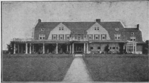
Residence of Ralph Peters, Esq., President L. I. R. R. Shingles stained with Cabot's Shingle Stains; Stucco with Cabot's Waterproof Cement Stains. Lined with Cabot's Quilt for warmth. Aymar Embury, II, Architect, New York.
