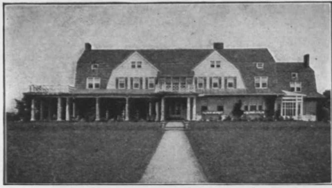
Residence of Ralph Peters, Esq., President L. I. R. R. Shingles stained with Cabot's Shingle Stains; Stucco with Cabot's Waterproof Cement Stains. Lined with Cabot's Quilt for warmth. Aymar Embury II, Architect, New York.
