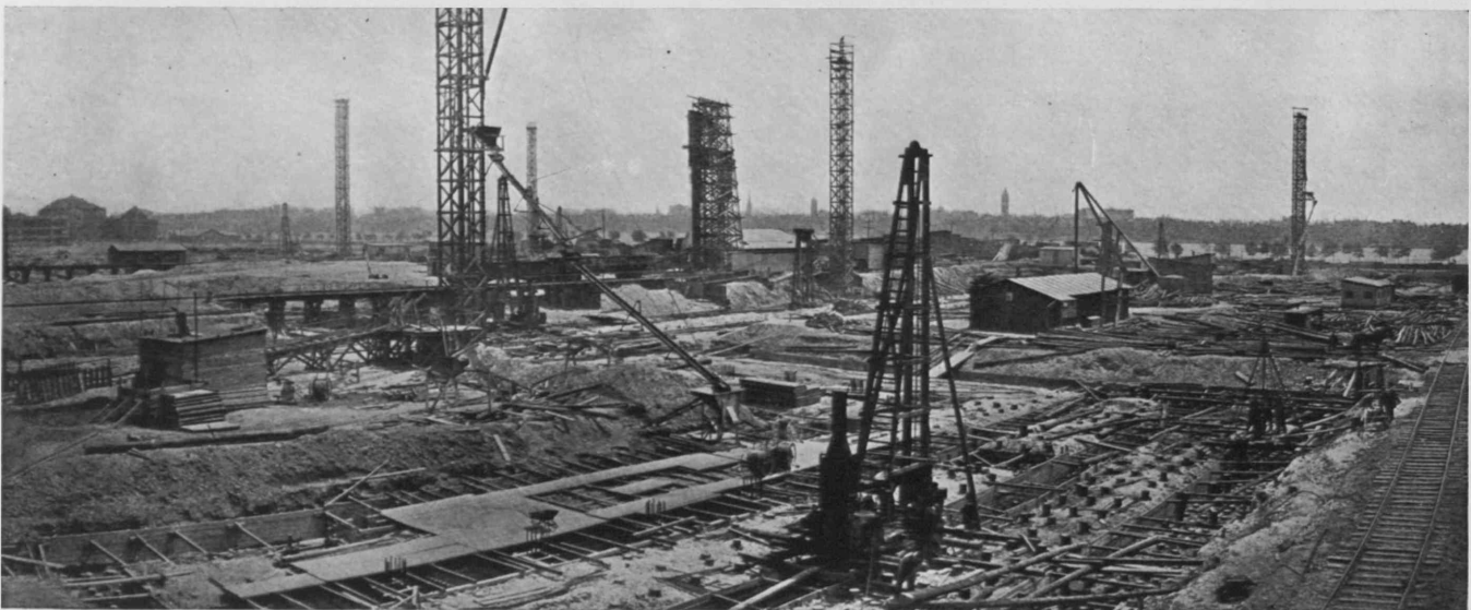
Concreting Foundations for New M. I. T. Buildings
