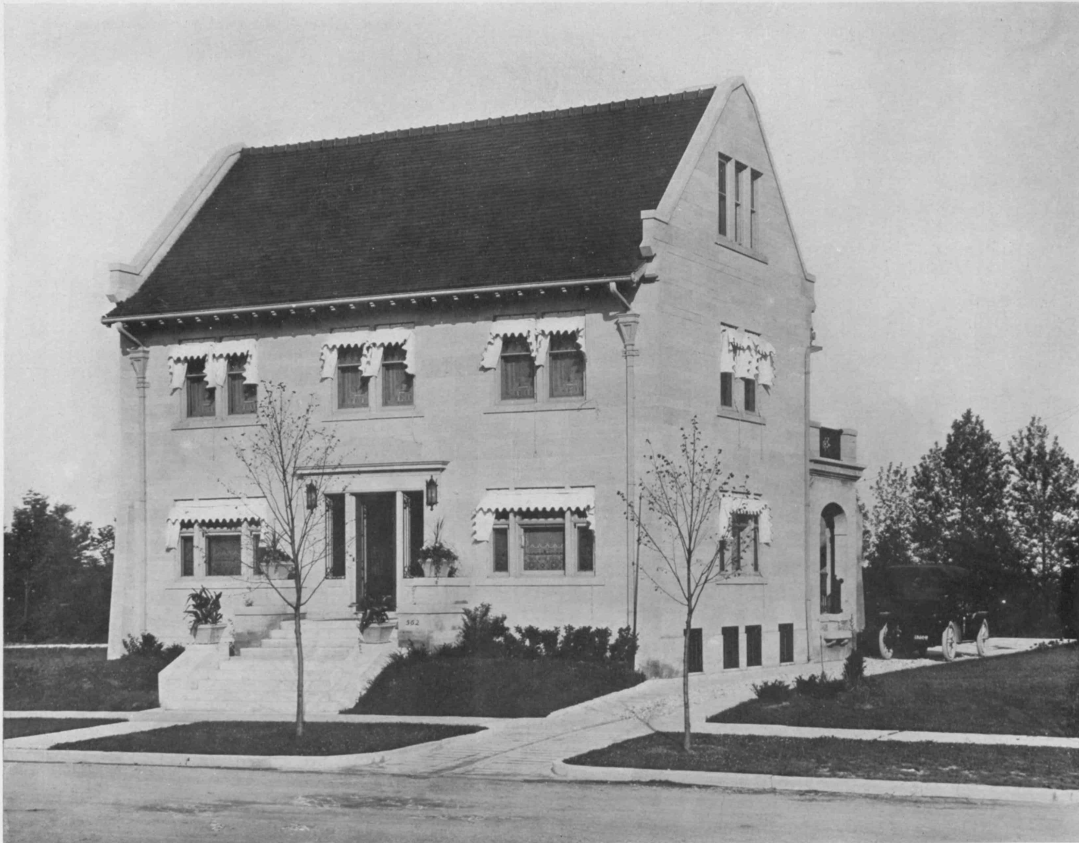
HOUSE, MILWAUKEE, WIS.
