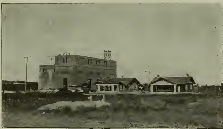
Sub-Station, Electrification Scheme.
