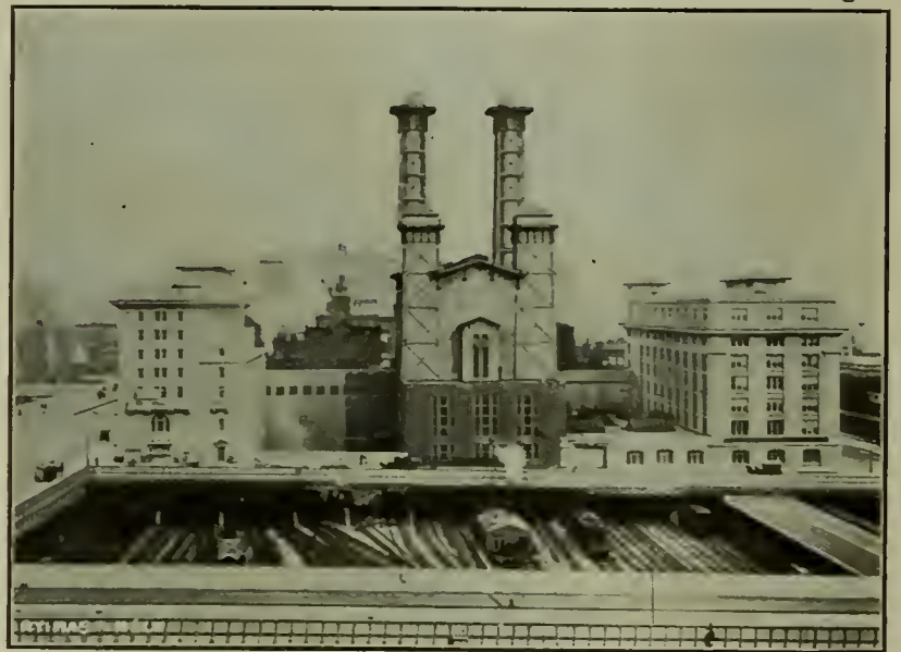
A Station Where the "Silent Power" is Born.
