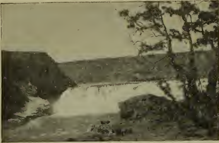
Great Falls, Mont., on the Missouri River. Site of a 60,000 K. W. Hydro-Electric Plant.
