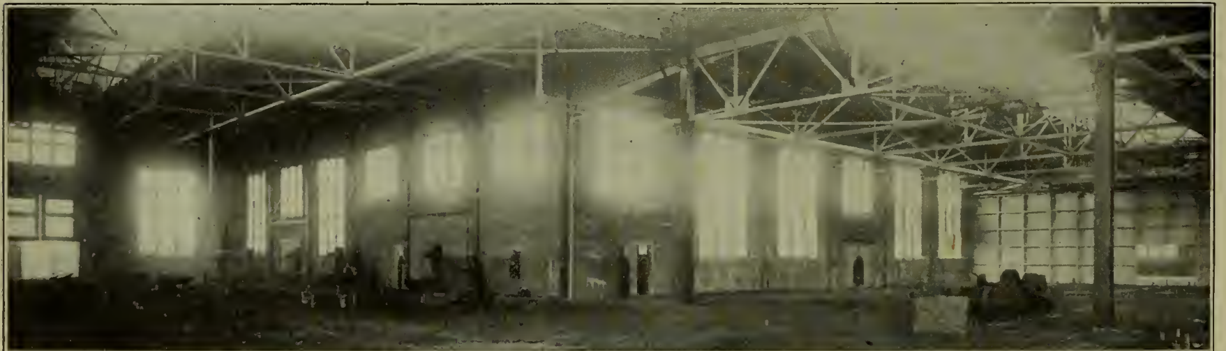
Interior of Blacksmith Shop.
