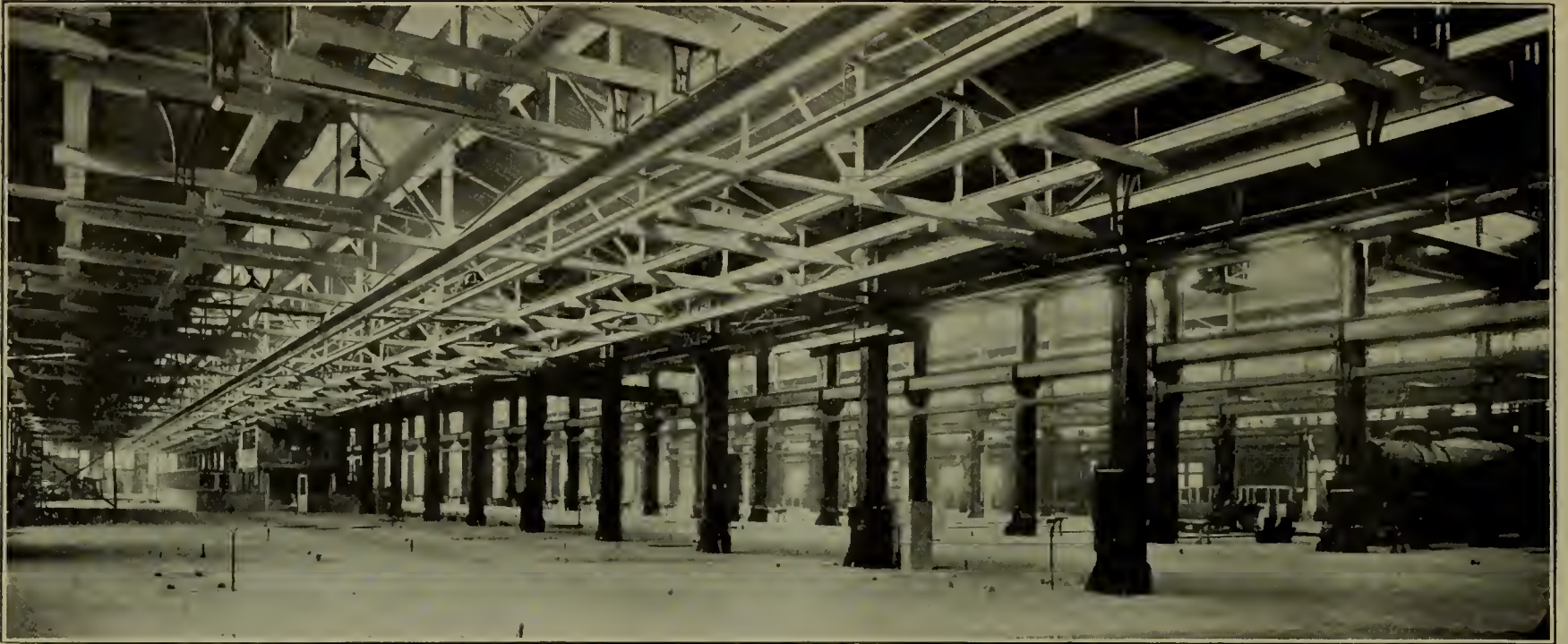
Interior of Machine and Erecting Shop.
