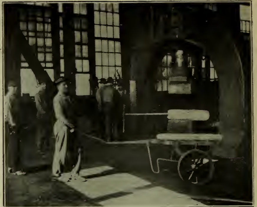
Slabs Made from Scrap Iron.
