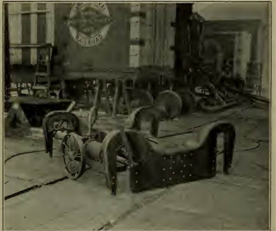
Reinforcing Fox Trucks.
