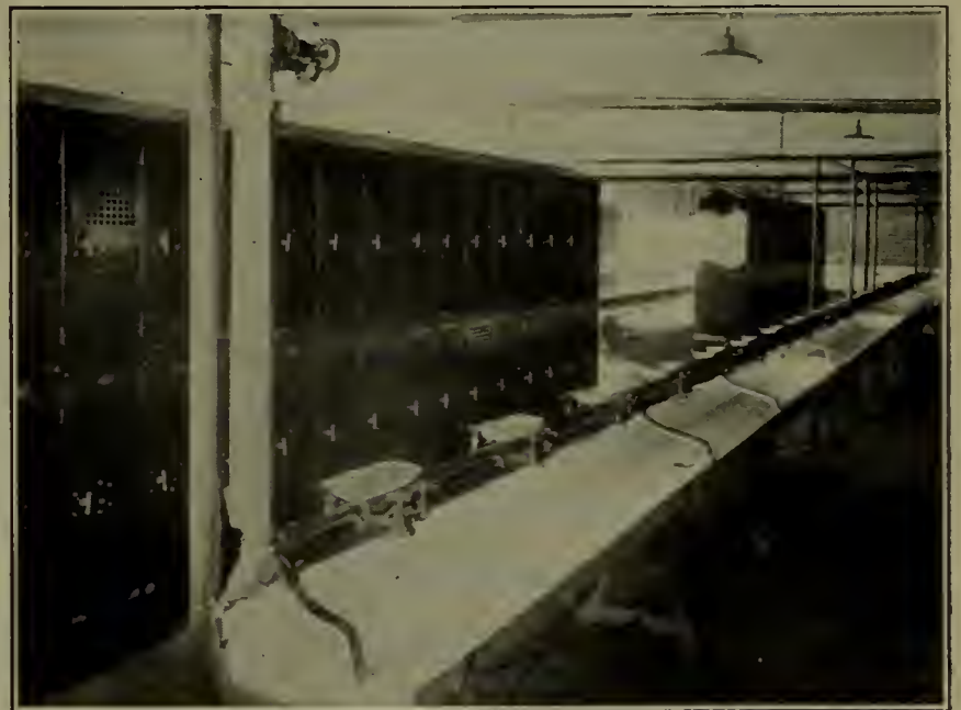
Corner of Wash Room, Locomotive Repair Shops.
