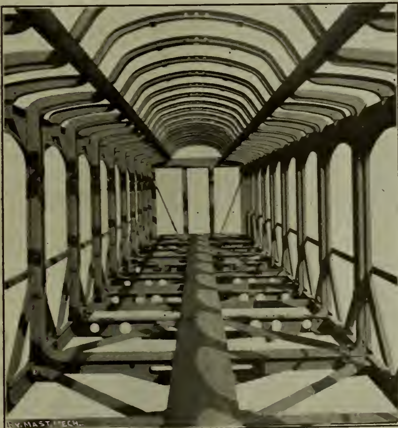
Interior frame Erie car, showing strong roof construction.
