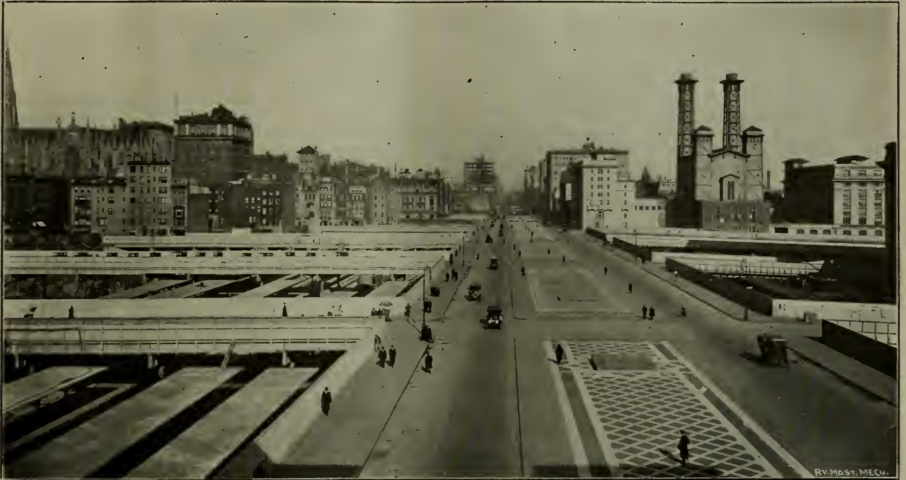
Looking north on Park Avenue from Our New Offices in the Vanderbilt Concourse Building, showing the area under which the inbound and outbound tracks are laid.
