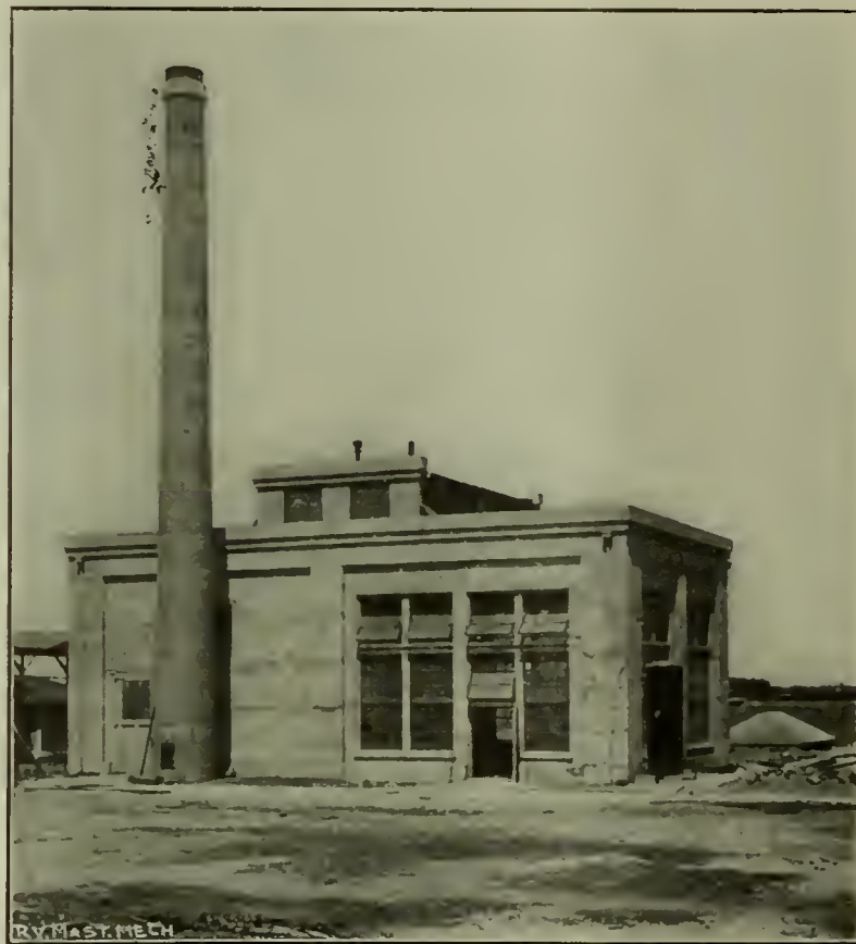
Power House with Underground Wires.
