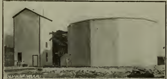
G. T. P. Oil Storage Tank.
