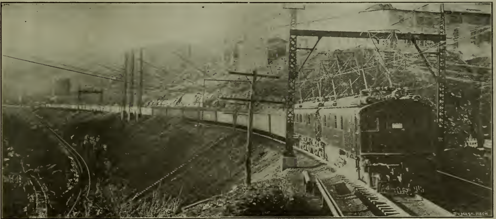
Heavy electrically driven train on the Norfolk & Western hauled by two units as one.
