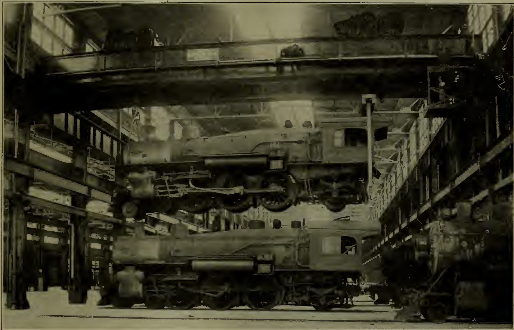
Erecting Bay, Locomotive Repair Shops of the Chicago & Alton R. R.
