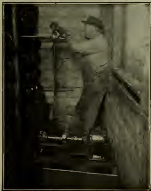
Removing Scale from Ammonia Condensing Pipes.
