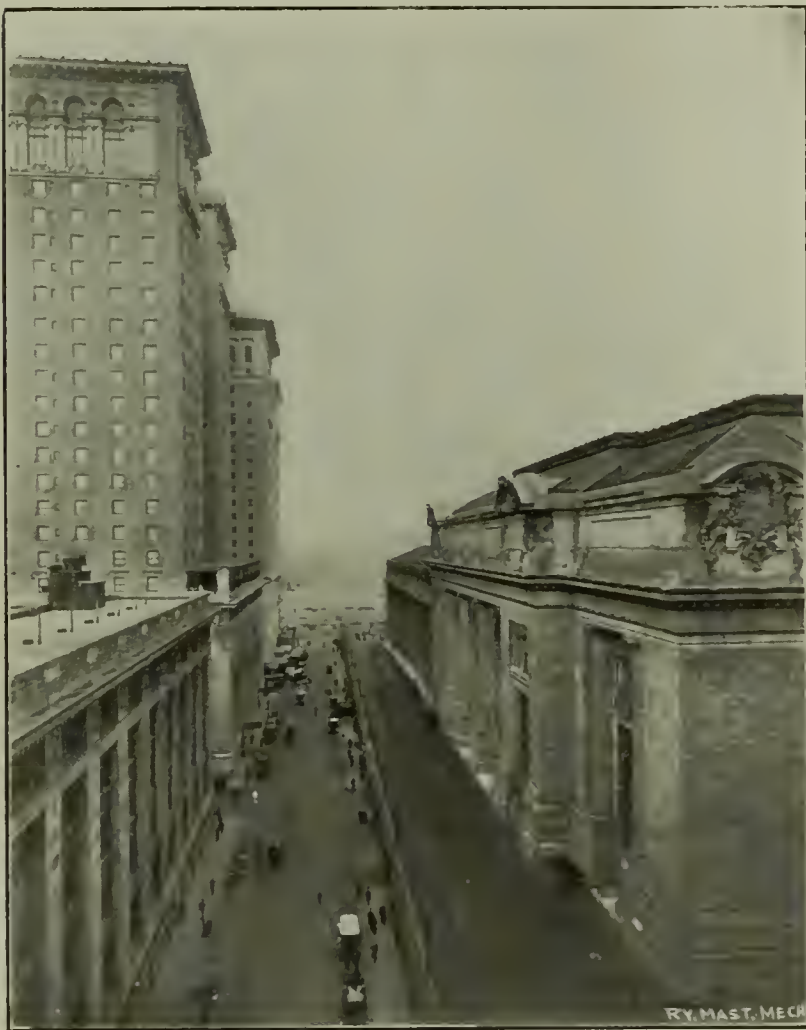
Vanderbilt Avenue north from Forty-second Street. The last tall building on the left is the Vanderbilt Concourse Building.
