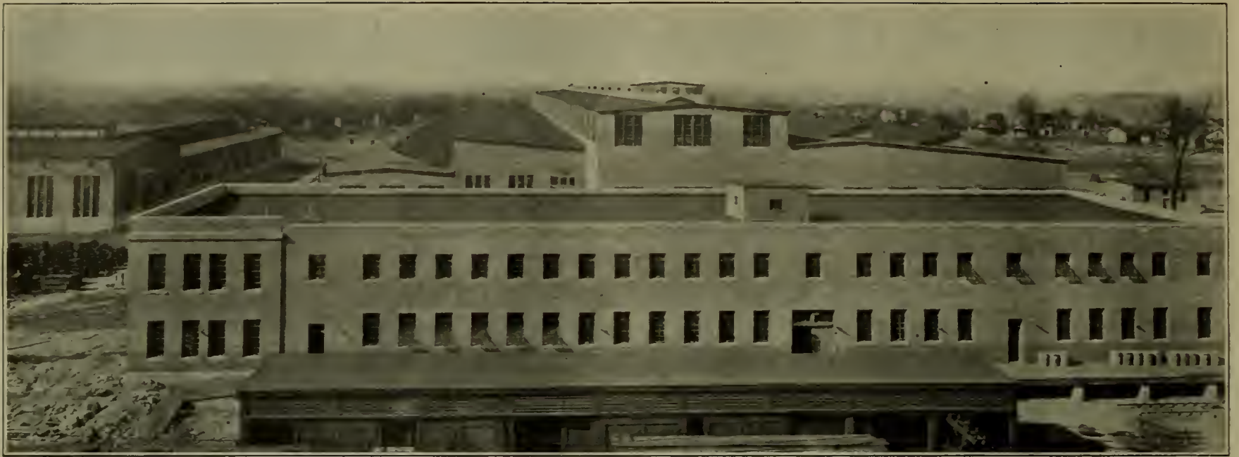
General View of New Locomotive Repair Shops of the Chicago & Alton.
