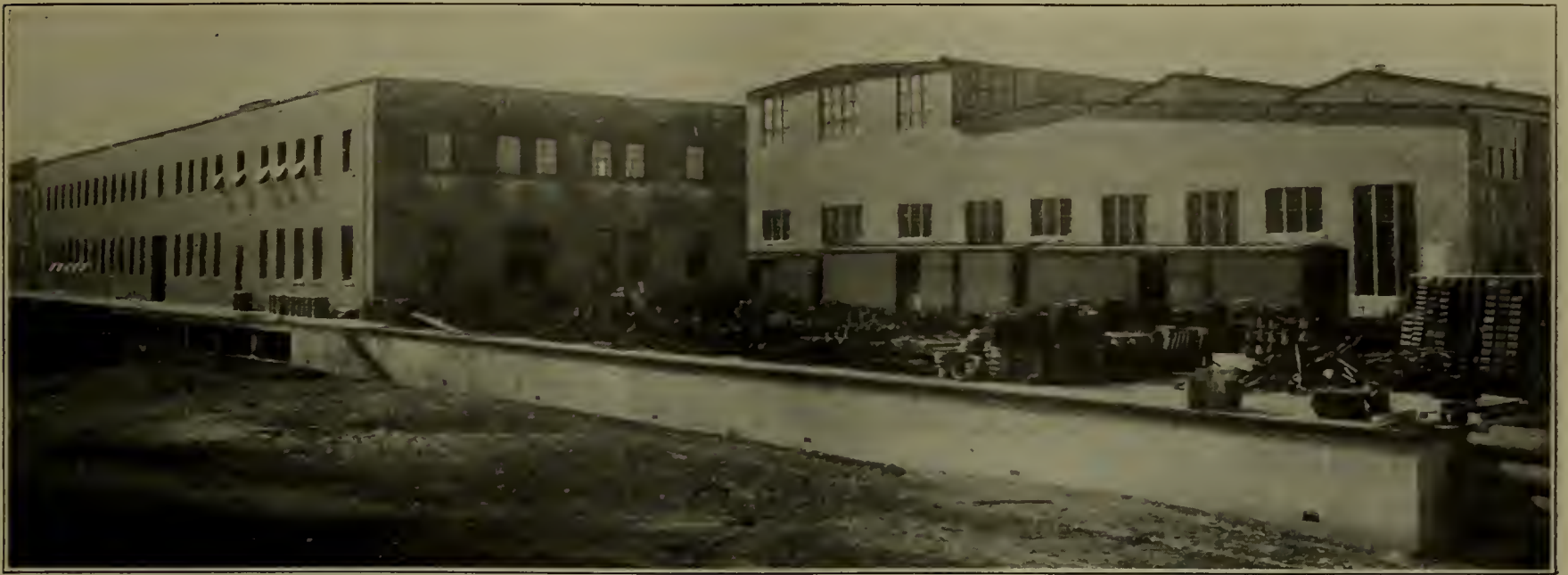
Castings Platform, Bloomington Shops.
