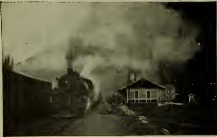
Avery, Idaho, Western Terminal of the Proposed C. M. & St. P. Electrification.
