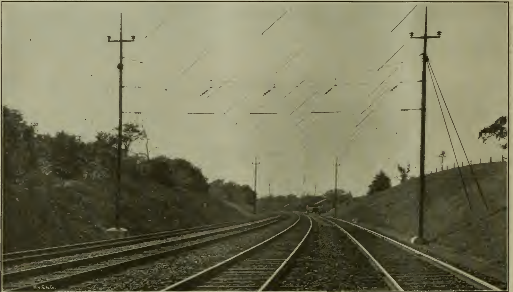
View of Pennsylvania Railroad, Showing Catenary Suspension System as Applied to Curves.
