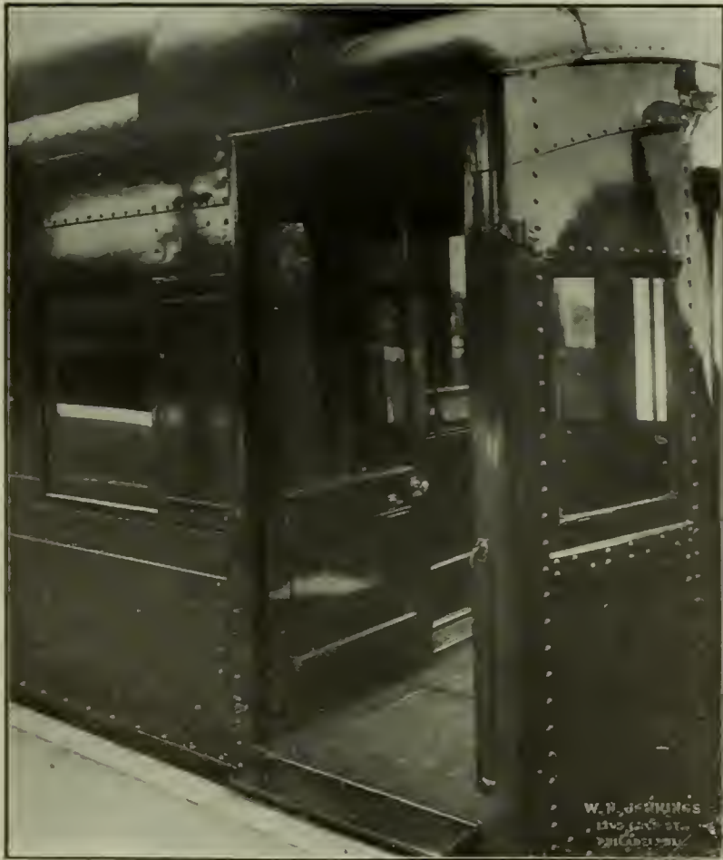
Door Open, Trap Down, Extension Out.
