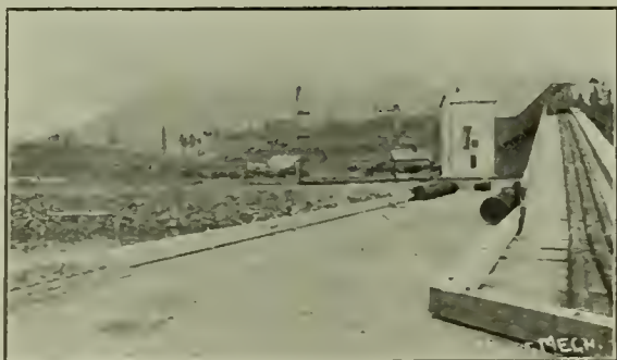
Oil Pipes on Foot Bridge, G. T. P.
