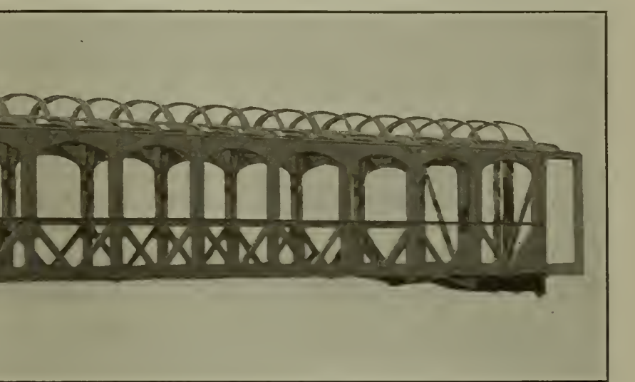
Steel framing of Erie passenger coach, showing heavy gusset plates back of door.
