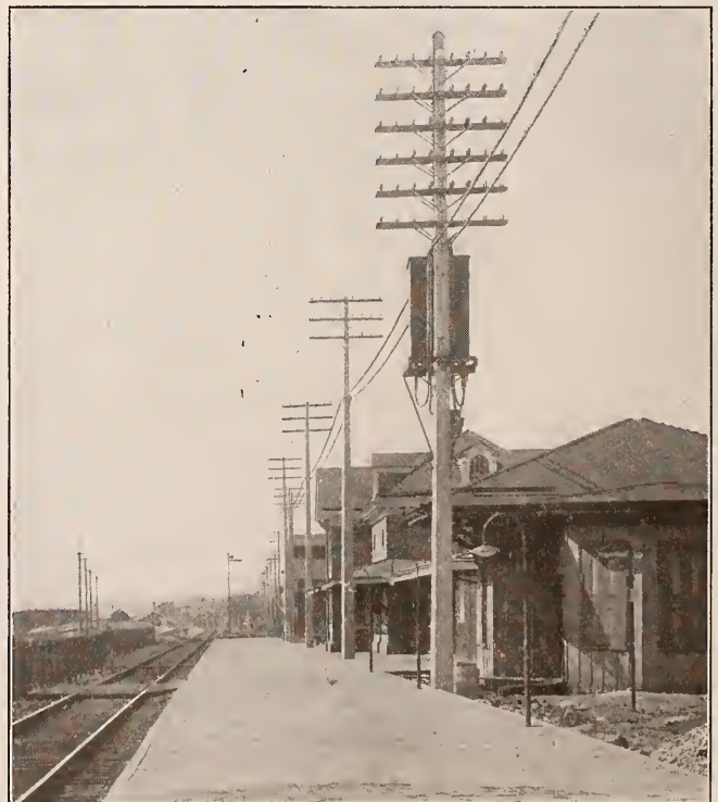
Fig. 5.—Square Heavy Concrete Pole Line
