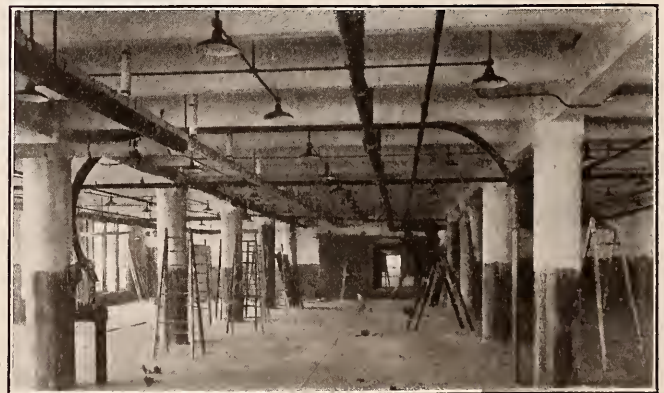
Fig. 7—Warehouse lighting installation
