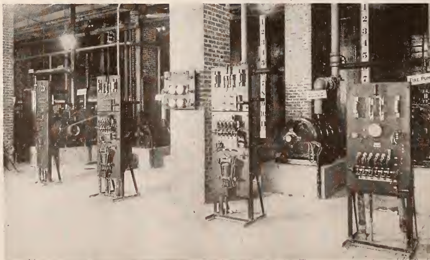
Pumps and Controllers in the Basement Machine Room
