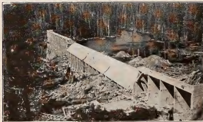
Fig. 2.—Another view of dam under construction
