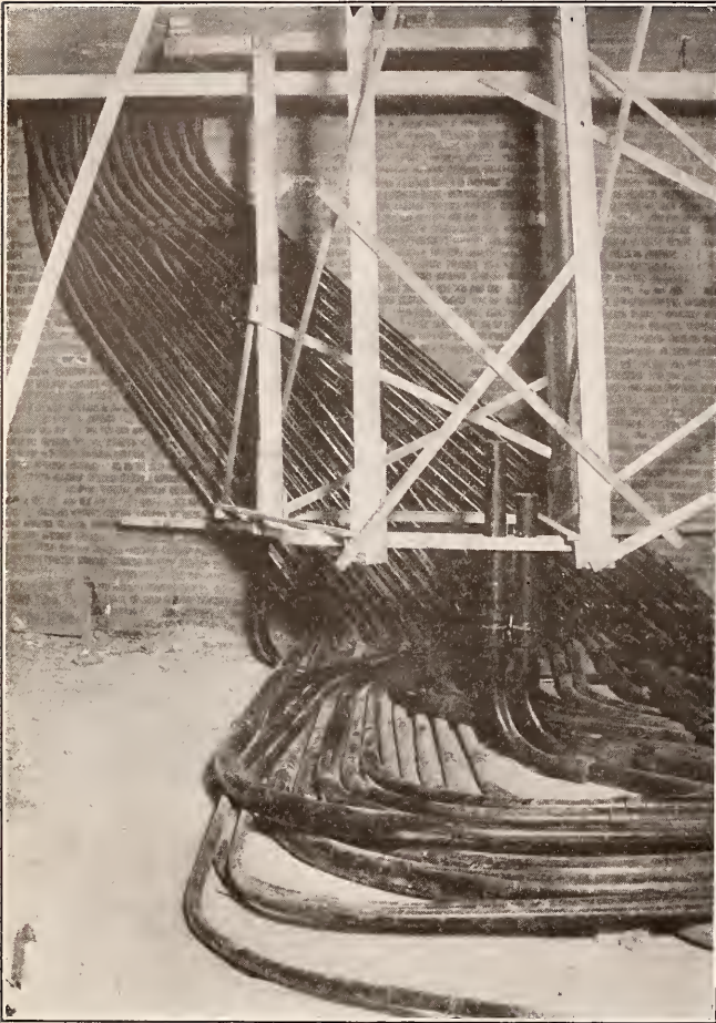
Fig. 10—Line of conduit risers in office building
