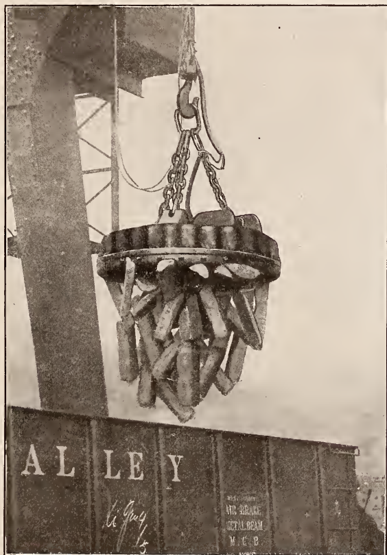
Lifting electro-magnets unloading iron
