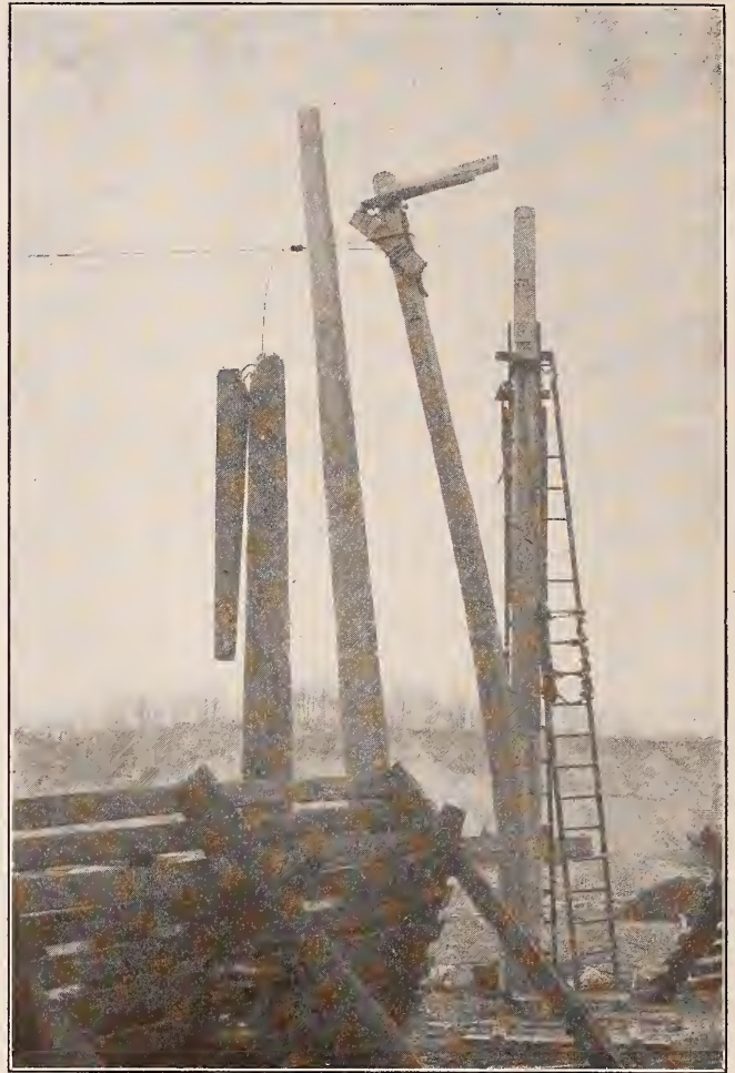
Fig. 2.—Pole No. 5 Under Test
