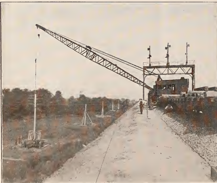
Fig. 1.—Building Hackensack Meadows Line. Poles weighing 5,000 to 6,000 lbs.
