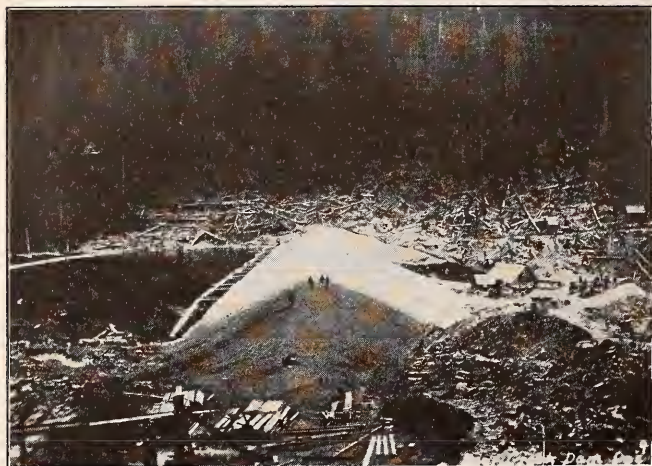
Fig. 1.—Dam under construction
