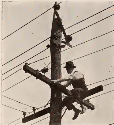
Universal Arrestor on a single phase lighting circuit.
