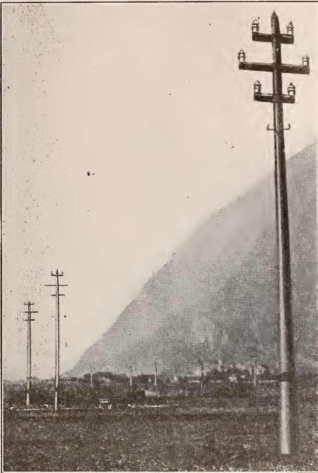
Fig. 6.—A Model European Hollow Concrete Pole Line
