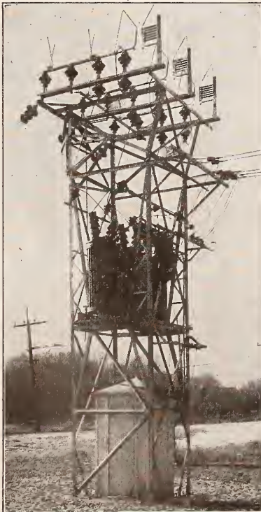
Fig. 7—Substation With Switch House
